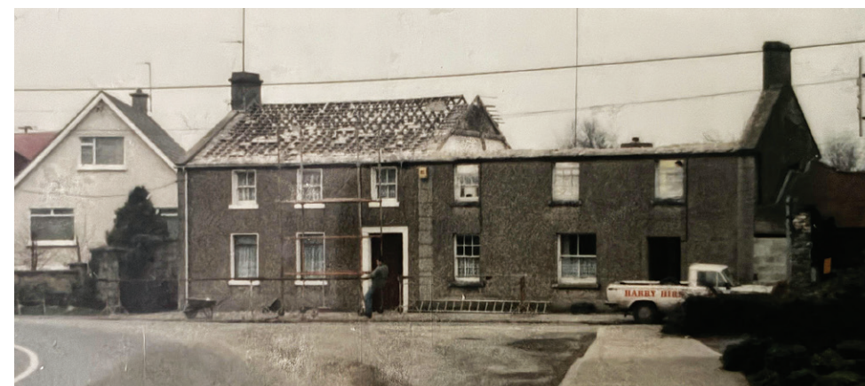
Barrack House before restoration, early 1990s. Courtesy of Pat Kelly
