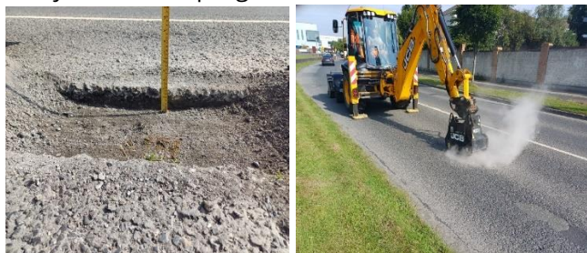
Trial hole samples taken on Barnageeragh Distributor Road to determine existing road build up prior to tendering for full resurfacing works as part of this year's roads programme.
