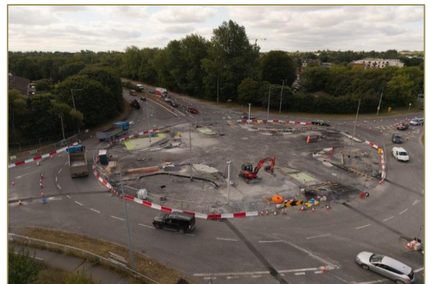
Works at Estuary Roundabout
