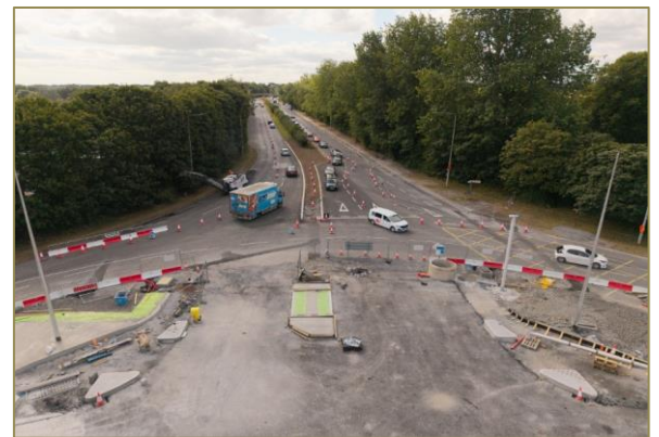
Works at Estuary Roundabout – Islands in place
