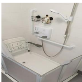
Level Access Shower recently installed
