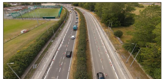
Cycle lane kerbs in place between Estuary Rd and Bostik junction
