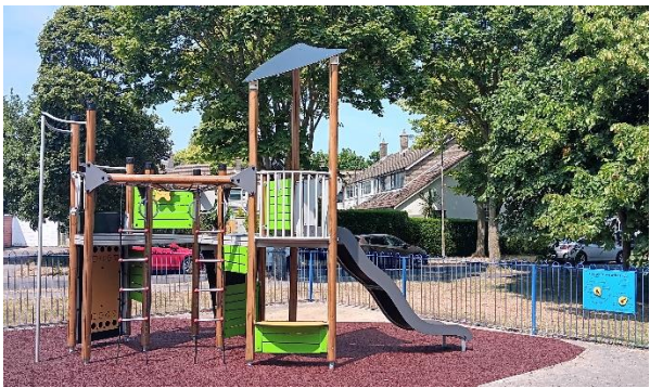
A new play unit has been installed, replacing the older unit beyond repair.
