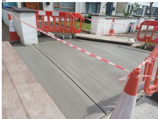
Replacement of concrete footpaths at Orlynn Park, Lusk by Balbriggan construction crew as part of roads general maintenance works.
