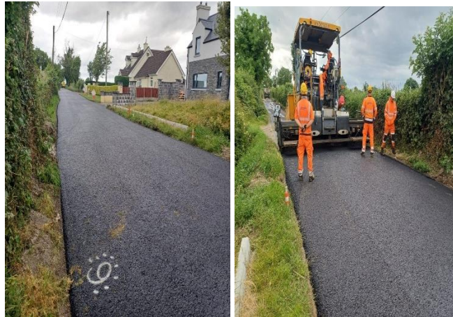
Roads programme continuing in preparation of this year's surface dressing season with the macadam overlay of Palmerstown Road, Oldtown.
