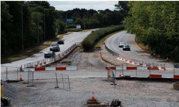
Site clearance at Malahide Rd and central medians as part of the project acceleration
