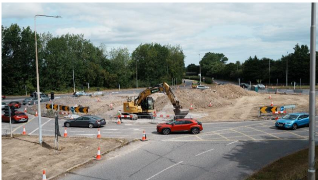
Site clearance at Malahide Rd and central medians as part of the project acceleration
