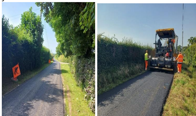
Macadam overlay on Leastown Lane as part of this year's roads programme. This road is to be surface dressed by roads outdoor staff at a later date this year.
