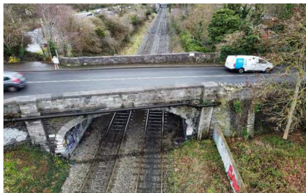
Aerial image of the existing railway bridge OBG11, looking east
