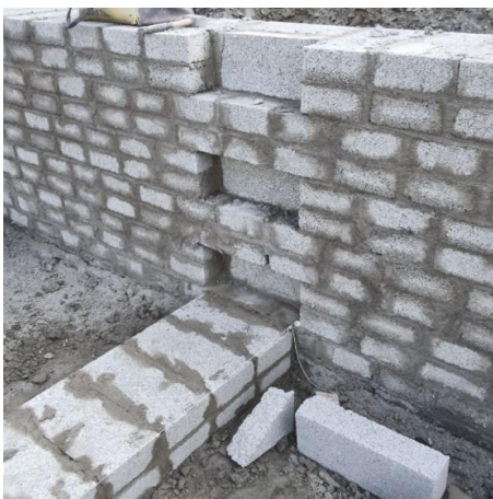
Checking blockwork on a site in Lusk
