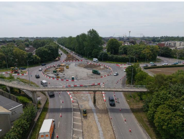
Works at Estuary Roundabout
