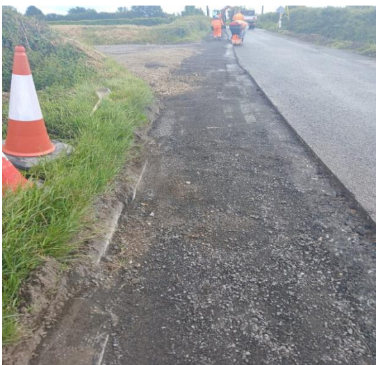
Road repairs carried out by Roads Crews at Cross of the Cage, Skerries ahead of this year's surface dressing program.
