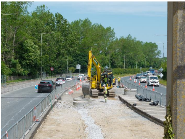
Works at Bostik for the new Bostik junction
