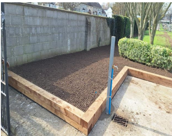
Landscaping works at Balgriffin Burial Ground
