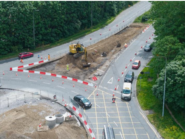
Works in the centre medium of the R132 road
