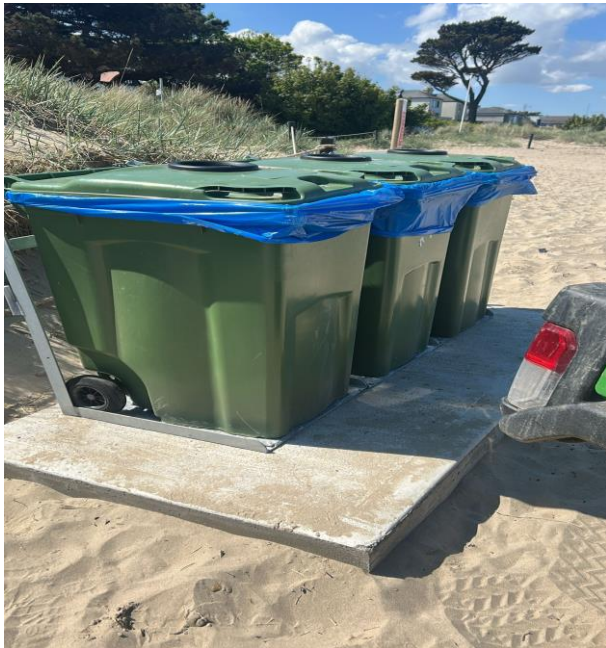
Installation of new bin bases Howth Malahide.
