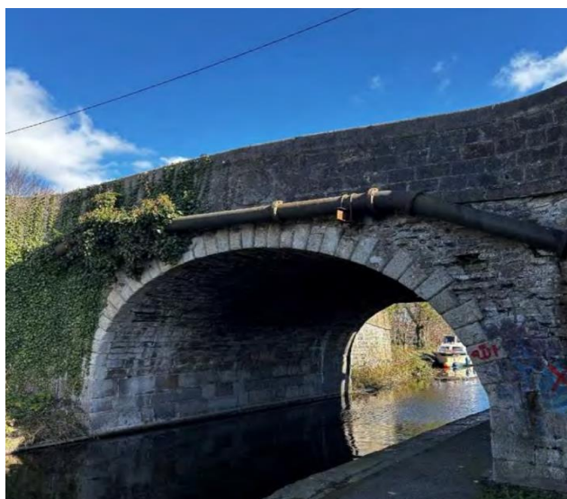
Image of the existing Granard Bridge, western elevation
