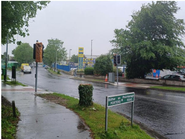
New pedestrian crossing constructed on Porters Road in Coolmine Industrial Estate, awaiting ESB connection.
