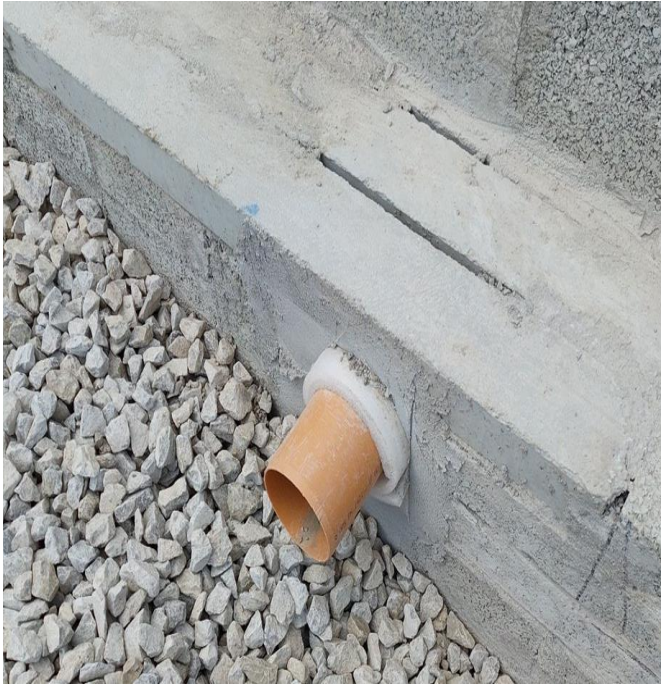
Checking Services at foundation level in apartments in Lusk.
