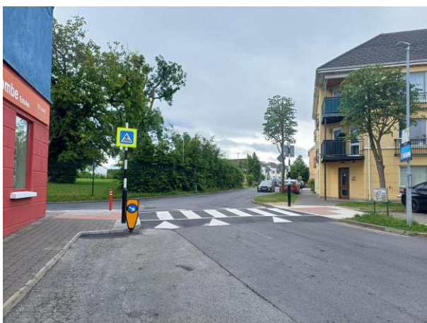
New pedestrian crossing completed on Sweeney Mews in Ongar Village.
