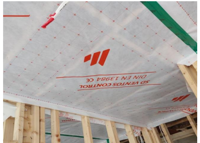
Inspecting Airtightness layer on a creche in Balbriggan
