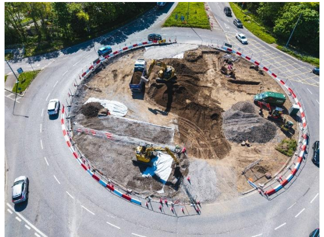
Works at Estuary Roundabout & Trench Boxes installed for Foul Sewer
