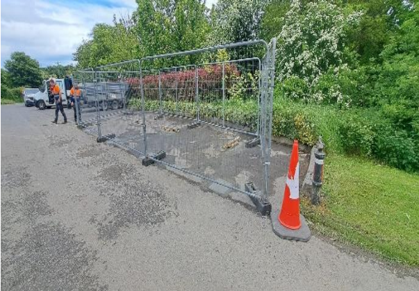
Landscaping works in Ballyboughal.
