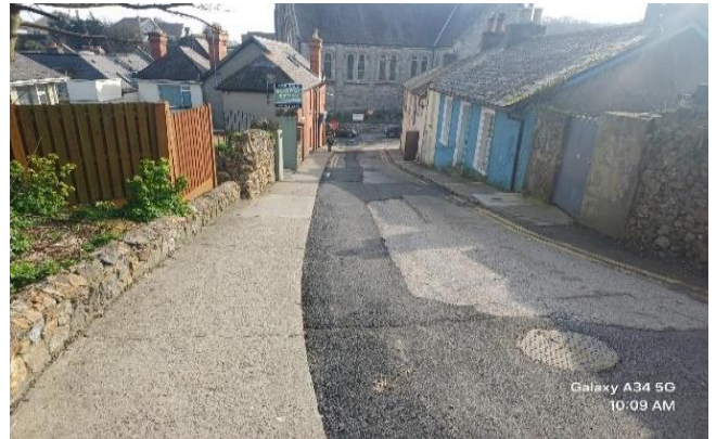
Tuckett's Lane works
