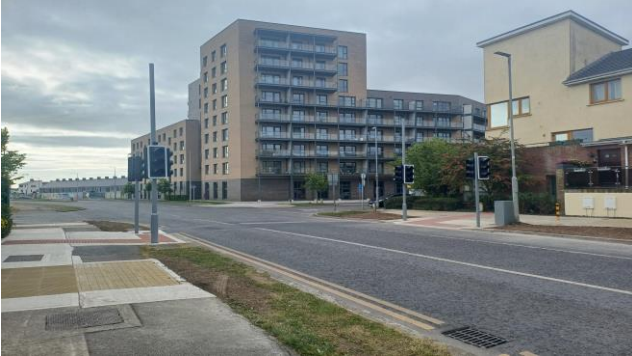
New pedestrian crossing being constructed on St Margarets Road in Dublin 11.
