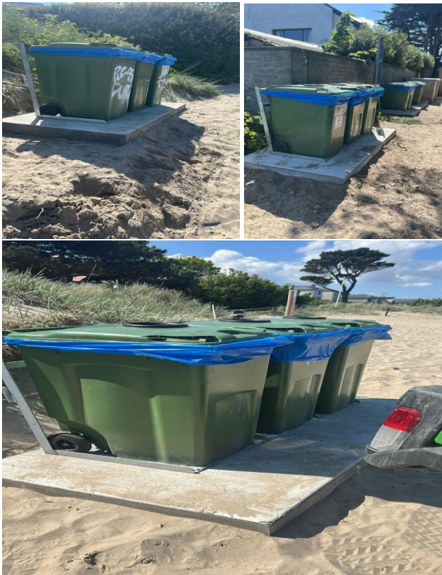
Installation of new bin bases Howth Malahide.
