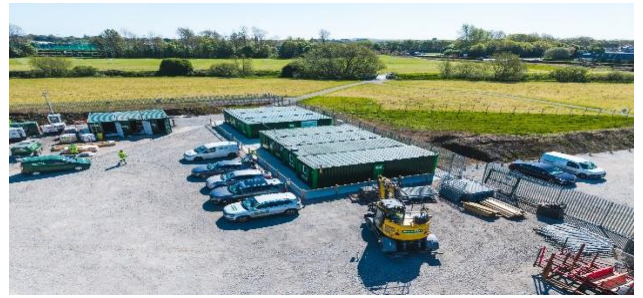
Site Compound Establishment
