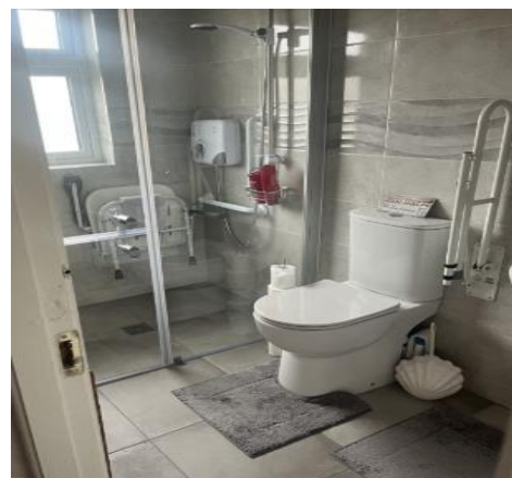
Recently completed bathroom adaptation works
