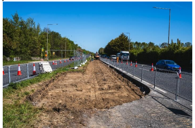
Works at Bostik for the New Bostik Junction
