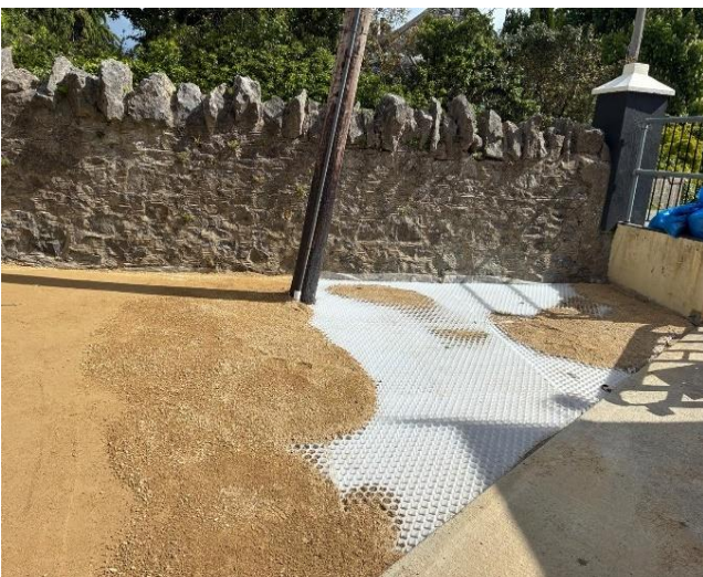
Resurfacing works complete in Oldtown, part of our Programme of Works.
