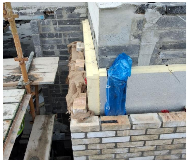
Checking vertical fire stopping and insulation on apartments in Skerries.
