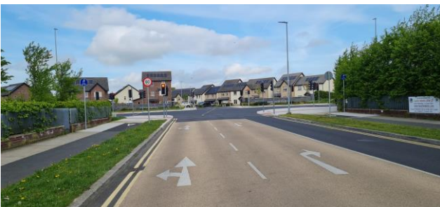
60kph sign installed on Barnwell Road.
