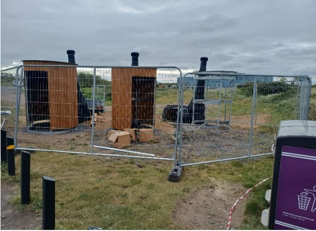
New Eco Toilets being installed in Donabate.
