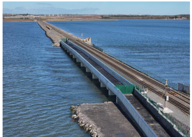
New estuary bridge and ramps looking northwards towards Donabate
