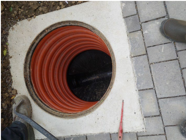
Checking drainage depths on site in Garristown.
