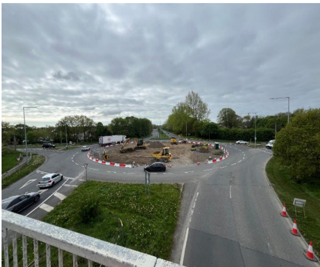
Works at Estuary Roundabout
