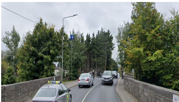
Existing footpaths at Granard Bridge
