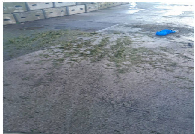
Annual deep cleaning of the Depot Wash Bay.
