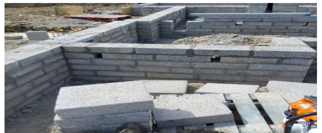
Checking Rising walls on a house in balbriggan
