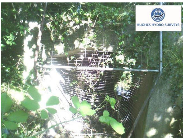
Figure 4-15 Downstream Inlet Culvert 7
