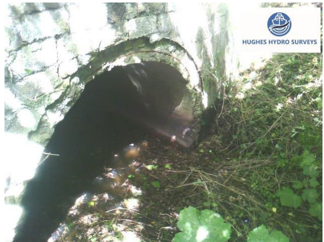
Figure 4-19 Upstream Inlet Culvert 9
