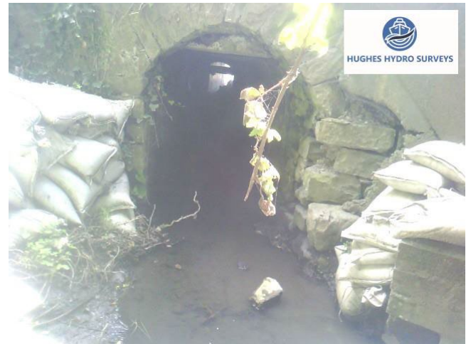
Figure 4-8 Upstream Inlet Culvert 2 - Arch
