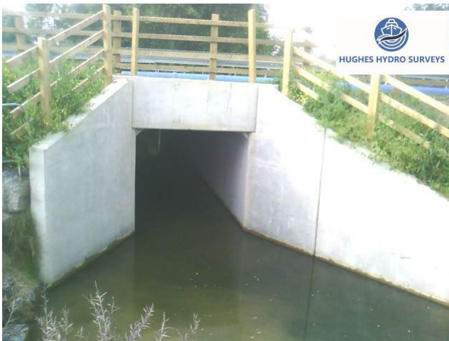
Figure 4-12 Upstream Inlet Culvert 4
