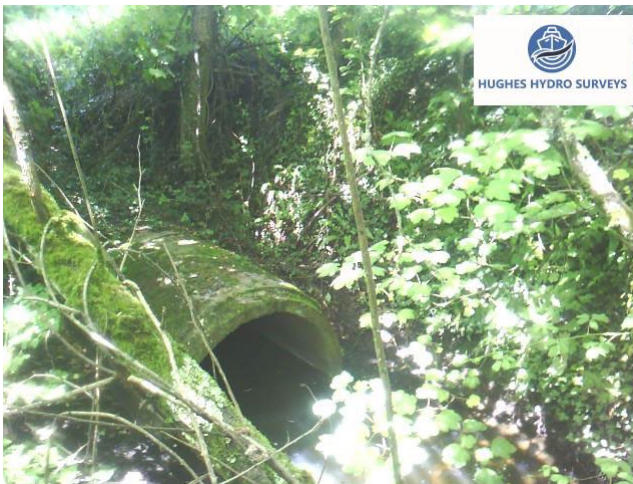
Figure 4-18 Downstream Inlet Culvert 9
