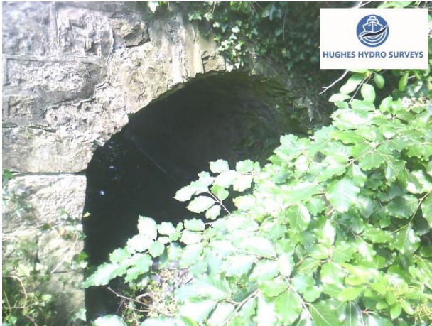
Figure 4-14 Downstream Inlet Culvert 5
