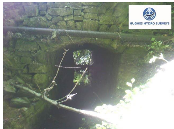
Figure 4-16 Upstream Inlet Culvert 7
