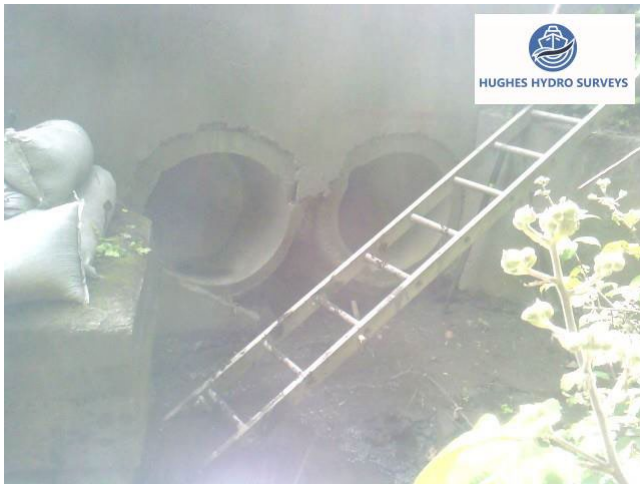
Figure 4-7 Upstream Inlet Culvert 2 - Twin Circular Culverts
