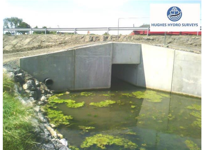
Figure 4-11 Downstream Inlet Culvert 3
