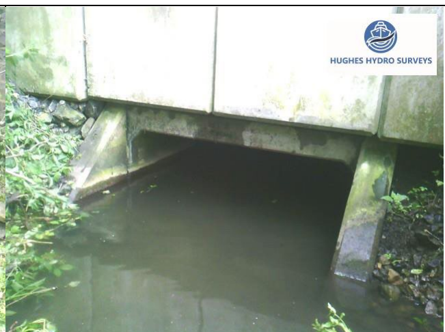
Figure 4-6 Upgraded Canal/Railway Culvert – Downstream Inlet (Hughes Hydro Surveys, 2025)
