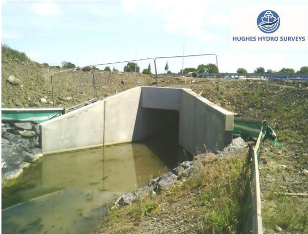
Figure 4-10 Upstream Inlet Culvert 3
