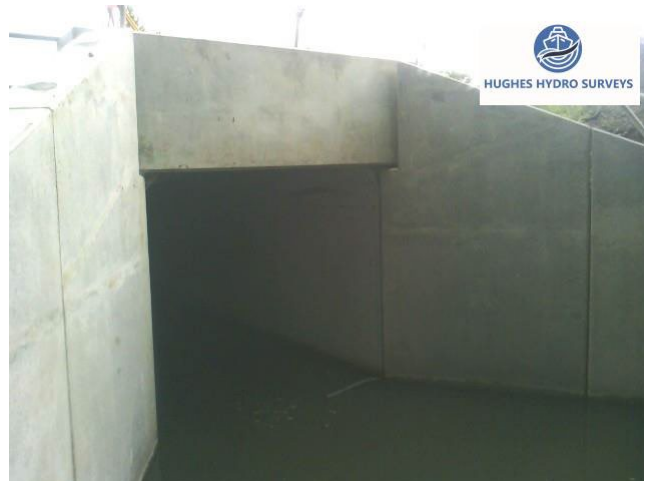
Figure 4-13 Downstream Inlet Culvert 4
