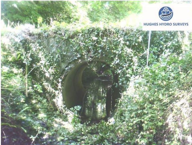
Figure 4-17 Downstream Inlet Culvert 8
