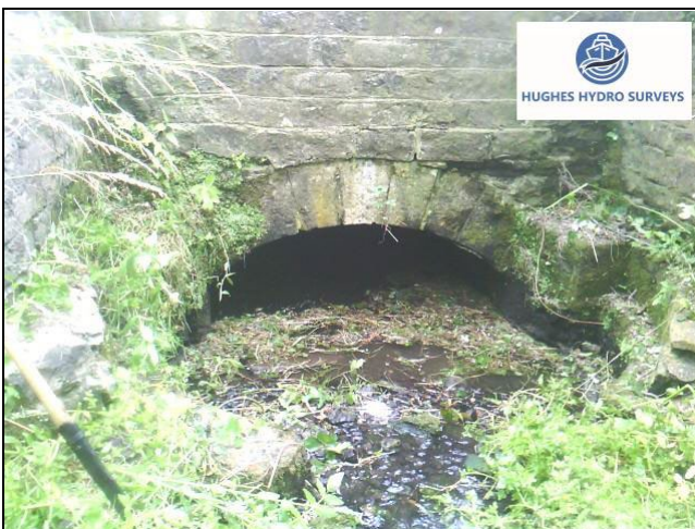
Figure 4-5 Upstream Inlet Canal/Railway Culvert (Hughes Hydro Surveys, 2025)
