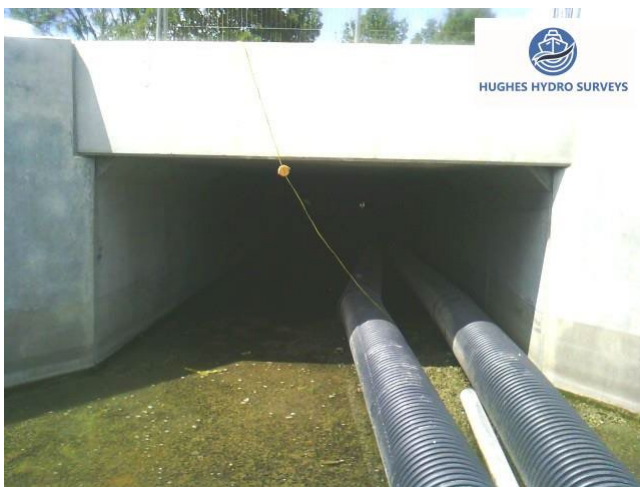
Figure 4-9 Downstream Inlet Culvert 2 - Extended Culvert Box
