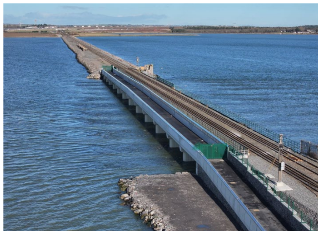
New estuary bridge and ramps looking northwards towards Donabate
