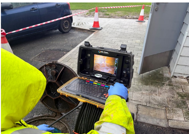
Jetting and clearing foul sewer serving the public toilets opposite Howth Market.
