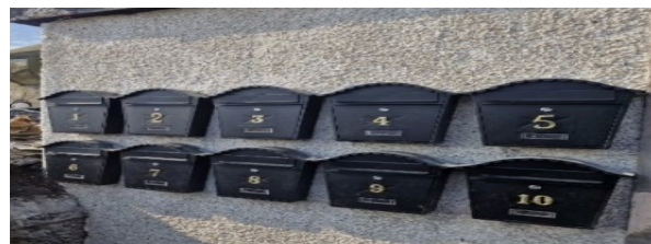
Installation of Post boxes at Moyne Park
