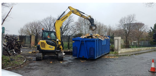
Waste removal at St. Philomena's Park
