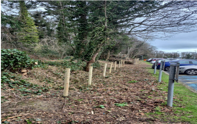
New fencing installed along perimeter of carpark.
