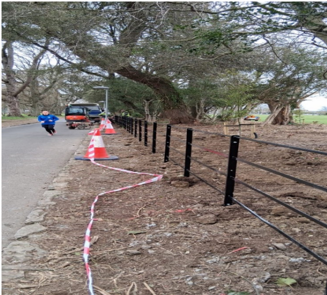
New fencing installed along the main avenue.
