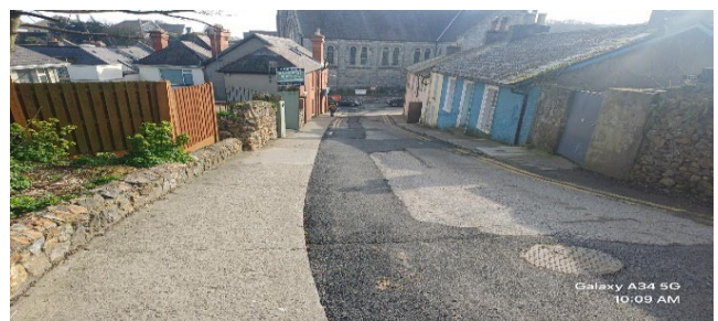
Tuckett's Lane works
