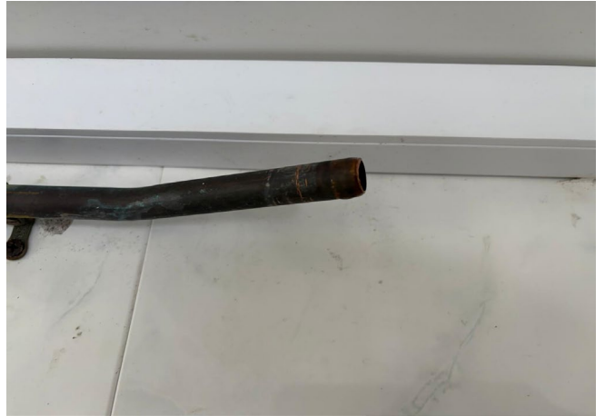
Robswall wall toilets Malahide new plumbing fittings installed to address leaking issue.
