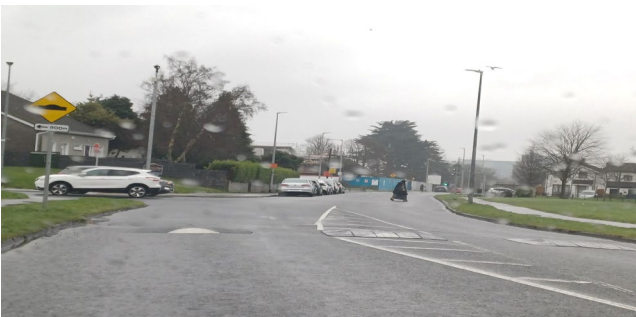
Left speed cushion replaced on Blackcourt Road.
