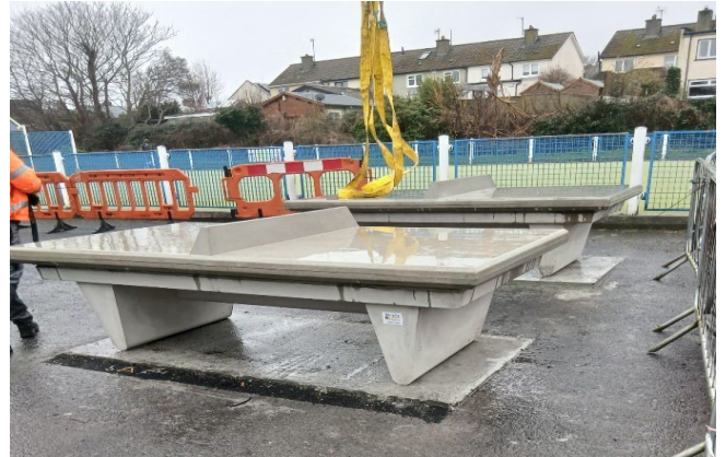
Plinths and ping-pong tables installed adjacent to the MUGA in Grace O'Malley.
