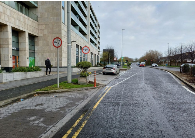
New hardstanding area installed for drop off/pick up passengers outside the Charlestown Shopping Centre.
