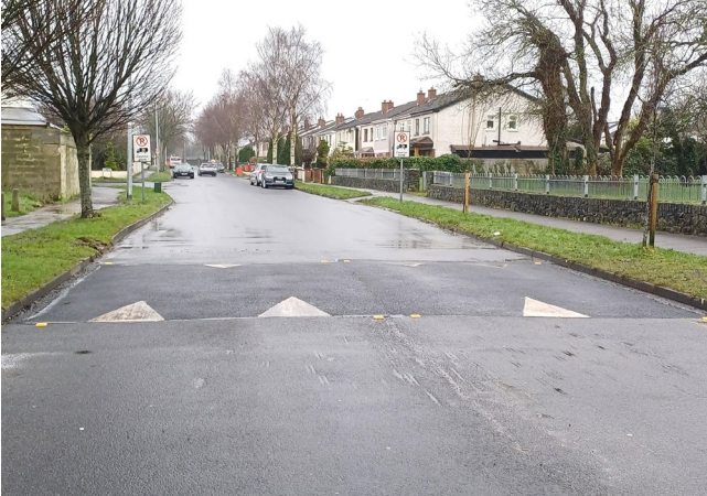
Traffic Calming Ramp replaced on Lohunda Downs.
