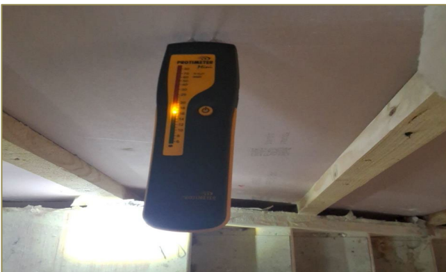
Checking plasterboard moisture content on a site in Malahide
