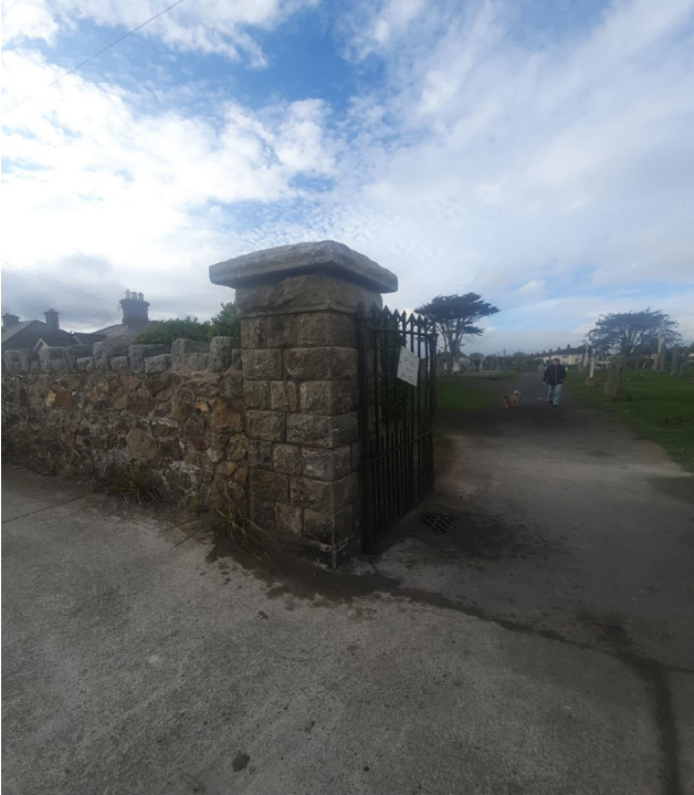
Entrance to Kilbarrack burial grounds rebuilding of pillars and refitting of gates following collapse due to storm damage.
