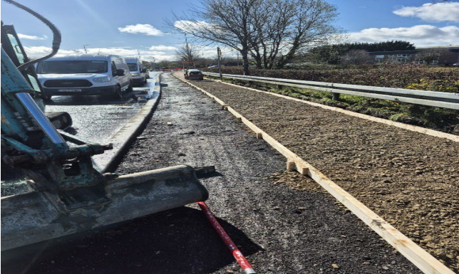
Footpath and cycle track renewal work on Stephenstown by-pass in Balbriggan as part of Area Engineer's general maintenance works.
