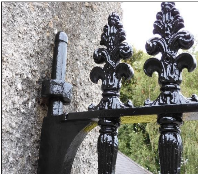
BHIS – Repair of decorative cast-iron gates, Donabate
