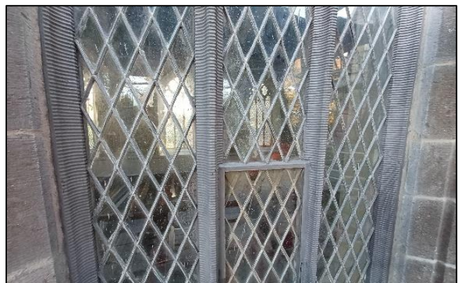
HSF - Repaired Window Tracery – St Columbas Church, Swords
