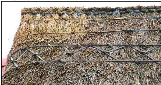
SIT Project – Repair to the twisted bobbin ridge and spraying bluestone treatment on a thatched house roof, Fingal 2025
