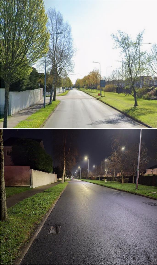
Lohunda Road Column Replacement and Cable Works. Existing lighting removed and new Lighting Scheme and cabling installed on opposite side of road. Before and After
