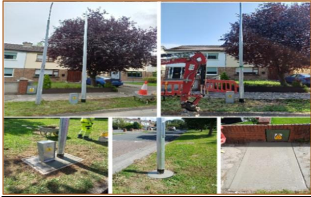
Lohunda Road Column Replacement and Cable Works. Existing lighting removed and new Lighting Scheme and cabling installed on opposite side of road. Before and After
