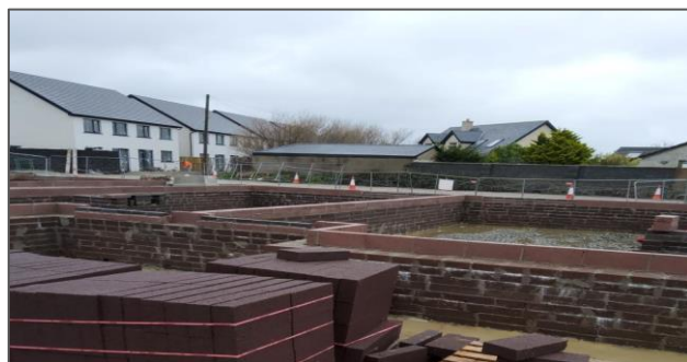
Checking foundations and rising walls on a development in Rush.
