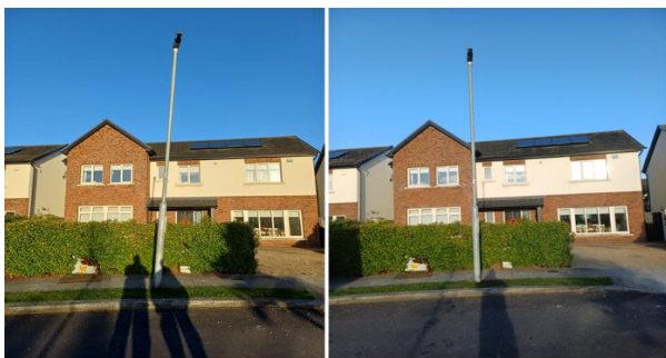
Leaning Column straightened
