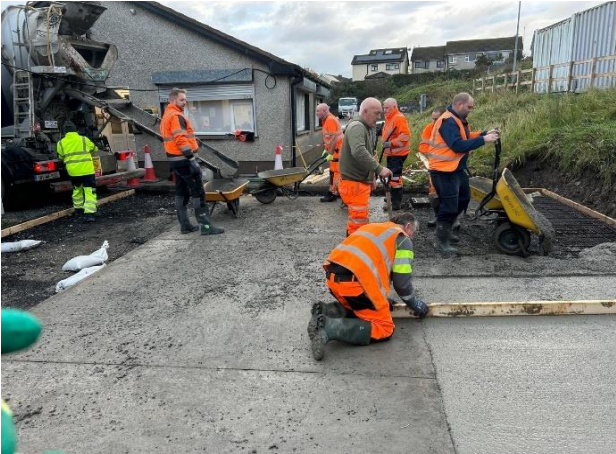
New concrete bases installed for new office at Fancourt Depot.
