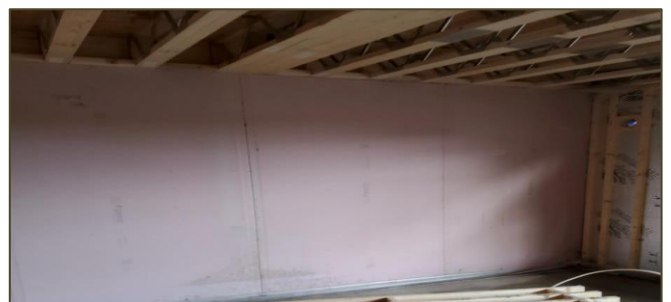
Checking ceiling joist and party wall on a development in Dublin 15
