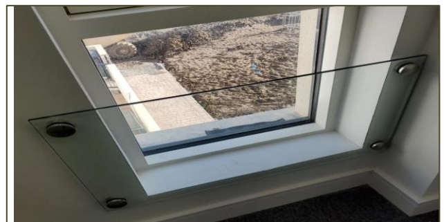
Checking Guarding in front of a low window on a development in Donabate
