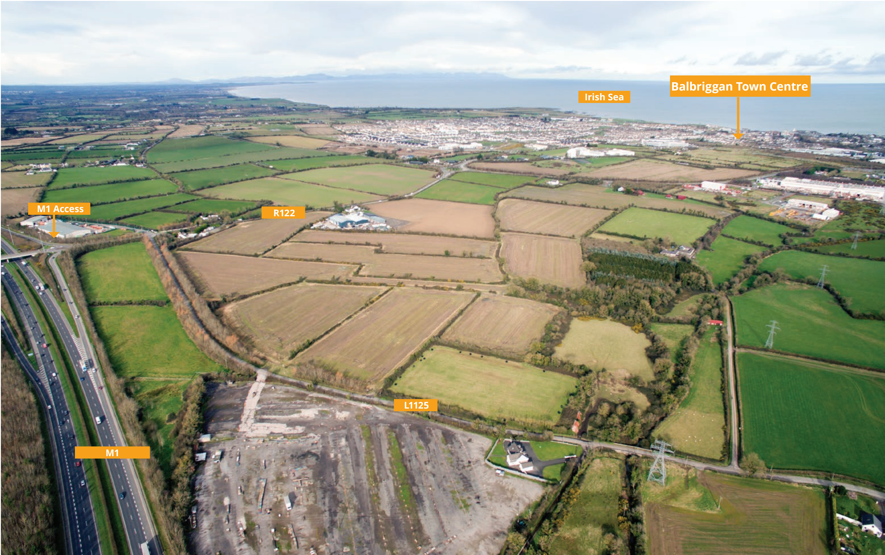
Aerial view of the Framework Plan Lands looking north from above M1 Motorway
