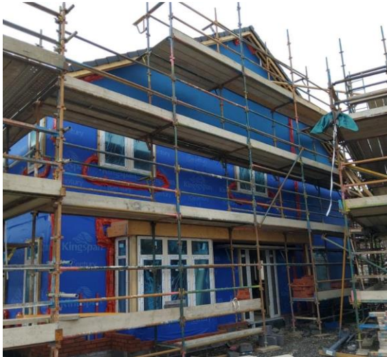
Checking Firestopping around windows and doors in a timber frame house in Dublin 15
