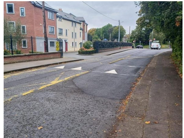
New ramp on Beechpark Avenue.
