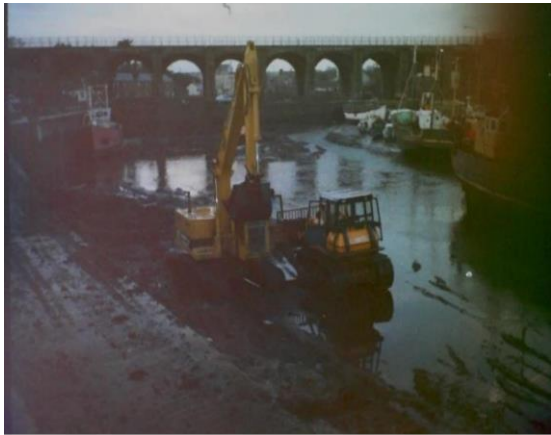
Photos show previous maintenance dredging undertaken in 1996.
