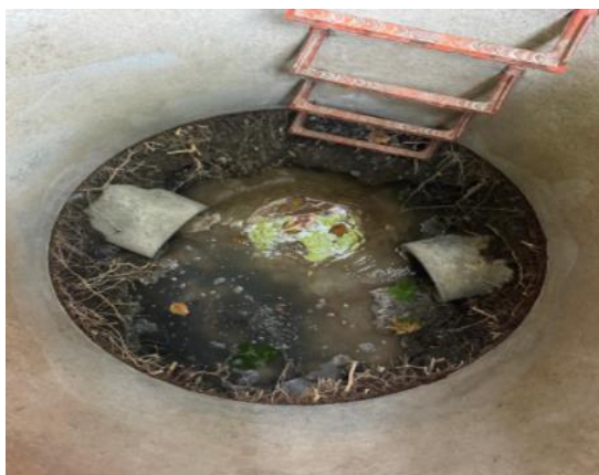
Survey in Coolmine.
