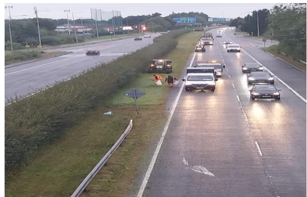
N3 Navan Road Grass cutting.
