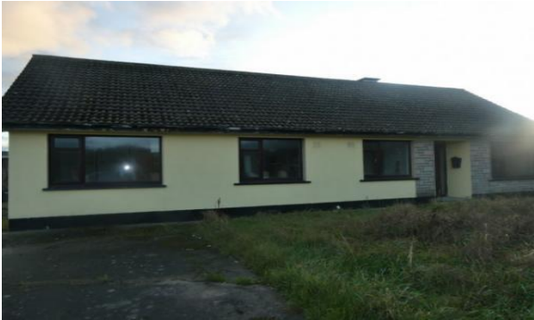
Works complete Property - Before and after
