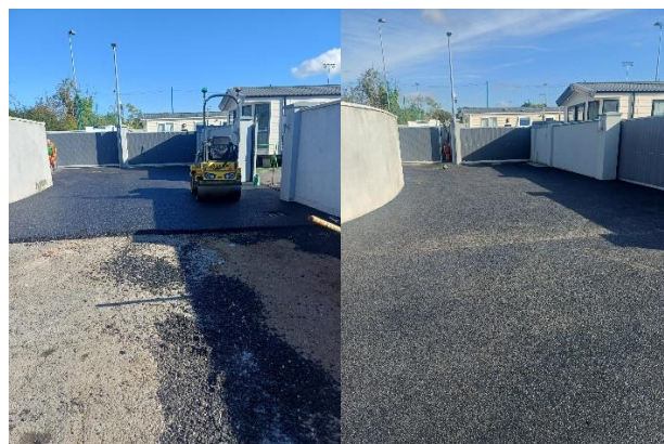
New tarmac laid in Saint Brigid's Lawn, Porterstown
