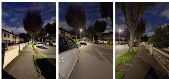
Lohunda Park after Column Replacements.
