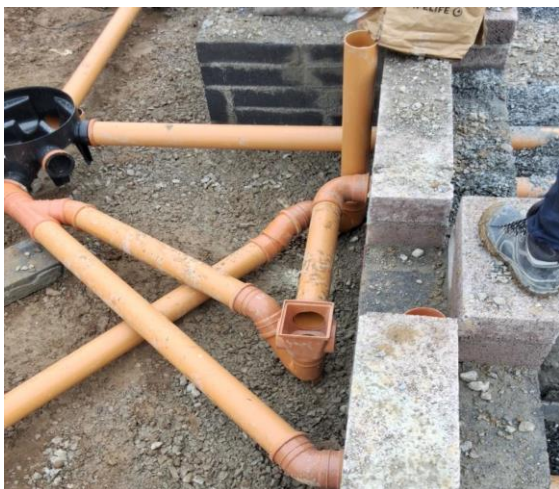
Checking foundations and drainage in duplex units in Skerries
