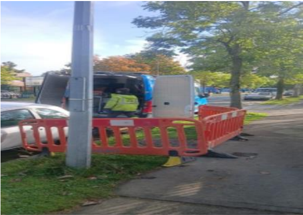
Survey in Coolmine
