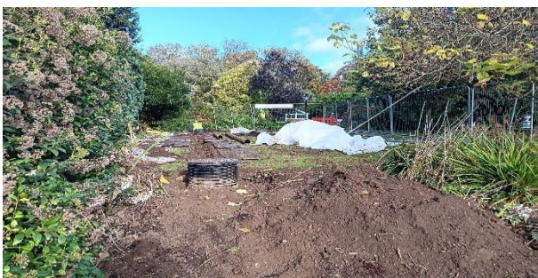
Drainage lines between pond and Dutch house.
