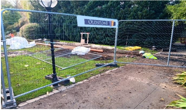
Drainage works to facilitate rainwater from Peach house and Dutch house.
