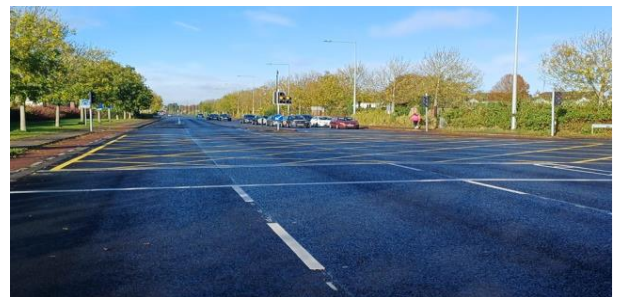
Yellow box installed at the junction of Ongar Distributor Road//Hartstown Link Road.
