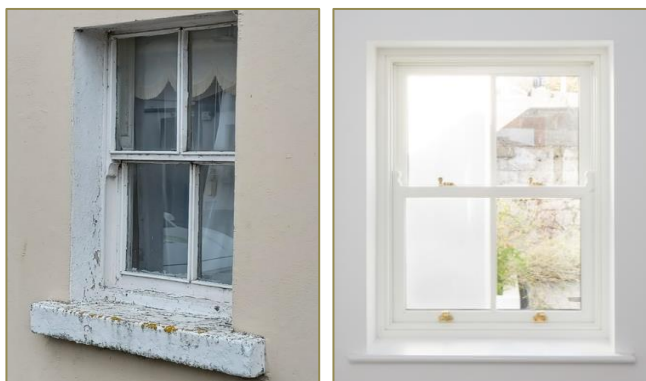
Figure 5 BEFORE and AFTER - Sash windows upgrade
