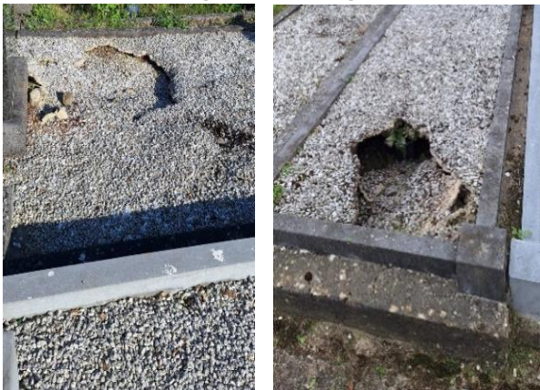
Work being carried out to remediate grave subsidence at Balgriffin Burial grounds
