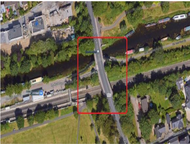
Granard Bridge Site location
