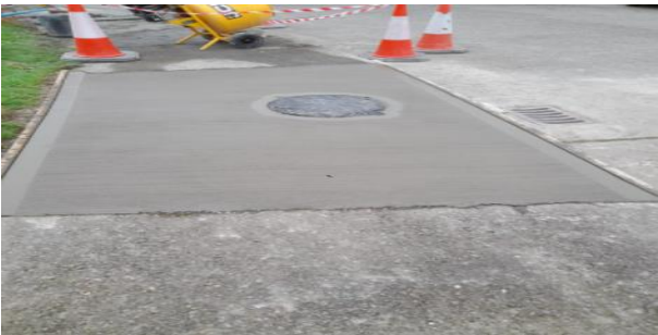
MH cover replacement, Loughshinney
