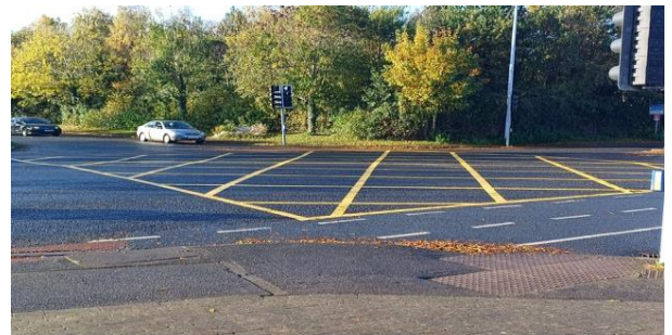
Yellow box installed at the junction of Ongar Distributor Road/Shelerin Road
