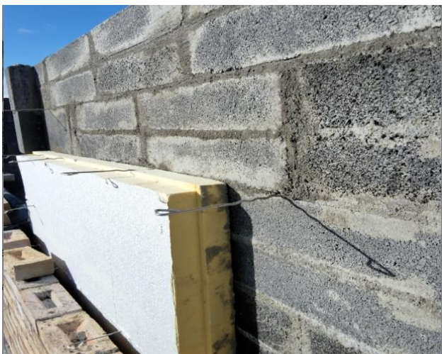
Checking Insulation in a duplex building in Kinsealy
