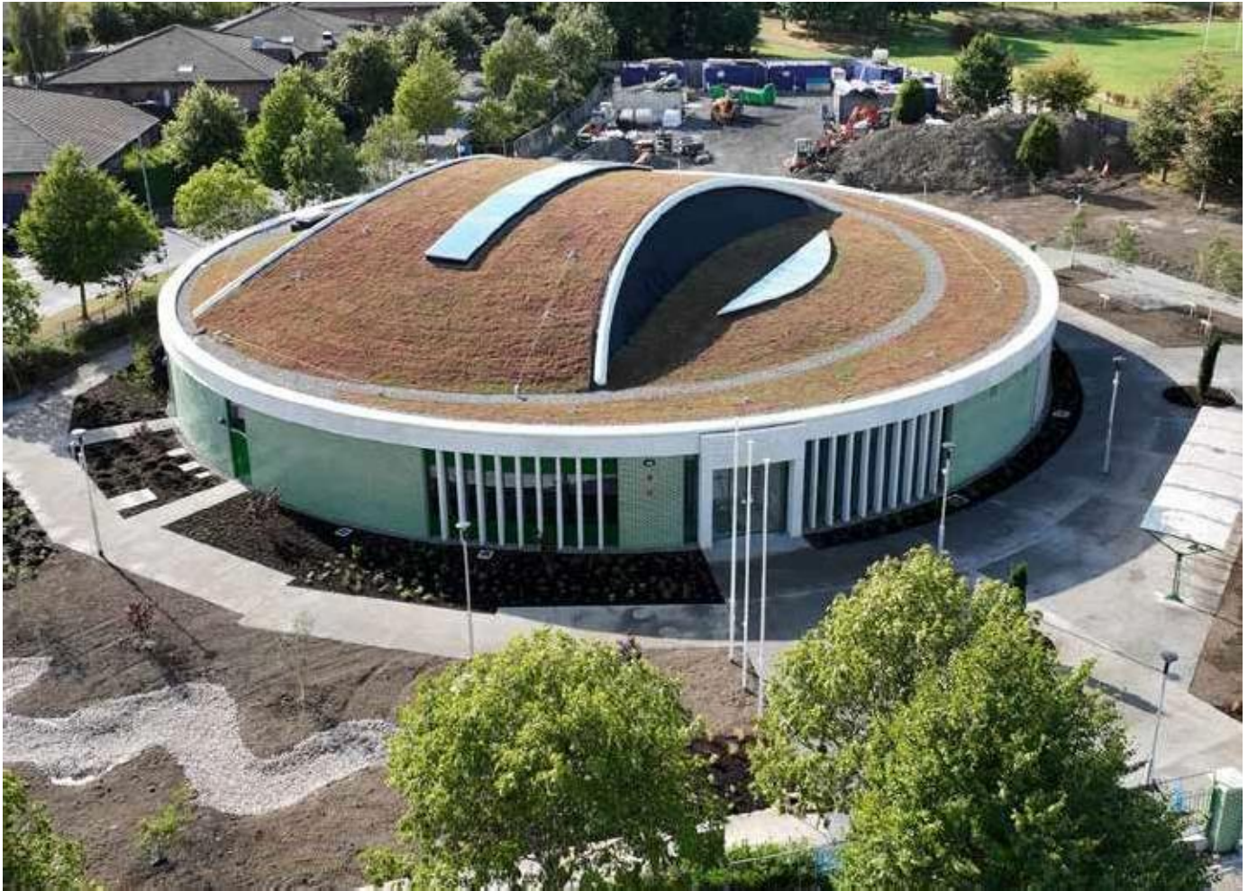
Meakstown Community Centre at Lanesborough Park
