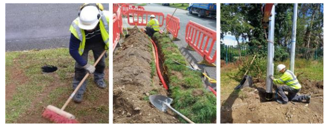
Installation of column sleeves, ducting and new public lighting columns, Lohunda Estate
