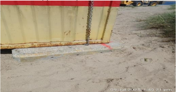
Below - Life guard huts Howth / Malahide concrete supports in place
