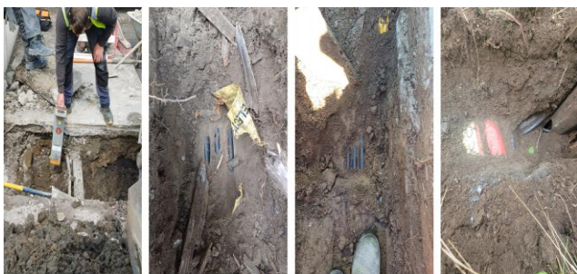
Cable location of ESB supply cables into public lighting columns, Lohunda Estate
