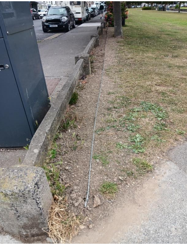
Above and below - Steel edging installed along the green open space at Howth harbour front.
