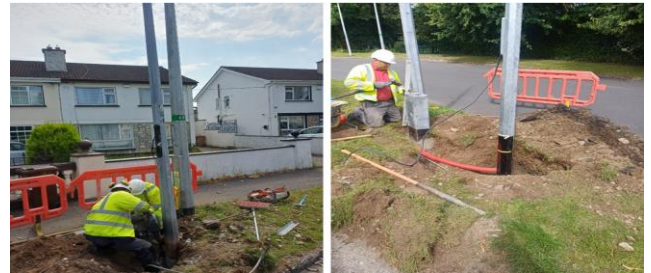
Transferring of ESB supply cables into new columns and section pillars, Lohunda Estate
