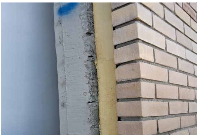
Checking Insulation in a wall of an apartment block in Rush
