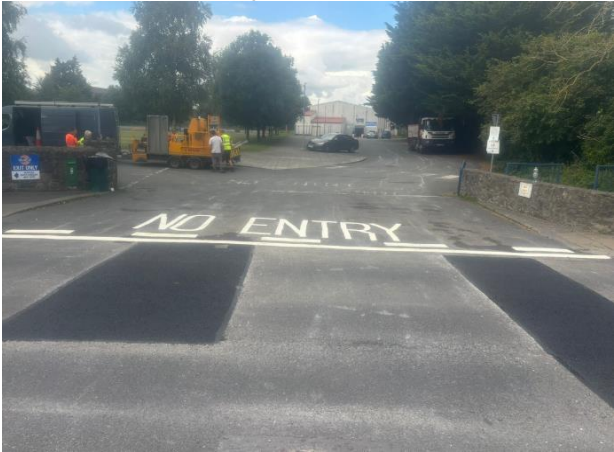
Ramp repair and new lining by car park exit of Malahide community school.
