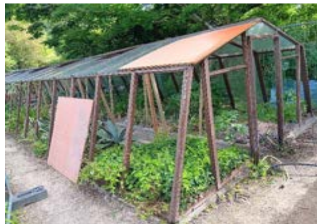
Glass panels removed from Old Dutch Glasshouse before restoration
