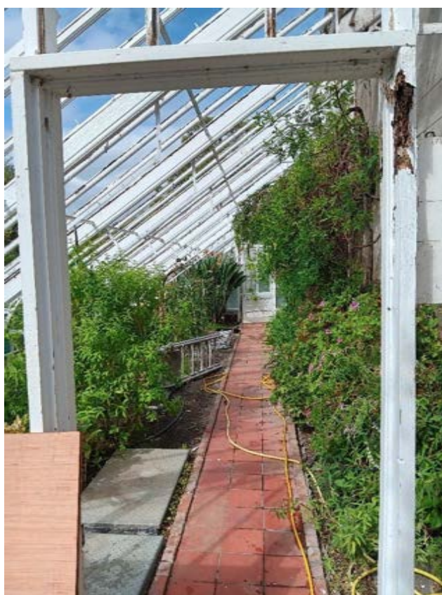
Peach House – Works have begun on the glass houses. Glass panels removed prior to restoration works.
