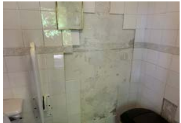
Works to be carried out to replace loose tiles at Malahide village toilets.
