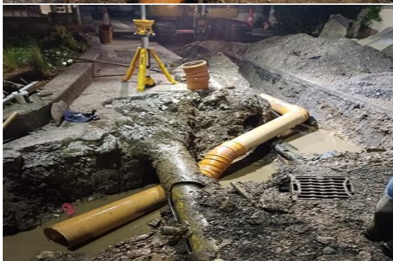
Replacement of Defective Drainage on Church Street and Harbour Road Howth as part of the 2025 POW.
