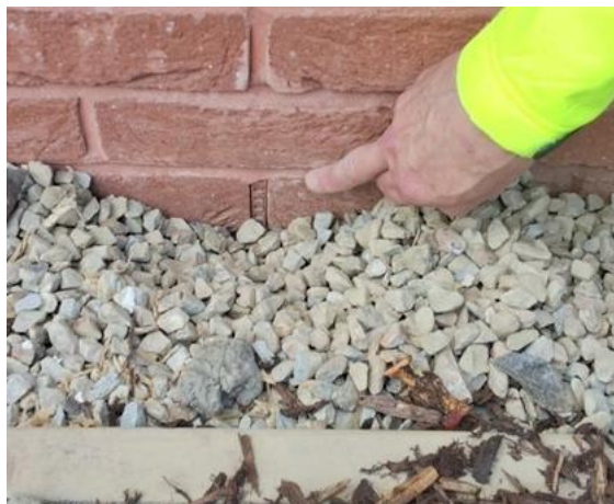
Checking weephole location on an house in Portmarnock
