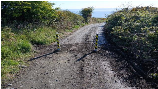
New removable bollards installed on pathways Howth to prevent unauthorised access.
