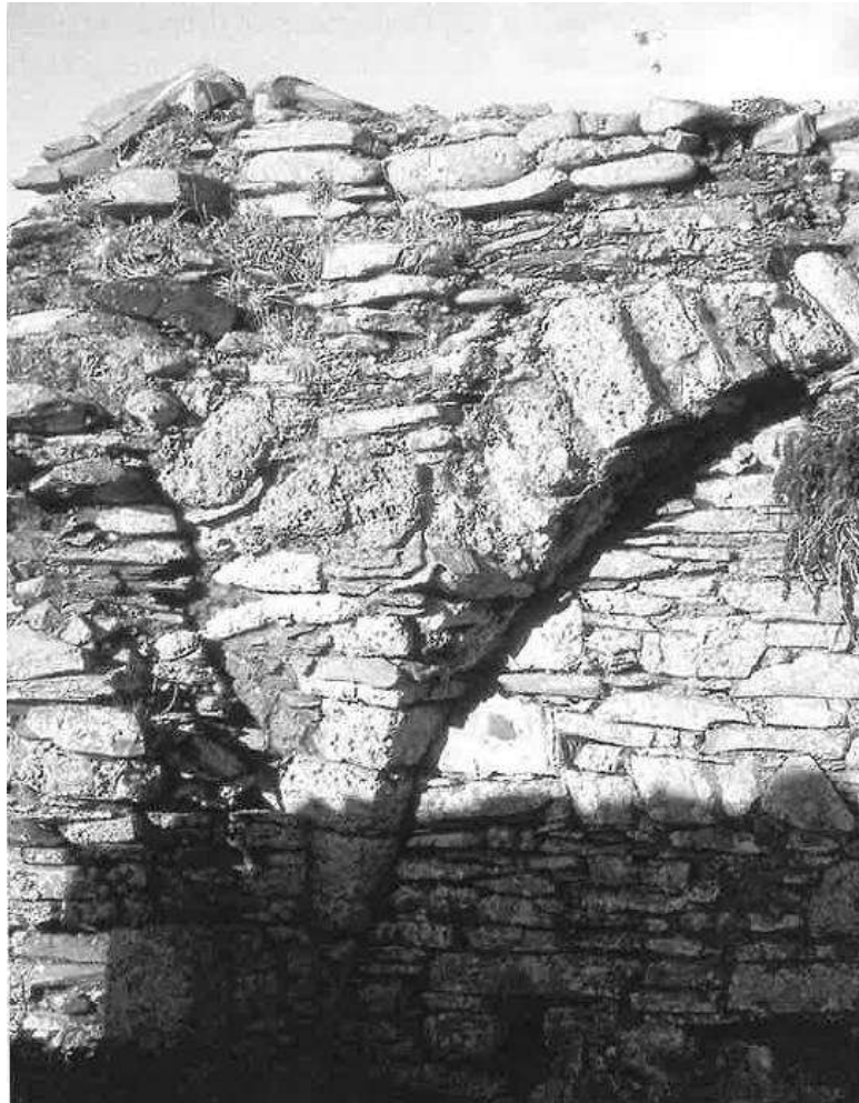
PLATE 38: Shaped tufa voussoirs at St Patrick's Church, Skerries (Ryan et al 2004)
