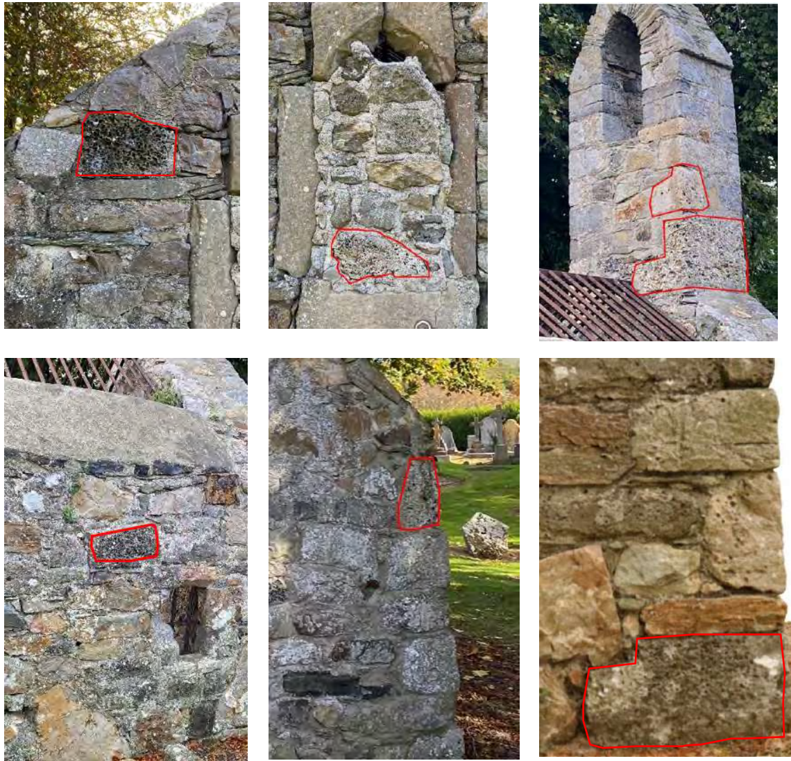
PLATES 6A-F: Clockwise from top left, wedge-shaped tufa blocks in a) eastern gable; b) eastern window infill; c) bellcote; d) northern wall; e) western gable and f) notched/rebated southeastern quoin
