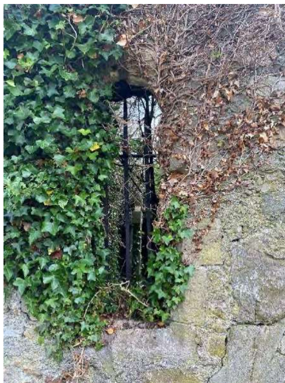
PLATE 14: Dundry Stone lancet headed window in north wall of chancel, Kilbarrack Church
