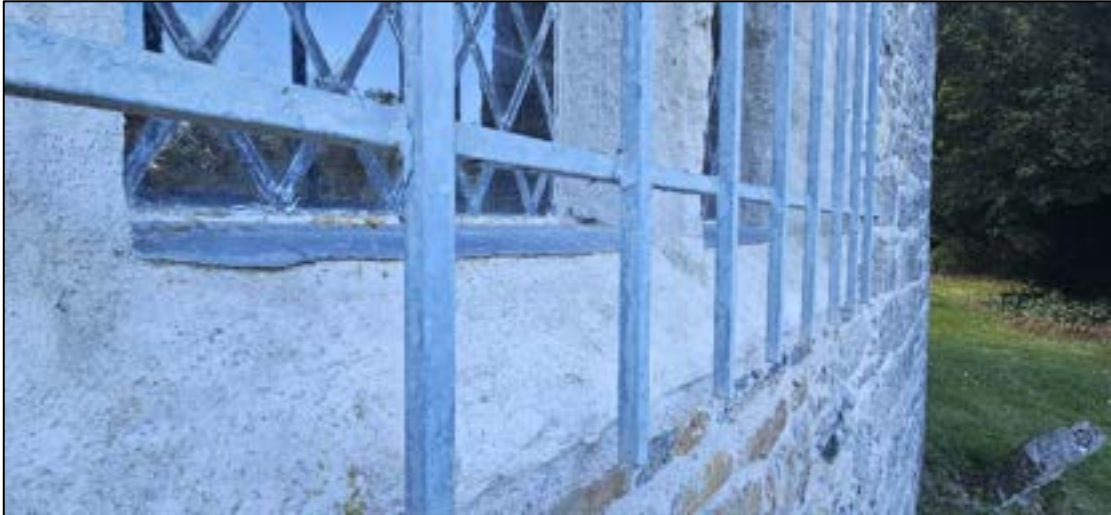
Plate 8: The details on the cill show that the shelter coat consisted of lime with a sand filler to provide thickness and stability to the shelter coat.
