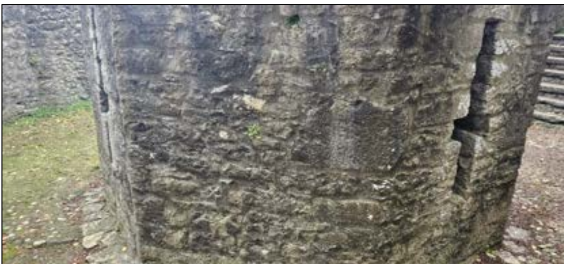
Plate 34: Detail of pointing on wall of Baptistry, facing east.
