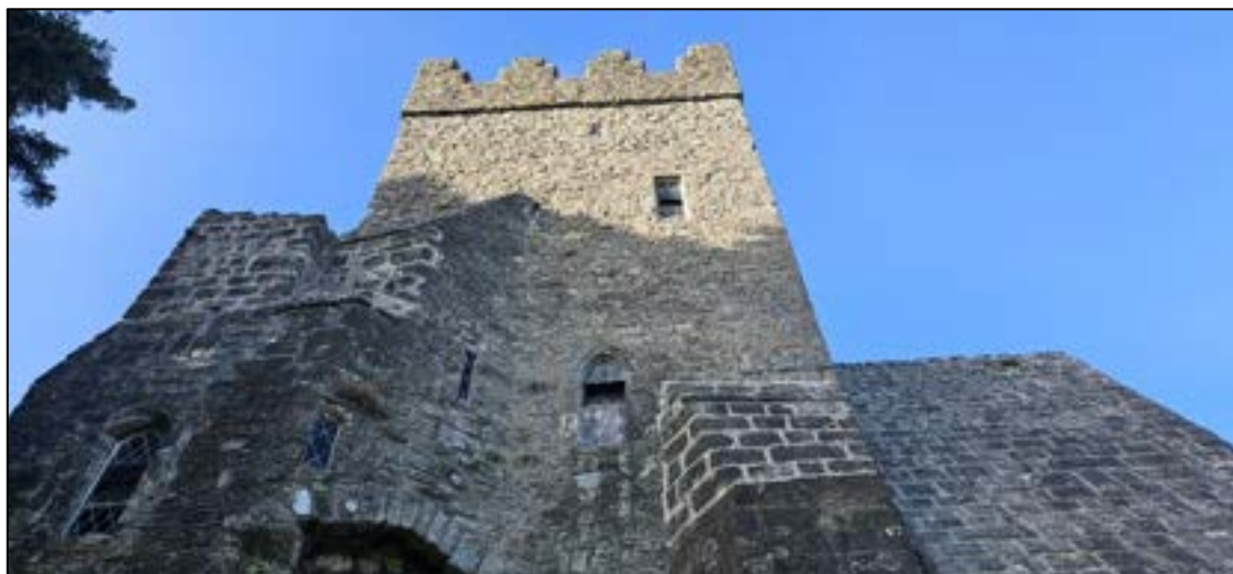
Plate 3: Detail of repointing works to tower, facing upwards to east.
