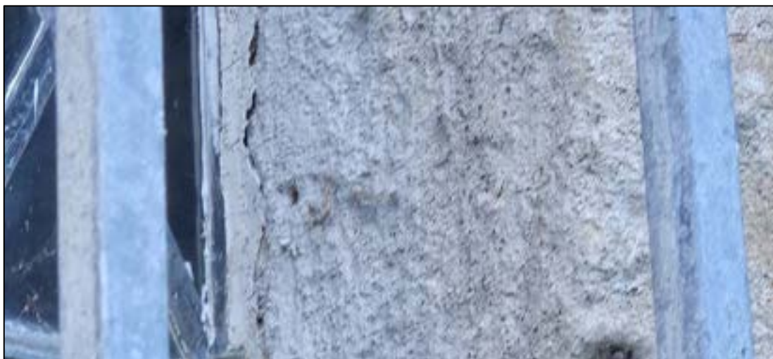
Plate 17: The sandstone appears more friable than the surrounding pointing.
