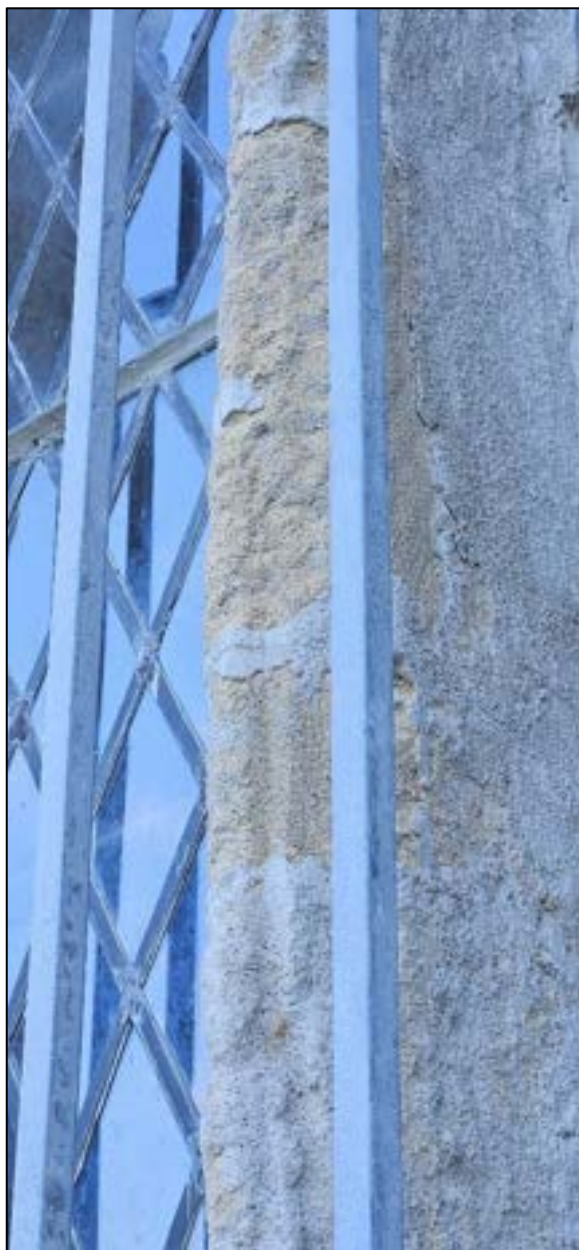
Plate 12: This image demonstrates how the parent and shelter coat are harder than the parent sandstone.
