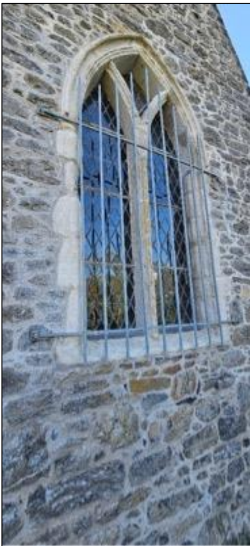
Plate 7: During the 2018 conservation works a shelter coat was applied to the east window to the chancel.
