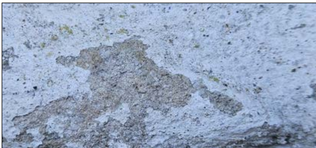
Plate 14: Decay on the sandstone cill shows parent material is likely to spall if not treated.
