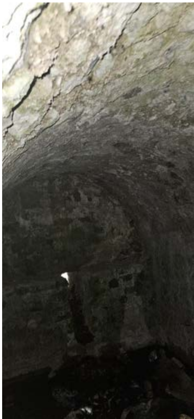
Plate 31: Decay to vault ceiling of St Catherine's Well, facing south.
