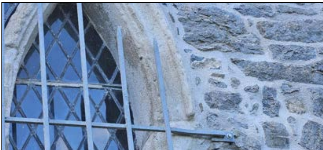
Plate 16: The pointing and deterioration of shelter coat on the northeast lancet; the adjacent lime pointing is in good condition.
