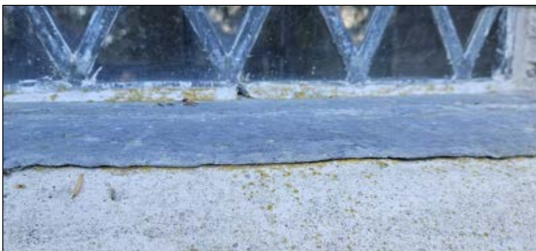
Plate 18: Minor faults in the putty should be addressed during repair.
