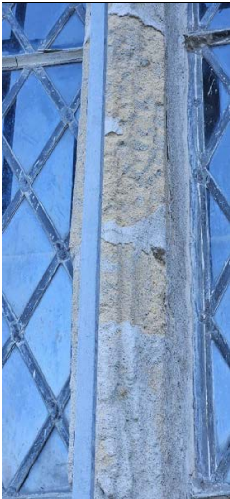
Plate 10: The central mullion shows alveolar, or honeycomb decay. The area is subject to extreme wetting and drying and salt crystallisation has caused spalling of the shelter coat.
