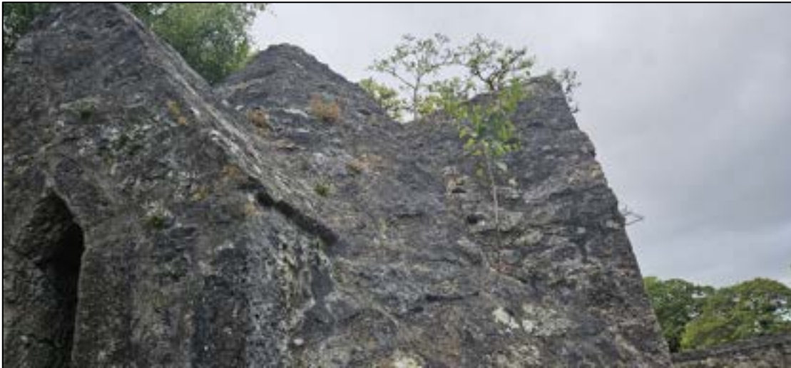
Plate 32: Vegetation growing from cracks in pointing of the Baptistry, facing northwest.
