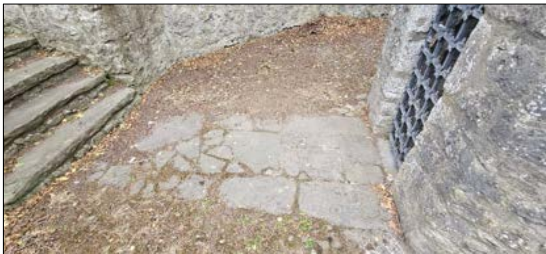
Plate 46: Damage to paving at entrance to Baptistry interior, facing west.
