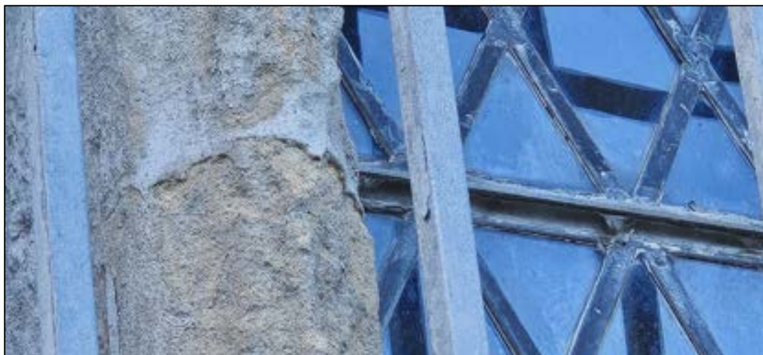
Plate 13: Secondary detail of harder parent and shelter coat.
