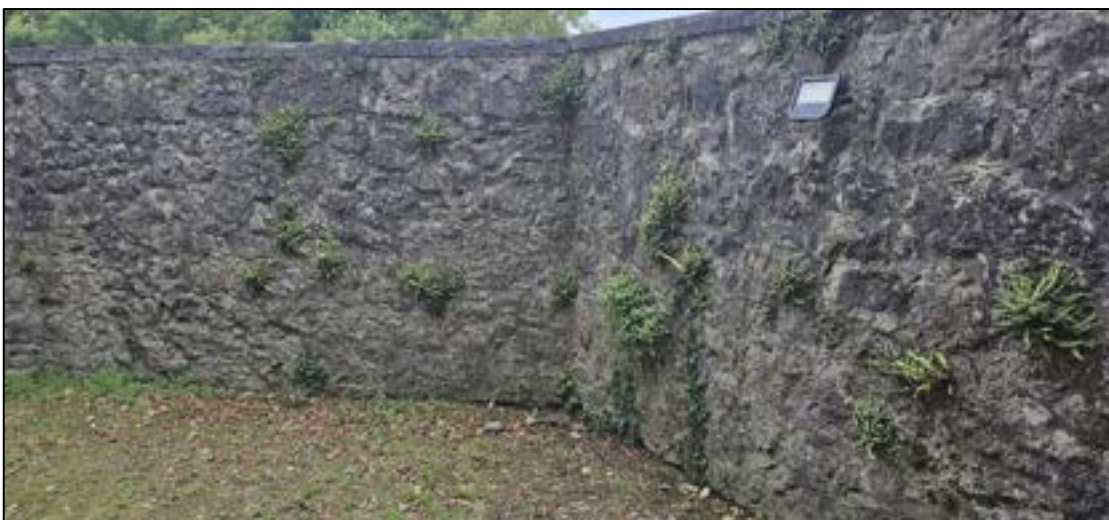
Plate 51: Vegetation on retaining walls of the Baptistry.
