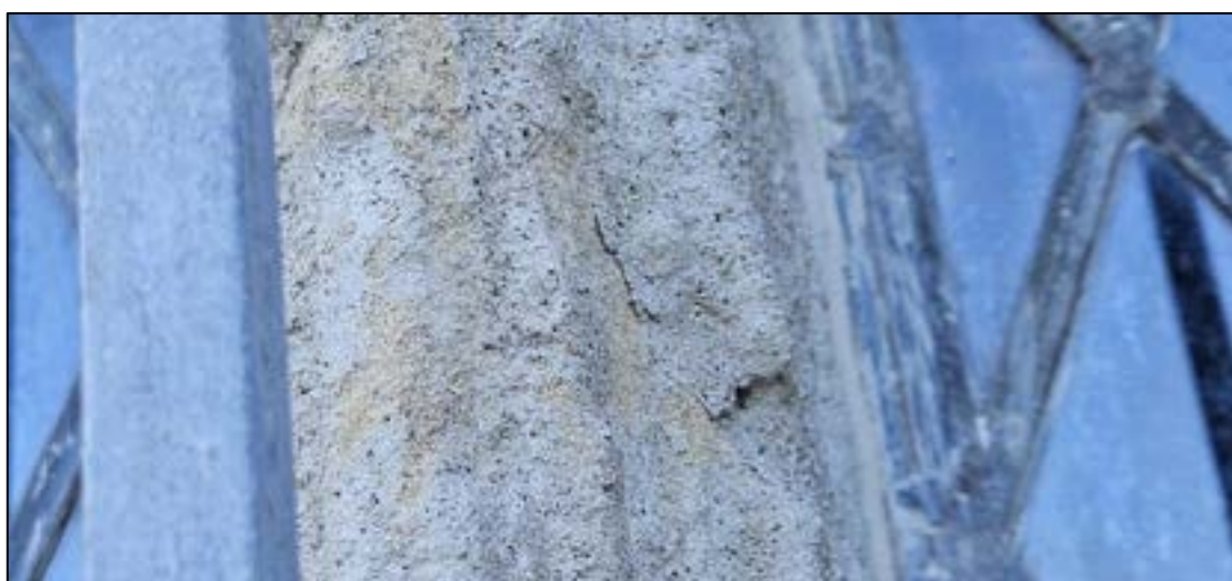
Plate 15: In one area only, cracking has occurred and material is likely to spall if not treated.
