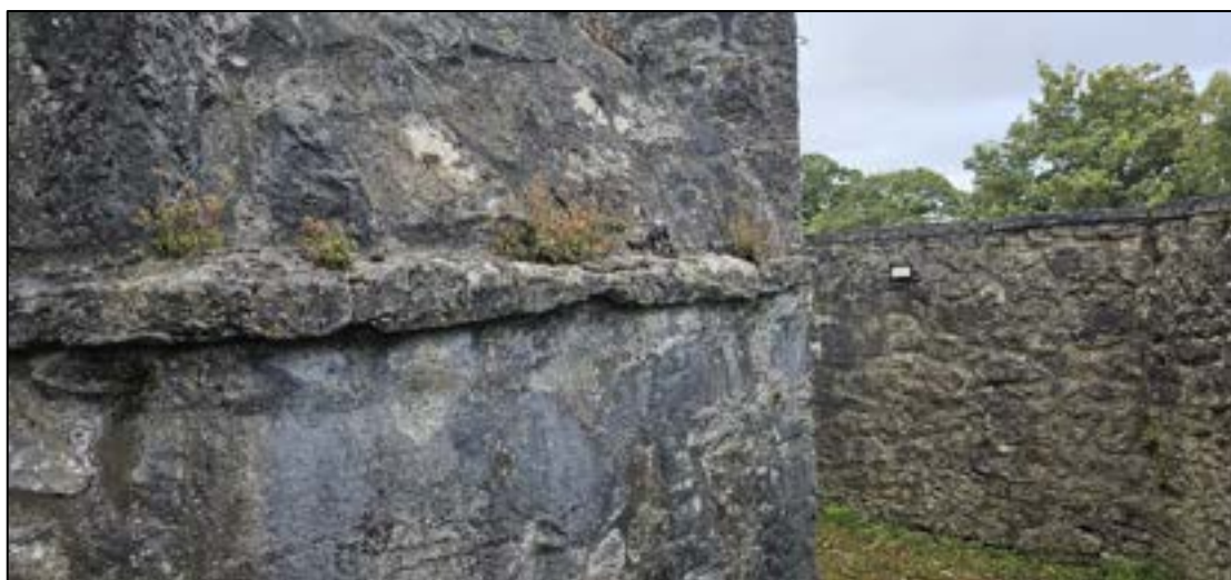
Plate 22: String course of Baptistry, which is in need of repair.
