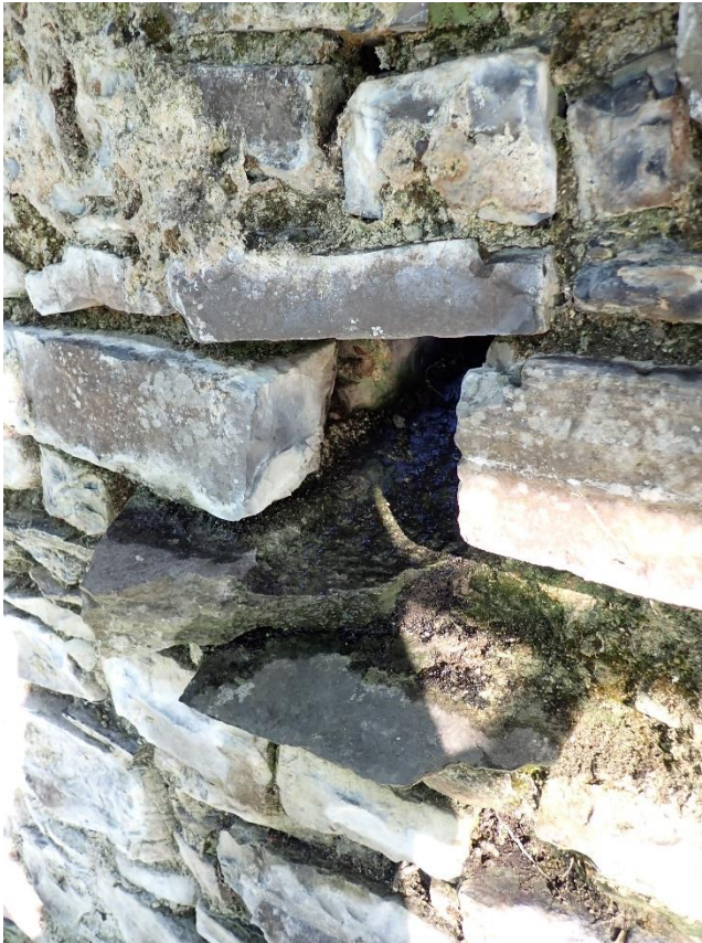
Plate 16: Damaged waterspout at north side of west wall which drains water from the north side of the flagstone roof.
