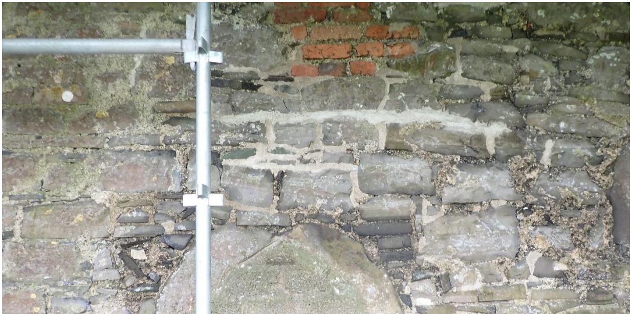
Plate 19: West wall, area above door has been stitched and re-pointed
