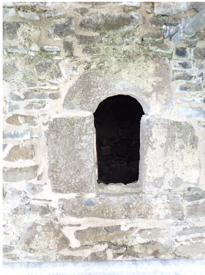
Plate 15: Round headed window to the third floor room, west wall after re-pointing
