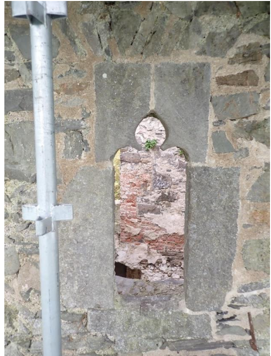
Plate 14: Trefoil headed window, north wall, before and after re-pointing. Note the off-centre keystone in the arch above
