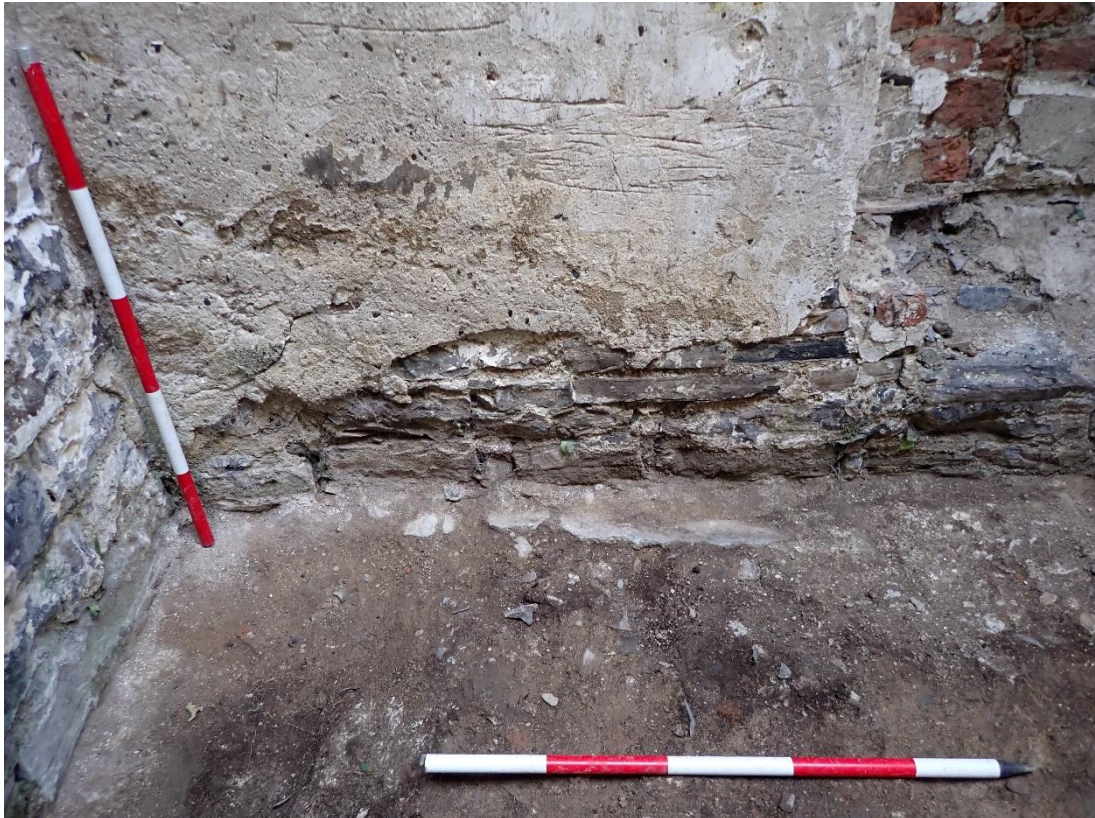
Plate 4: The NE corner, long narrow flagstones laid against the north wall, with some packed small stones towards the centre
