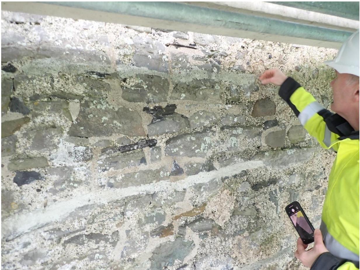
Plate 20: JK inspecting the north wall where the vertical crack was stitched and re-pointed
