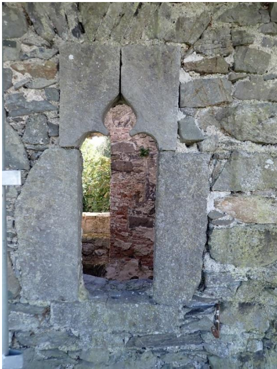
Plate 14: Trefoil headed window, north wall, before and after re-pointing. Note the off-centre keystone in the arch above
