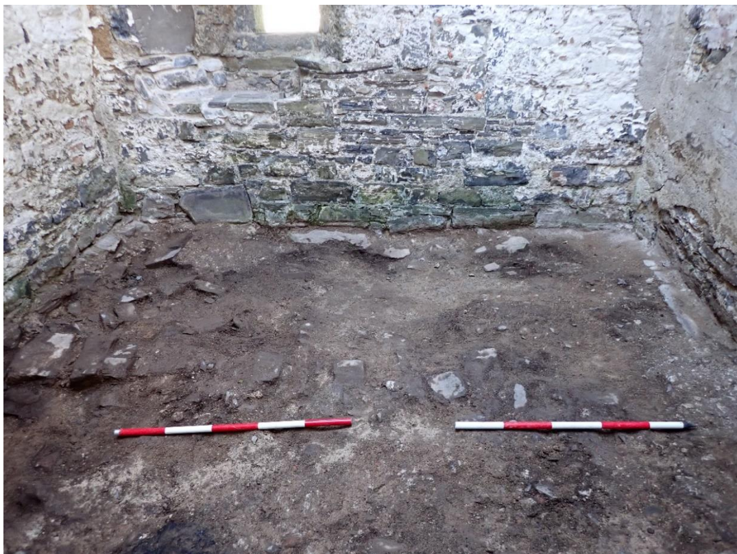
Plate 3: View looking north. Large, narrow flagstones can be seen laid along the west and north walls and the stones along the crown of the vault have been exposed
