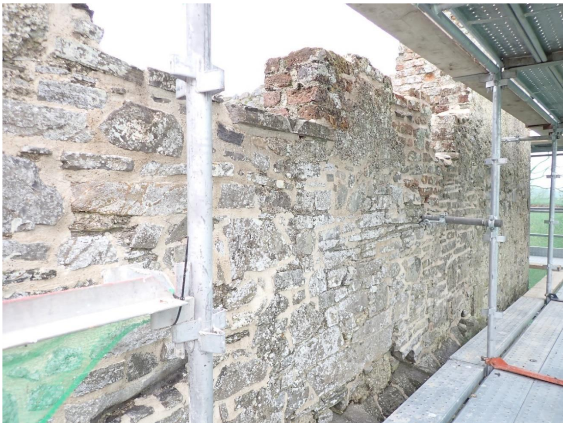
Plate 13: North wall, top floor, showing re-pointing of exterior wall and battlements
