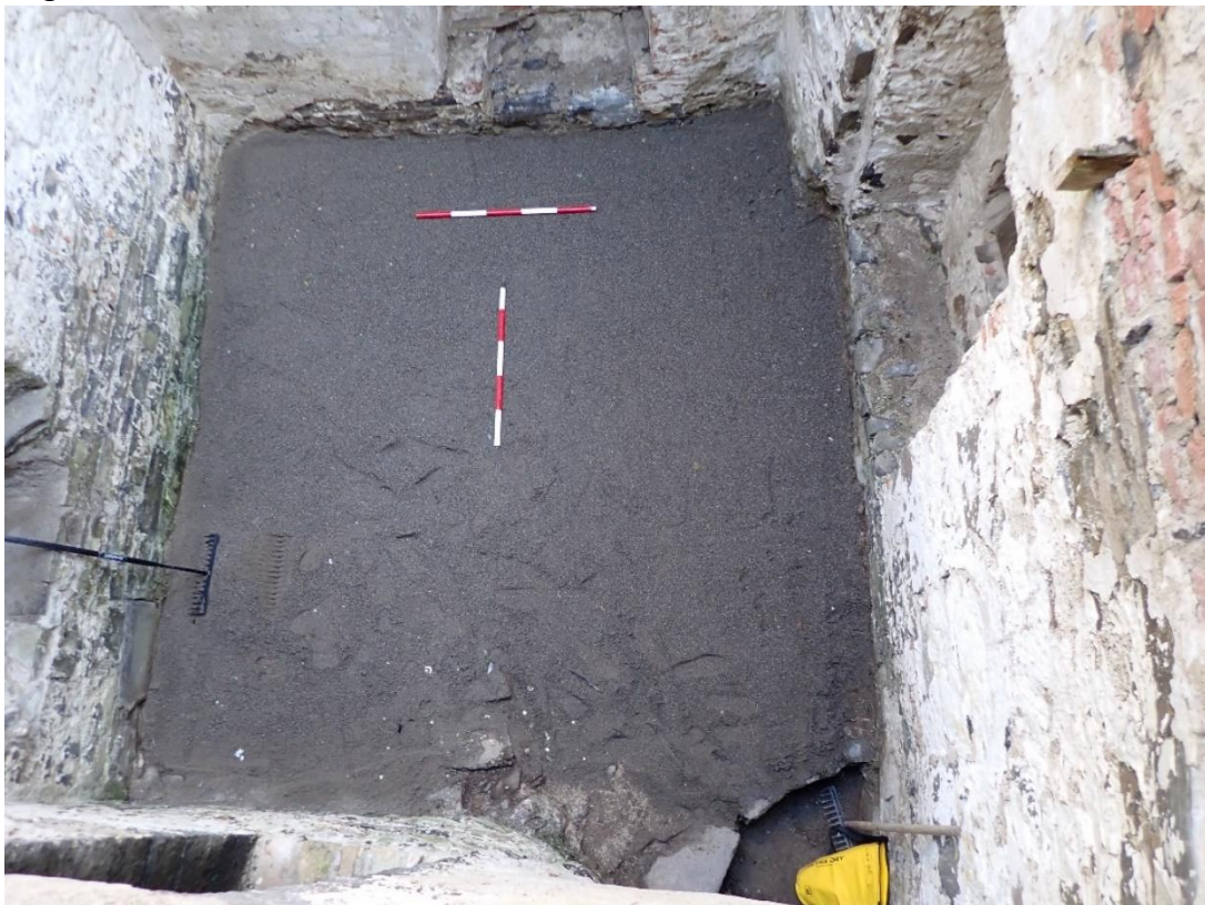
Plate 7: Sand laid on the exposed mortar to protect it
