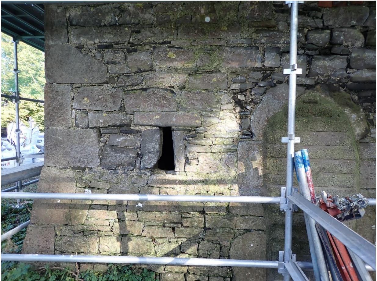
Plate 18: Lower northwest section of the west wall before conservation. Note area above door.
