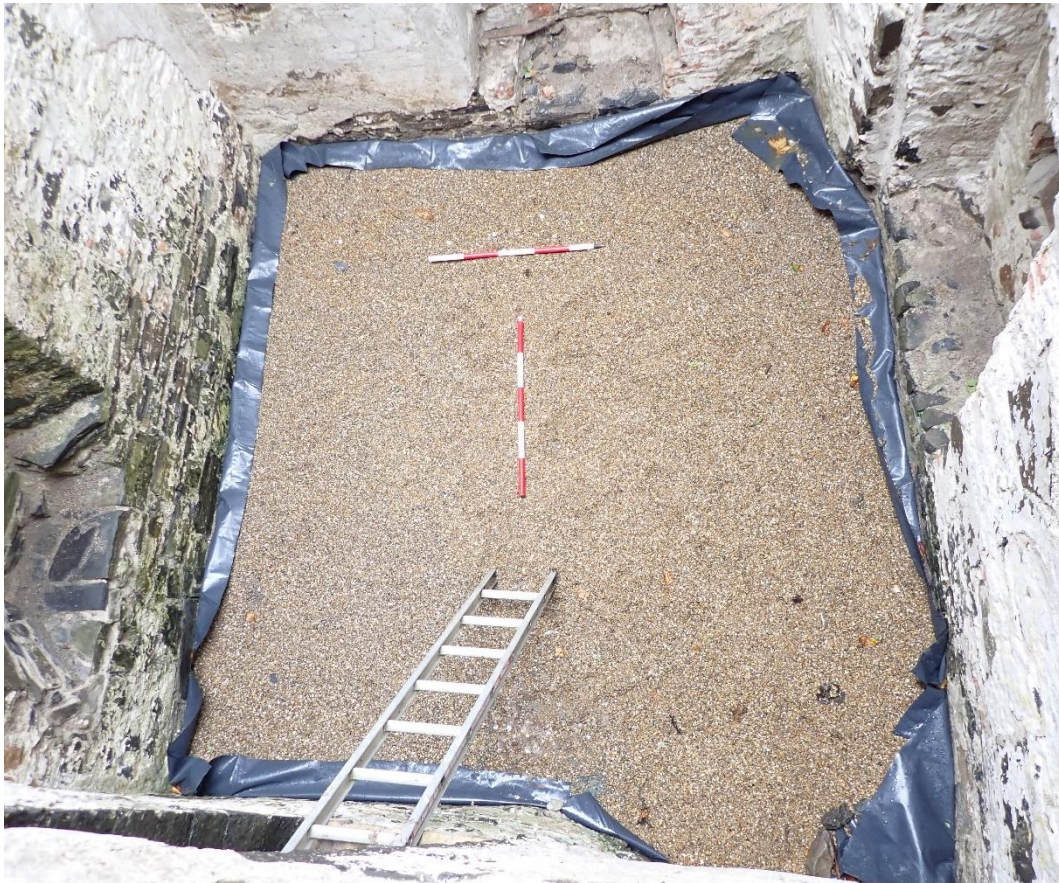
Plate 8: Impermeable membrane with gravel covering it laid over the sand, from west
