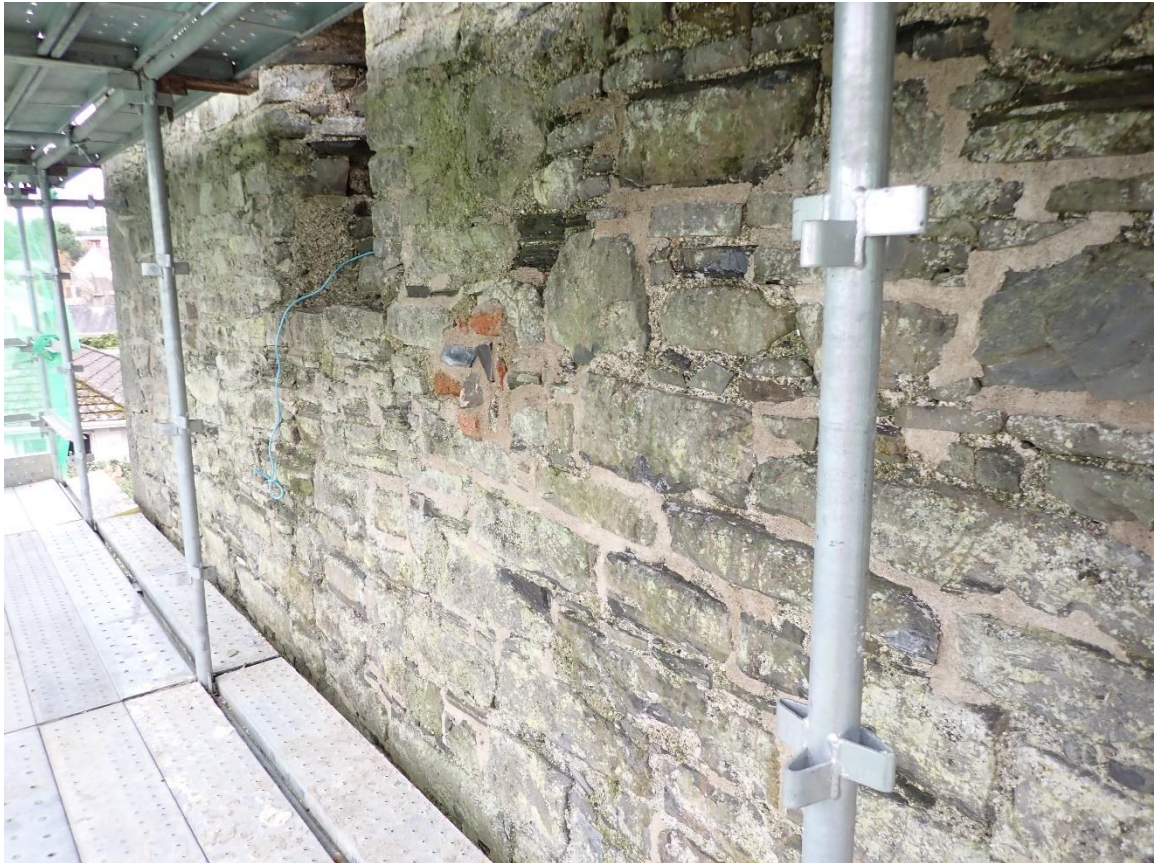
Plate 12: North wall, first floor above vault after re-pointing
