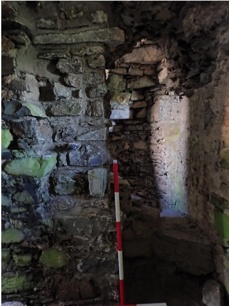
Plate 10: Re-built section of unsupported masonry where a gap was broken into the second floor room, west side, from the stairs
