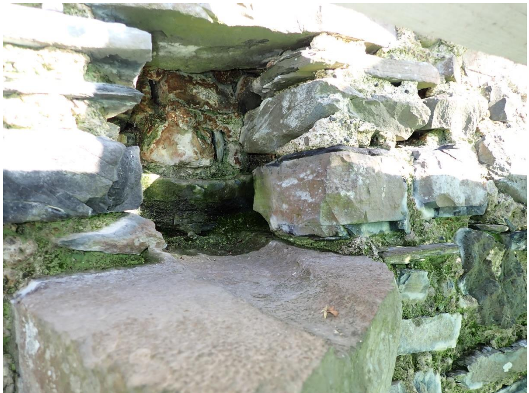
Plate 17: Blocked spout on south side, west wall
