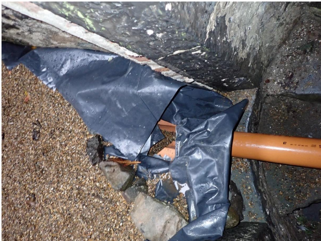
Plate 9: part of drainage system leading out over the step and ultimately draining out a window in the west wall
