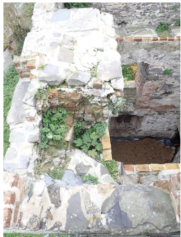
Plate 20: JK inspecting the north wall where the vertical crack was stitched and re-pointed
