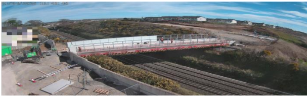
Bridge showing some Kalwall parapet panels being installed
