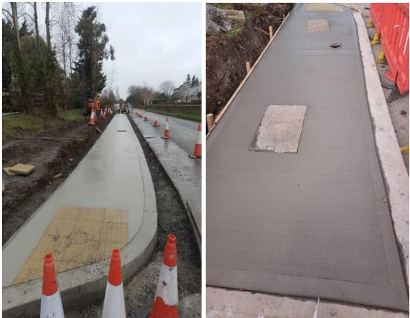
Installation of new footpath along Kinsealy Lane.
