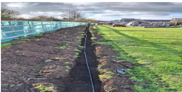
New water pipes for additional water taps around cemetery. Fingal Burial Grounds works carried out by outdoor staff.
