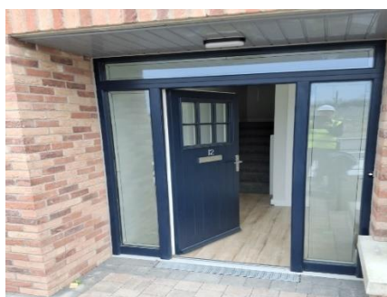
Checking level access and drainage detail to a threshold of a house in Oldtown.
