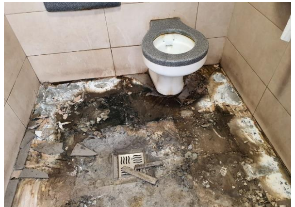
Following damage - removal of broken tiles Howth toilets in preparation for new replacements.
