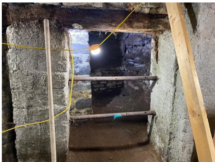
Plate 21: Timber lintel in place
