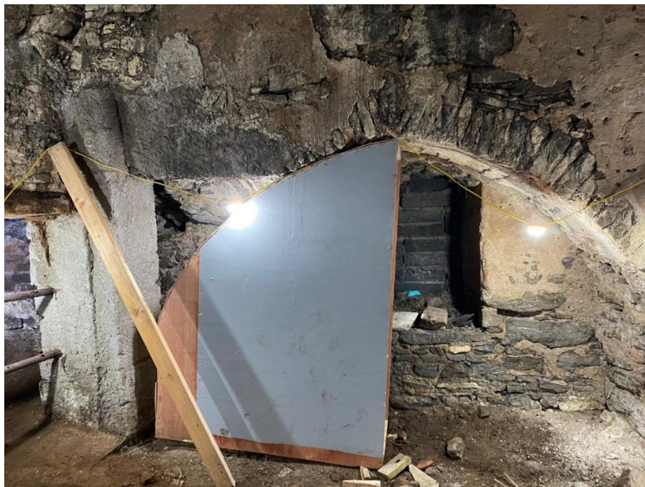
Plate 19: Ground Falsework inserted during reconstruction of ground floor arch, facing west
