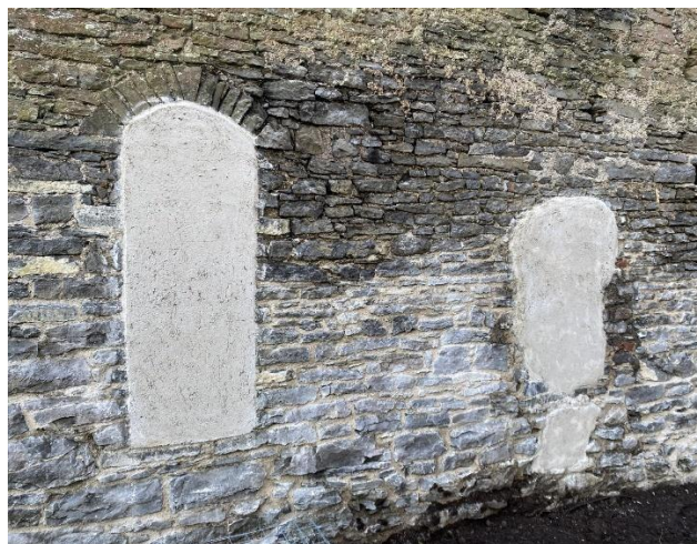
Plate 34: Lime render over blockwork infill of opes in western gable
