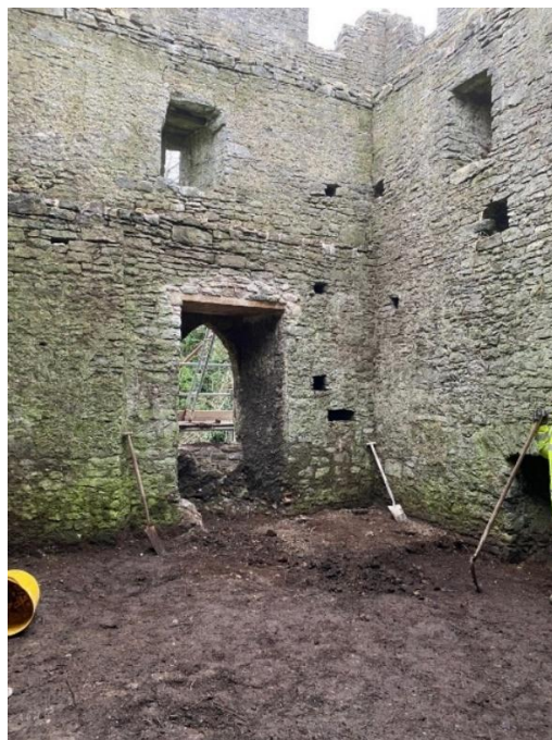
Plate 11: Hand removal of soil overlying vault, with replaced western lintel visible, facing west
