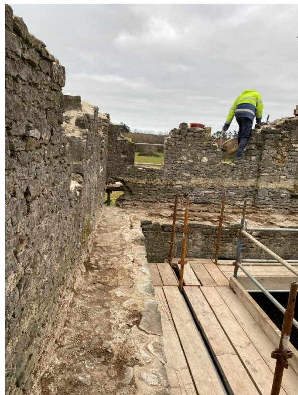
Plate 25: Western wall walk following removal of brick
