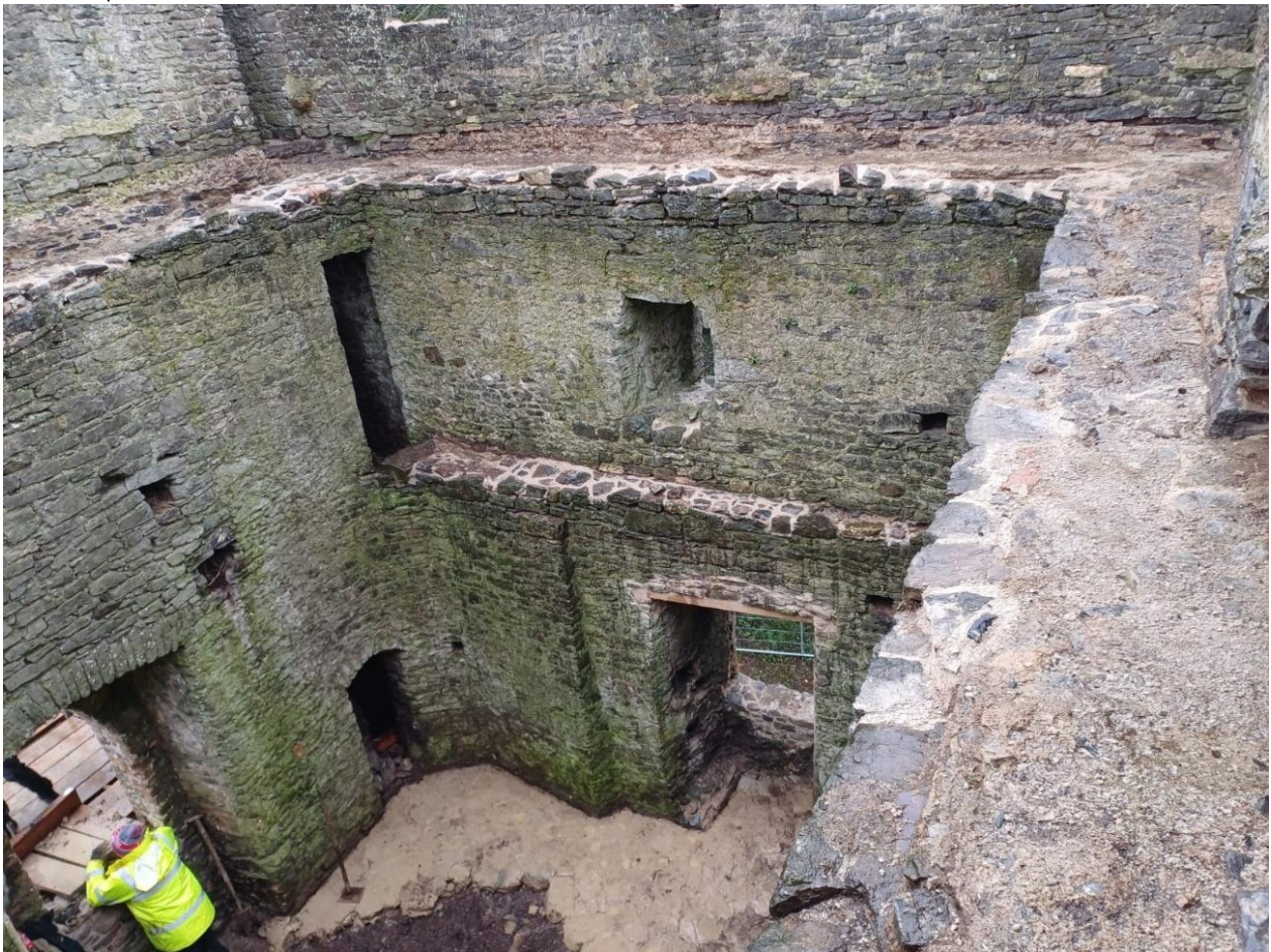
Plate 27: Rough racking on wall walks, facing southwest
