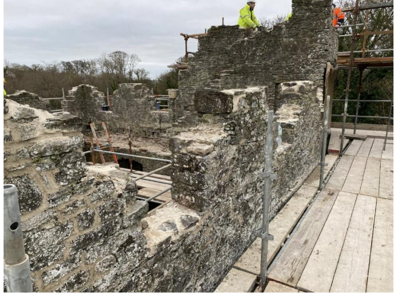
Plate 26: Flaunching on eastern wall top
