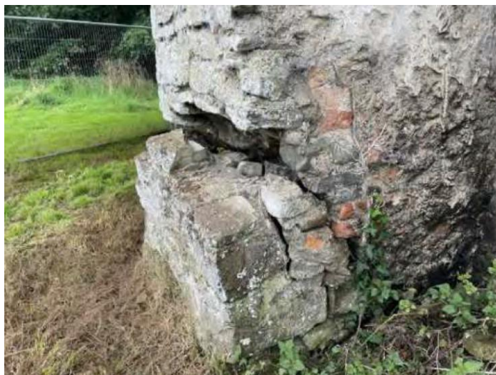
Plate 2: Subsidence in southeast corner wall, facing south
