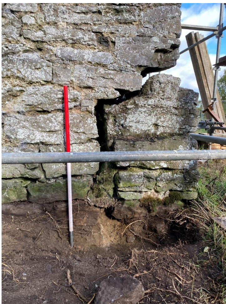
Plate 2: Subsidence in southeast corner wall, facing south
