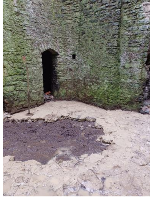
Plate 15: Installation of puddle clay art first floor level, facing northeast
