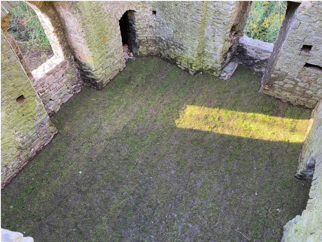
Plate 16: Grassed sod installed over puddle clay at first floor level
