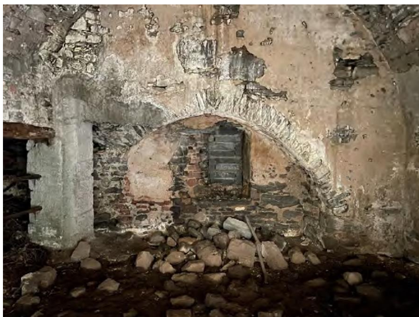
Plate 17: Ground floor interior showing compromised arch, hoof-pocked muck and loose stone, facing north
