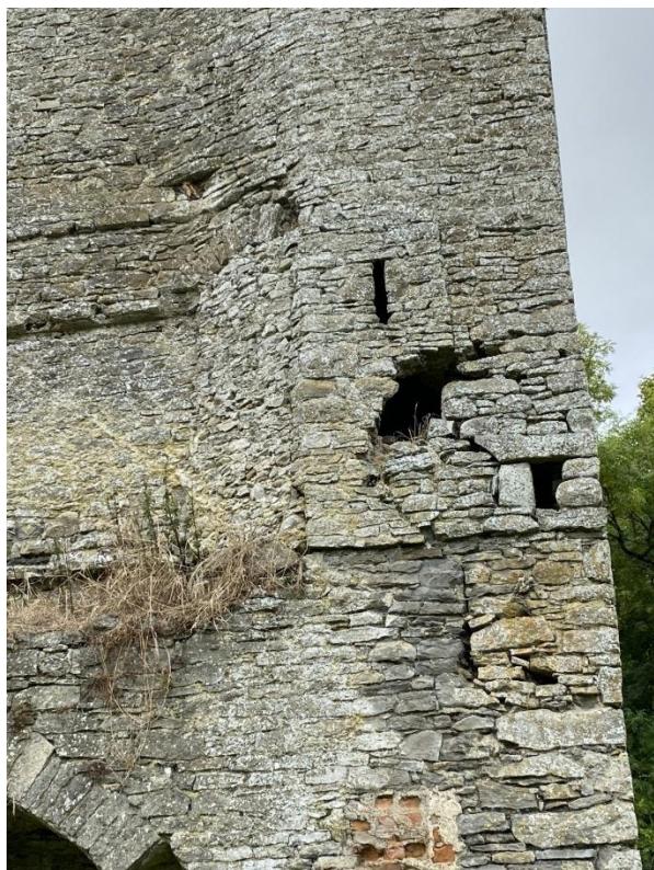
Plate 31: Gap in the masonry at the northeast stairwell, facing west
