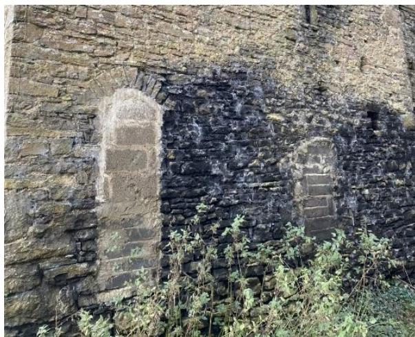
Plate 33: Blockwork infill of opes in western gable
