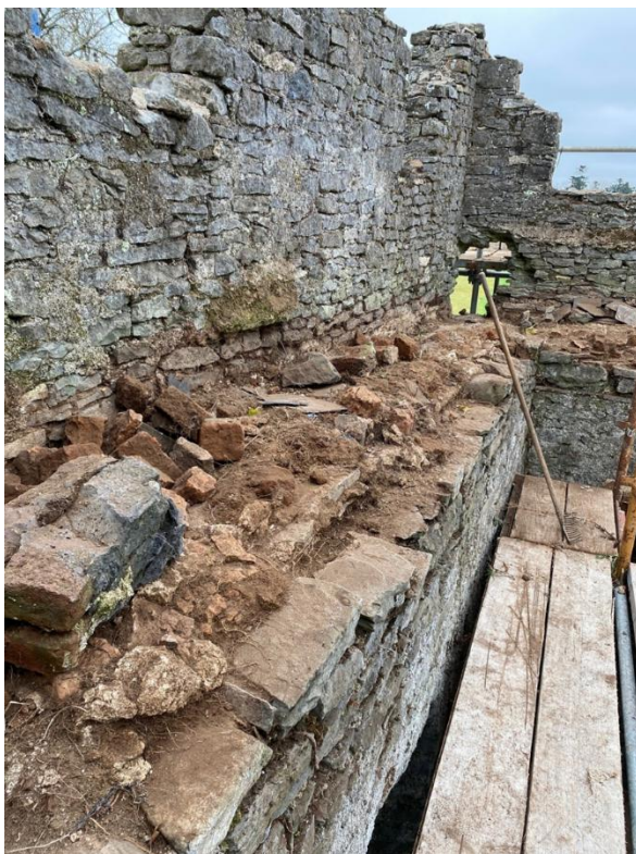
Plate 24: Loose brick on western wall walk
