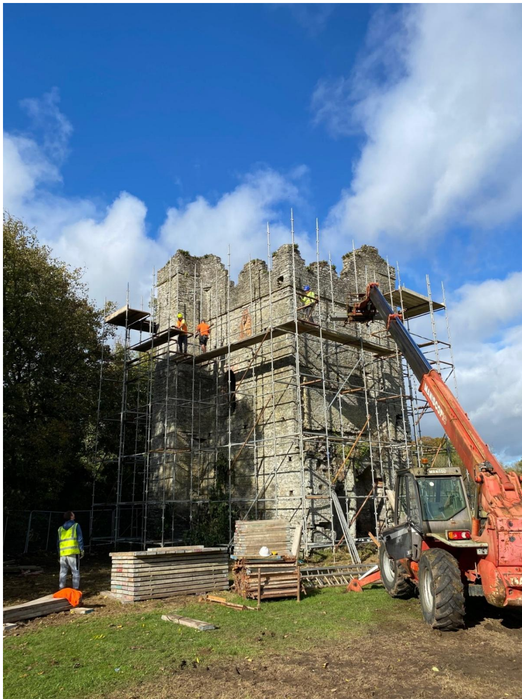
Plate 1: Erection of scaffolding prior to conservation works
