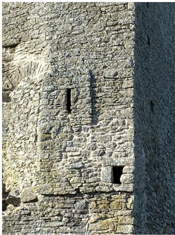
Plate 32: Repaired masonry at the northeast stairwell, facing west
