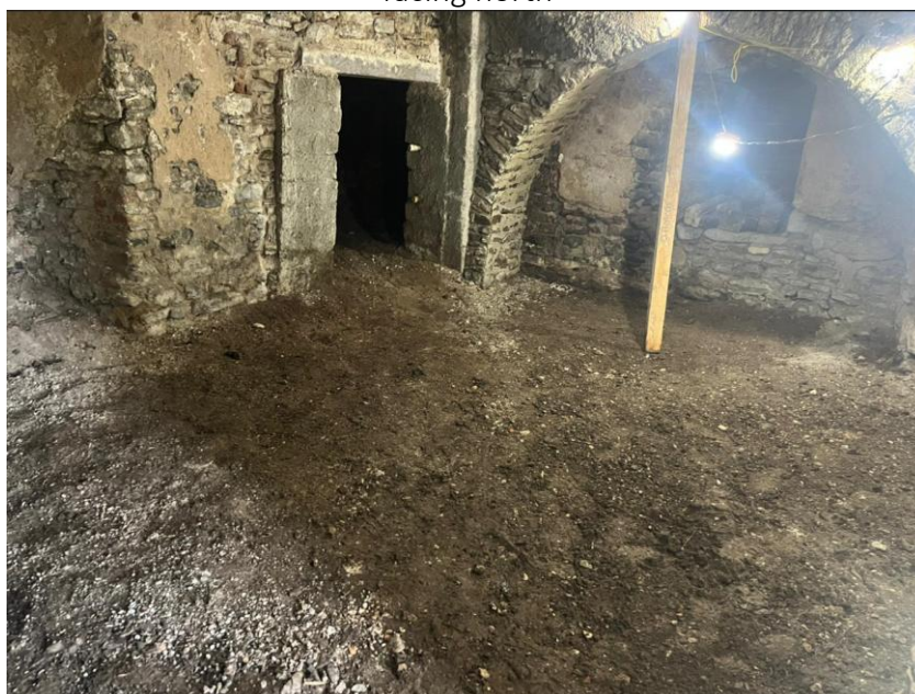
Plate 18: Ground floor interior following reconstruction of arch and removal of muck and stone
