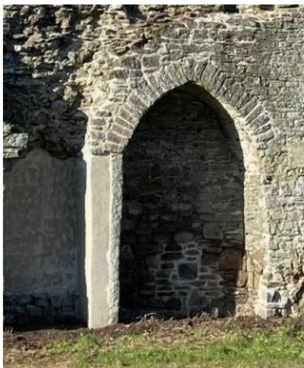
Plate 9: Lime mortar harling and repair to arch, facing west
