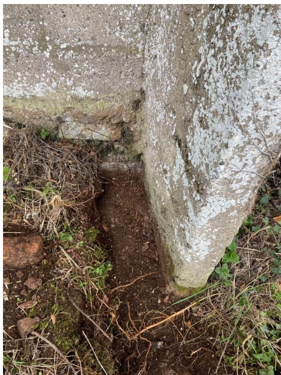
Plate 8: Base of single-leaf wall
