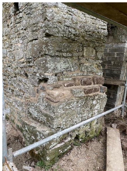
Plate 5: Lime mortar repair to projection, facing northwest
