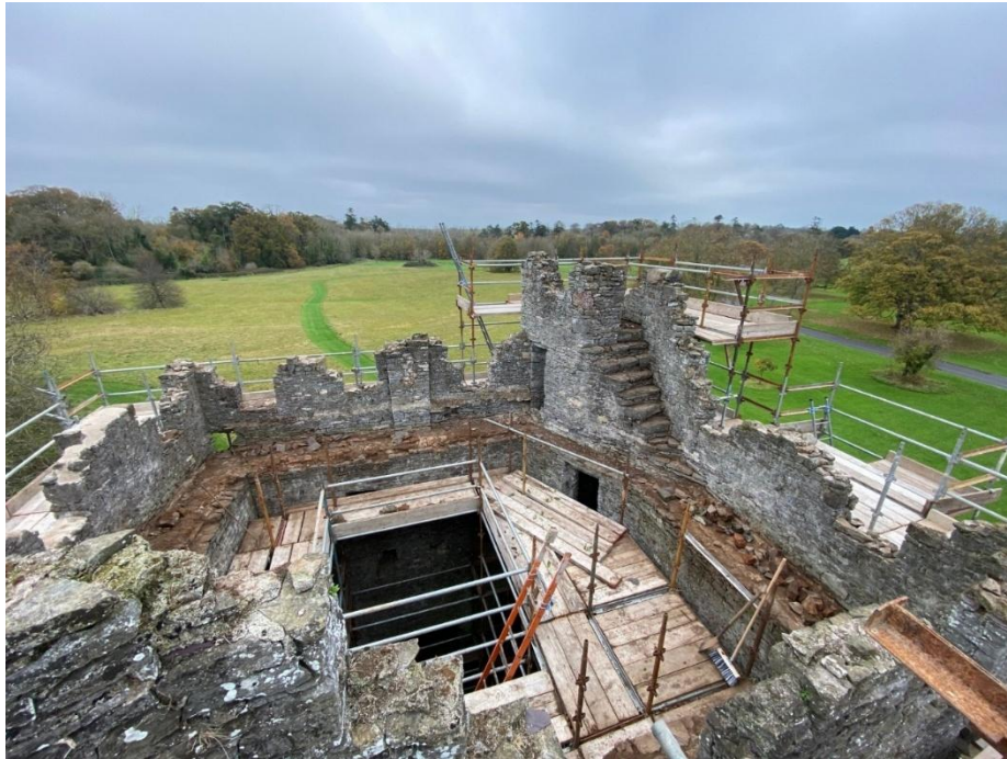
Plate 23: Upper levels showing loose redbrick on wall walks
