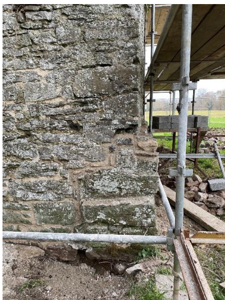
Plate 4: Lime mortar repair to projection, facing north
