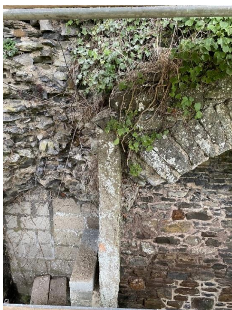
Plate 6: Single-leaf wall supporting compromised arch, facing west
