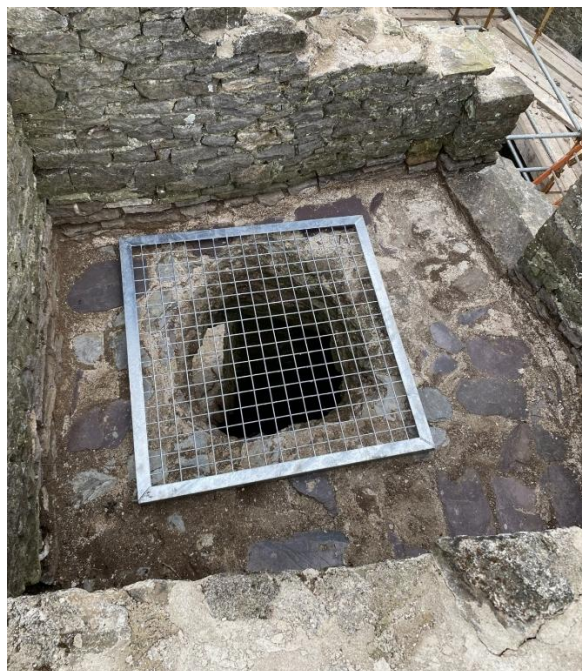
Plate 28: Metal grille over improvised 18th century chimney. Facing north
