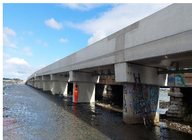
Bridge in place and painting of bridge piers ongoing
