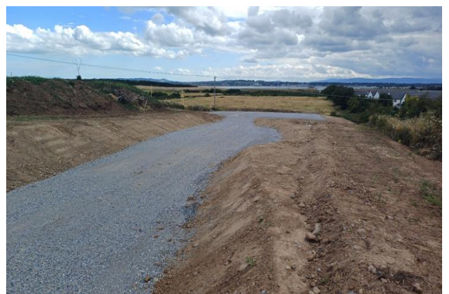
Photograph of haul road for construction vehicles to access the site from the eastern side of the railway.
