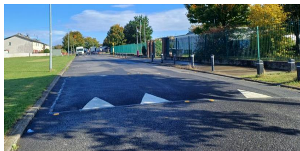
St. Margarets – Rivermeade Drive – New Traffic Calming Ramps
