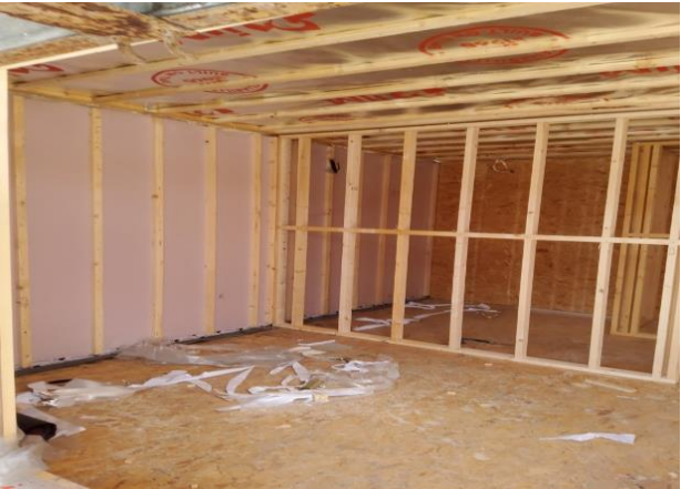
Stud walls being assembled in a timber frame house in Rush.
