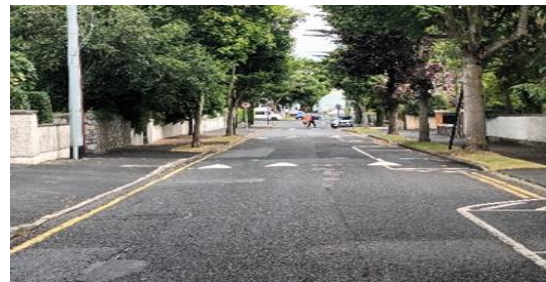
New Traffic calming scheme for Grove Road Malahide with 5 new ramps installed.
