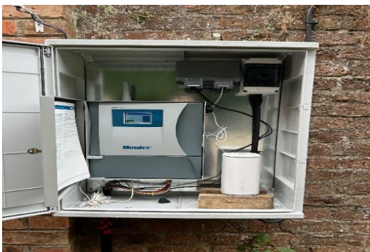
Hunter control panel with Wi-Fi for new irrigation system.
