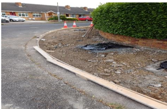
Operations roads crew are currently replacing defective footpaths in Binn Eadair View Sutton.
