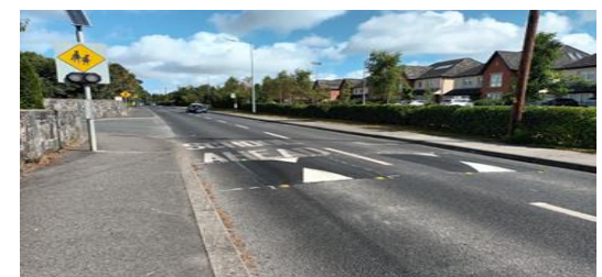
Additional traffic calming on the R124 approaching Malahide Community School. Two new speed cushions provided.
