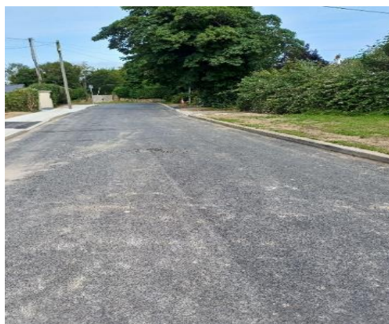
Operations Roads Crews laid ducting and replaced the defective concrete and tar footpaths on Grey's Lane to bring it up to taken in charge standard. This was a historical estate not taken in charge. It was overlaid in early 2024.
