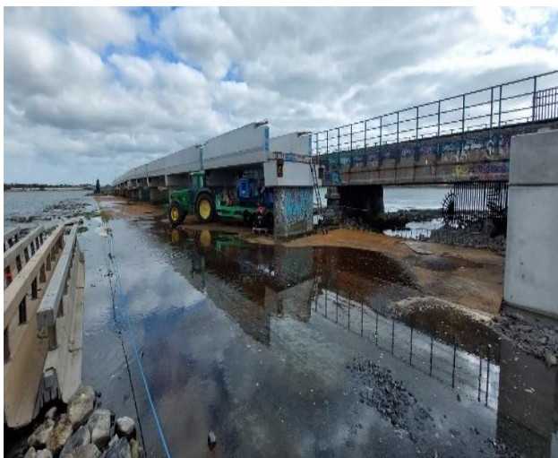
Precast units in position to form the Broadmeadow Bridge - 16 th August.
