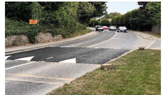
Additional Traffic Calming Construction on the Drumnigh Road (3 Bus Ramps and 1 set of cushions)
