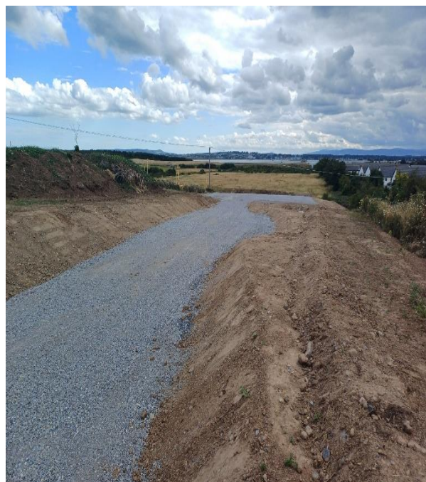
Photograph of haul road for construction vehicles to access the site from the eastern side of the railway.
