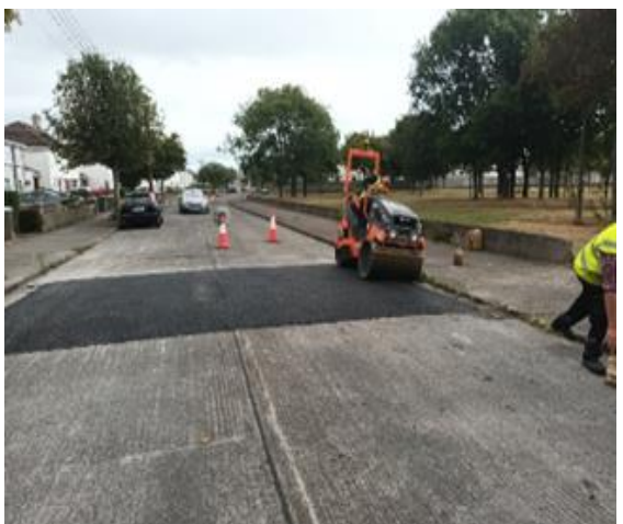
New Traffic calming scheme for Alden Road with 6 new ramps provided.
