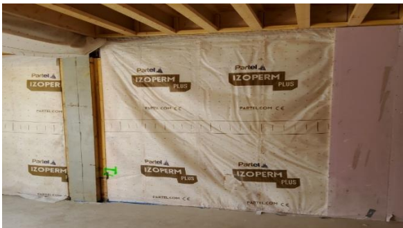
Checking air tightness membrane and fire proof plasterboard at a house in Castleknock.
