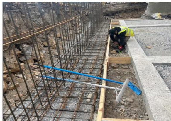
Foundation and retaining wall construction works being carried out at Howth East Pier above
