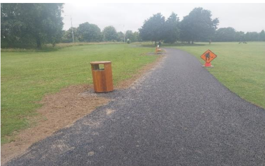
Approx 1 Km of Footpath widening and over lapping at Tir-Na-Nogg Park in Carpenterstown
