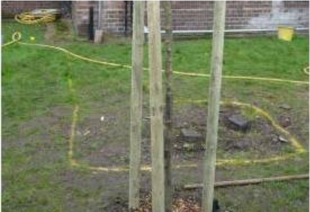
Image: recently planted tree and rain garden redesigned around the underground services
