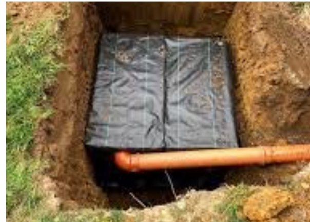
Image: soakaway being installed
