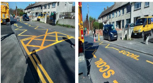
St. Teresas Catholic Primary School Balbriggan. Installation of 'School' keep clear markings, school warden crossing markings and double yellow lines.
