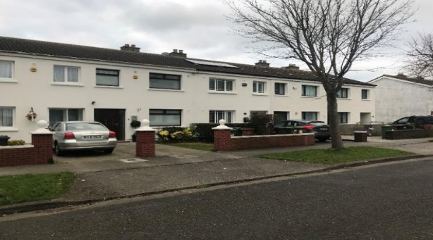
Post-works – Strandmill Estate, Portmarnock (external wall insulation, new windows and doors)
