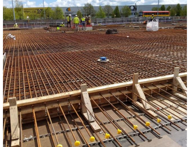
Inspecting steelwork in a ground floor slab of an apartment block in Charlestown.
