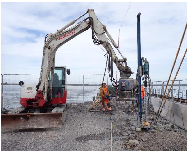
OHLE Mast Strengthening Works – Southern Access Haul Road – Broadmeadow Estuary
