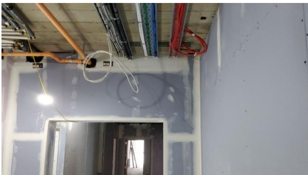
Inspecting fire stopping above a doorway in a compartment corridor in Santry.
