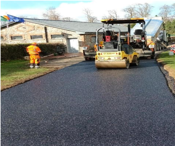
New overlay carried out outside the pavillion road.
