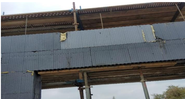
Inspecting ICF (Insulated Concrete Formwork) on a site in Rowlestown.
