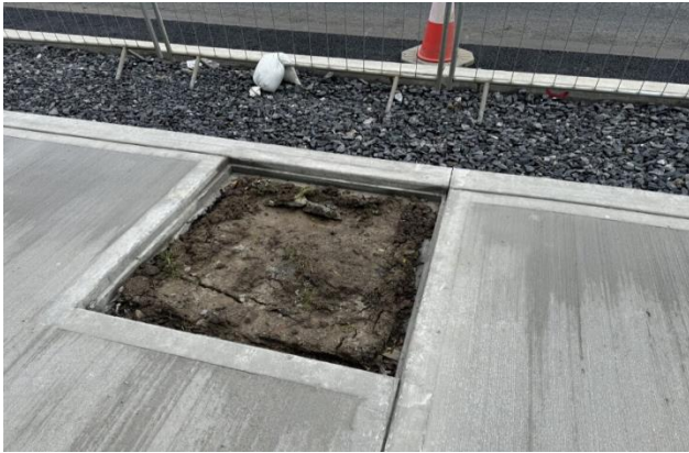
Works progressing on Harry Reynolds Road just South of Fingal Bay Business Park with Tree Pits installed.
