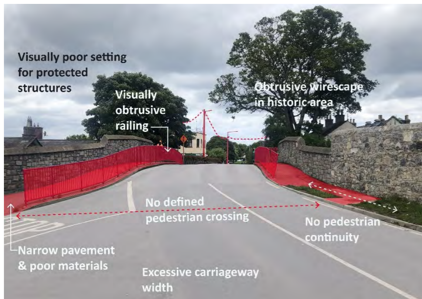
Fig. 7-6: Current View of the Bridge
