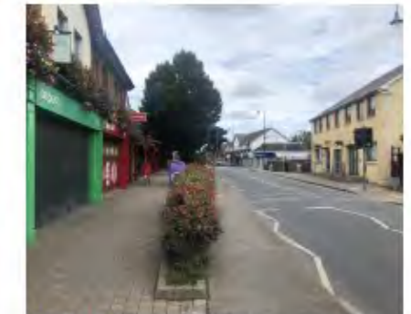
Poor positioned planting
