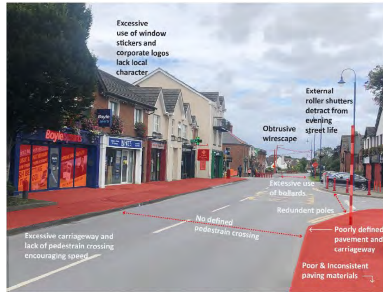
View of Main Street—Illustrates uncoordinated streetscape, excessive carriageway width and extensive black surface, poor quality footpaths, poor pedestrian continuity, and unplanned verges and planting create an overall discordant streetscape that lacks distinctiveness and creates a poor sense of place and identity, exemplified in this section of Main Street.
