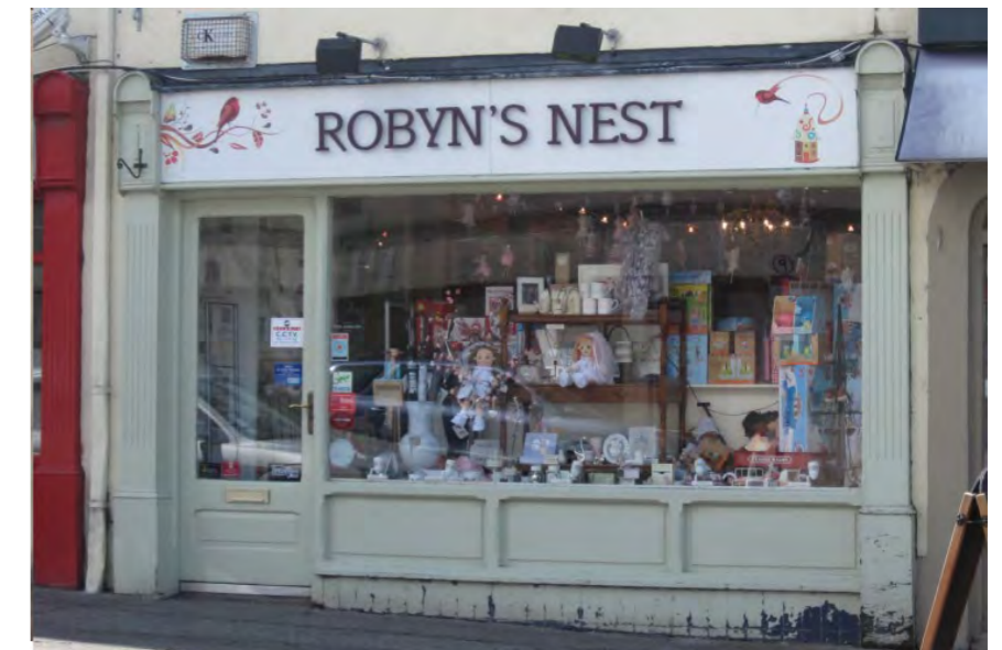
Fig. 9-17: Example of Appropriate Shopfront Design
