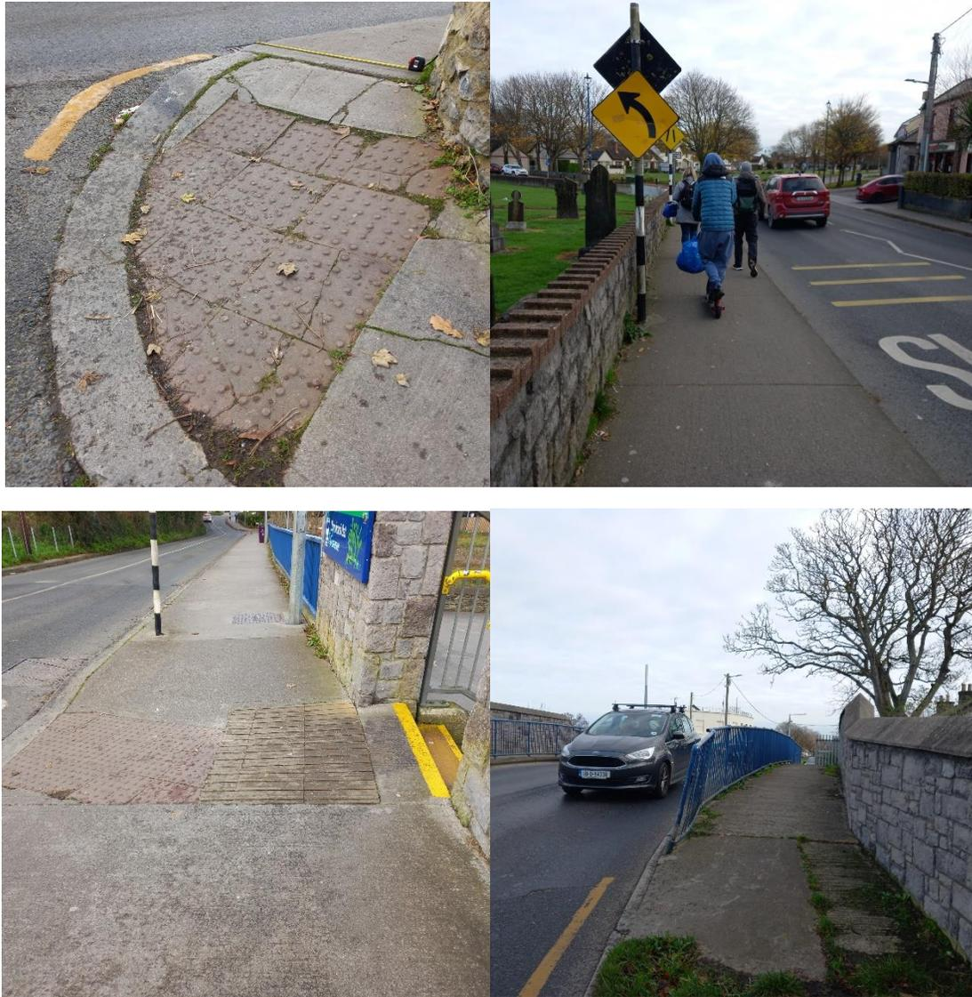
Incorrect use of tactile paving which is badly maintained, can lead to trips and falls.
