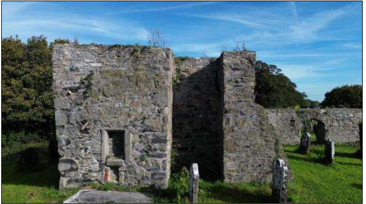
Plate 10 View of southern elevation of tower, facing north
