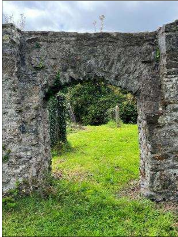
Plate 8 View of doorway, facing south
