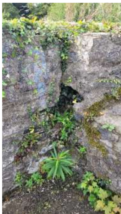
Southwest internal corner above vault.
