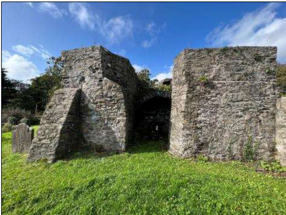
Plate 9 View of western gable end of church, internally
