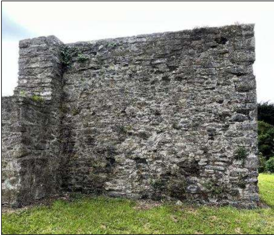
Plate 14 Northern elevation of residential tower, facing south
