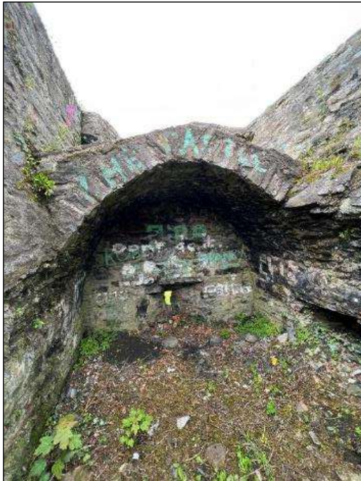
Plate 15 View of nave/ground level of tower, facing west
