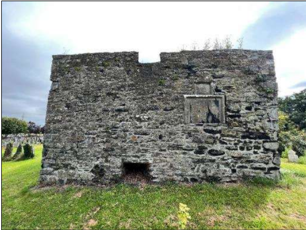
Plate 12 Western elevation of residential tower, facing east
