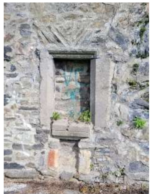
Window south elevation of Tower.
