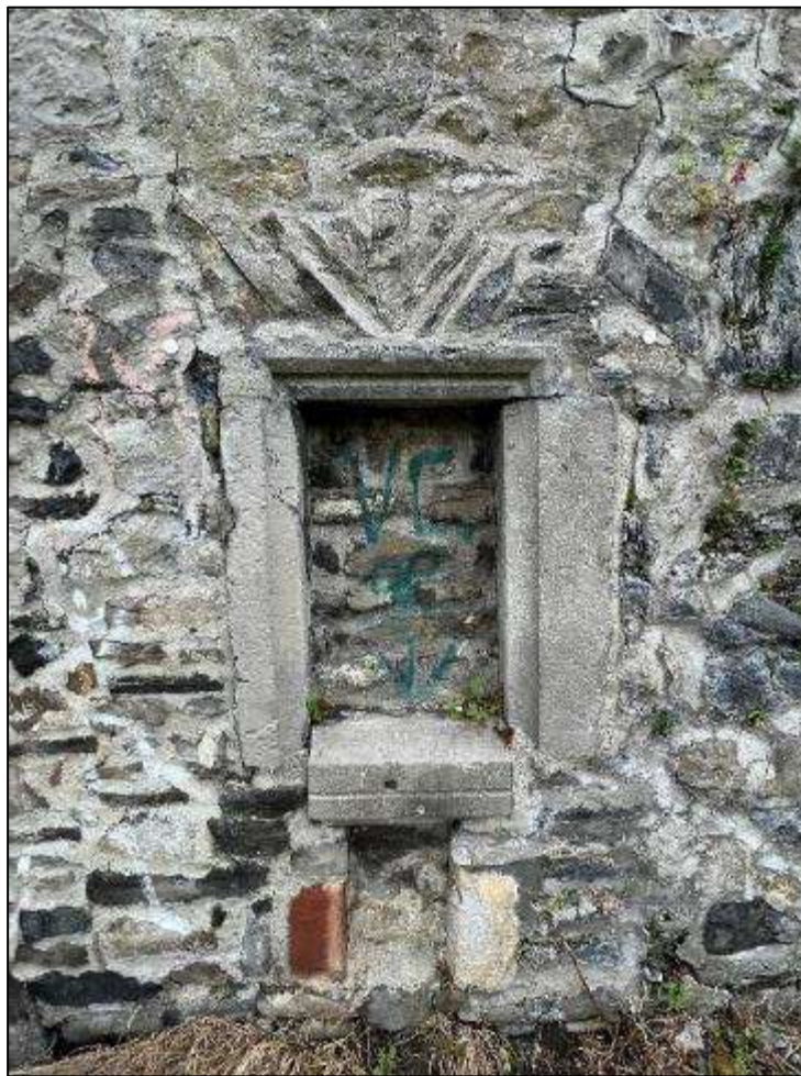
Plate 11 Blocked window opening on southern elevation, facing north
