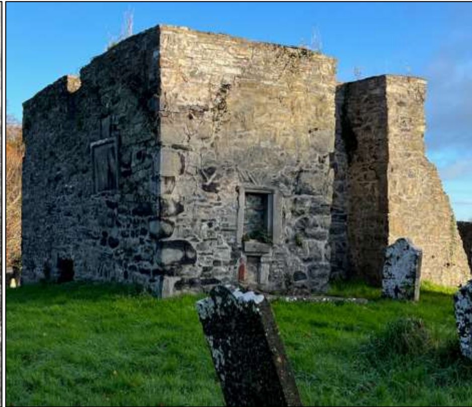
Plate 16 View of tower from northwest, present day
