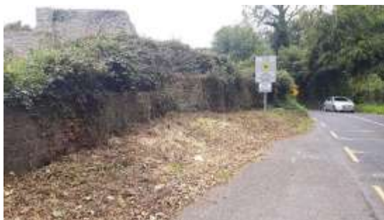
West wall, partially cleared Autumn 2023. Note poor sightlines to south.
