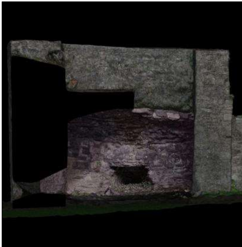
Plate 20 West to East section through tower, showing massing (Archer Heritage Planning)
