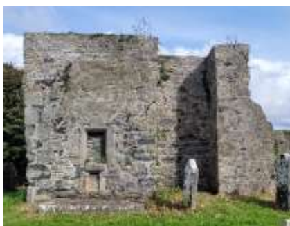
South elevation of Tower.
