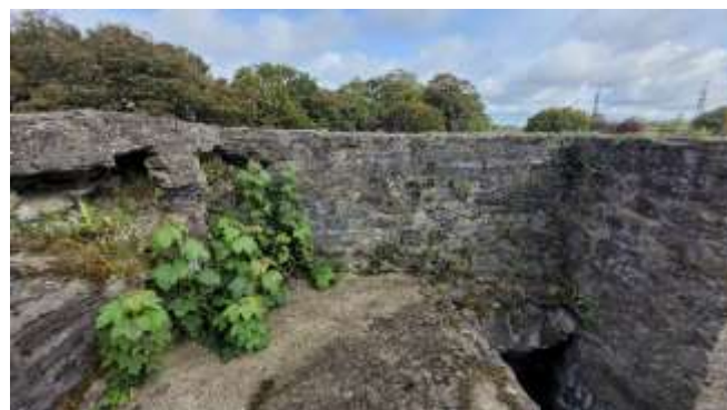
Tower vault top looking north.
