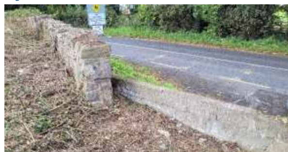
West wall contains a mix of stone and block.
