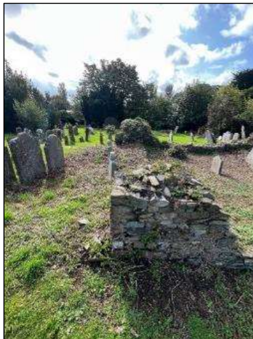
Plate 7 East wall of church, facing south
