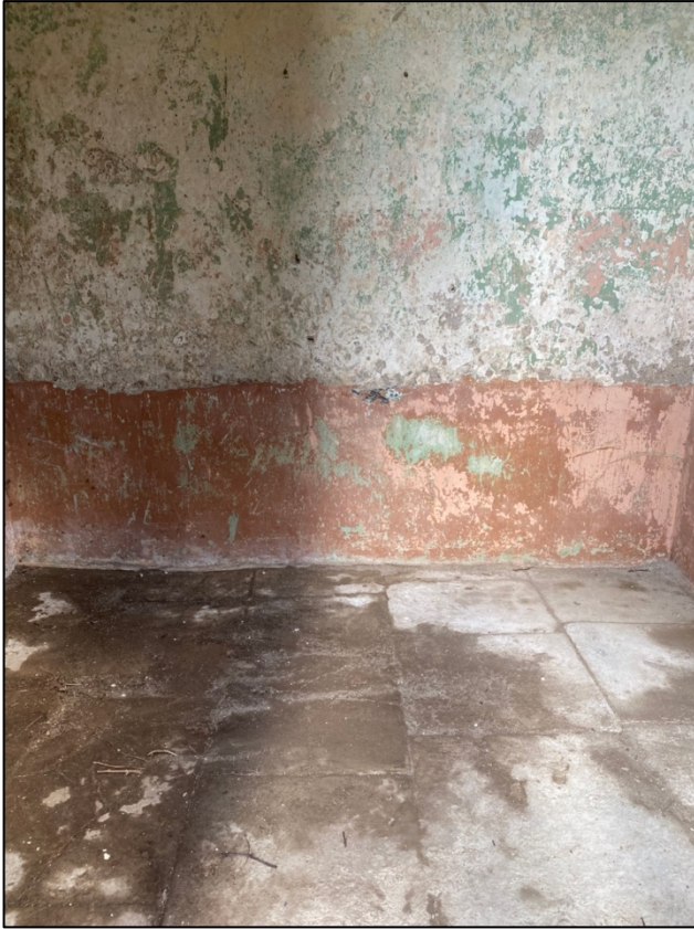
Plate 31: Detail of cleared floor slabs in bell tower, facing north-northeast.
