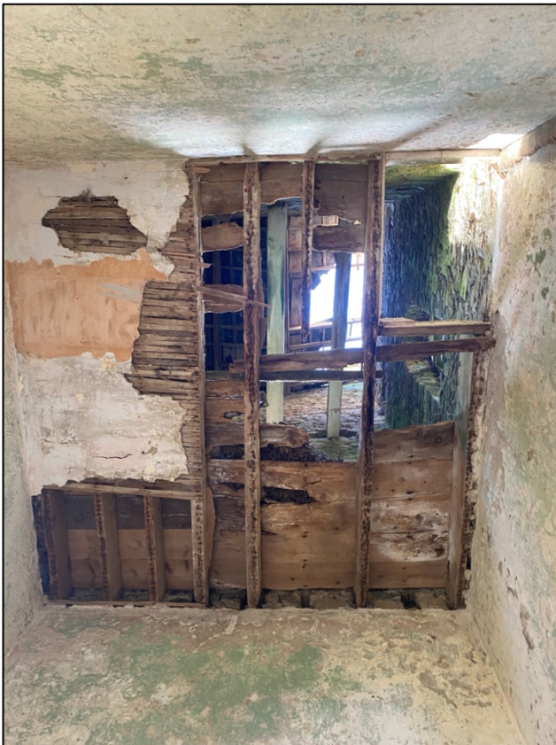
Plate 22: Extant timber sections in ringing platform of bell tower.
