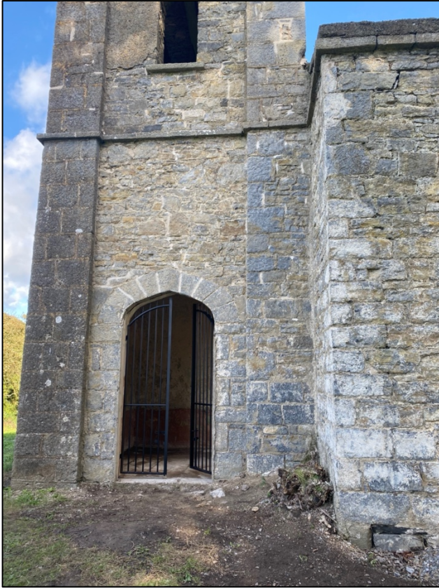
Plate 29: Newly fabricated and fitted gate to bell tower, facing north-northeast.
