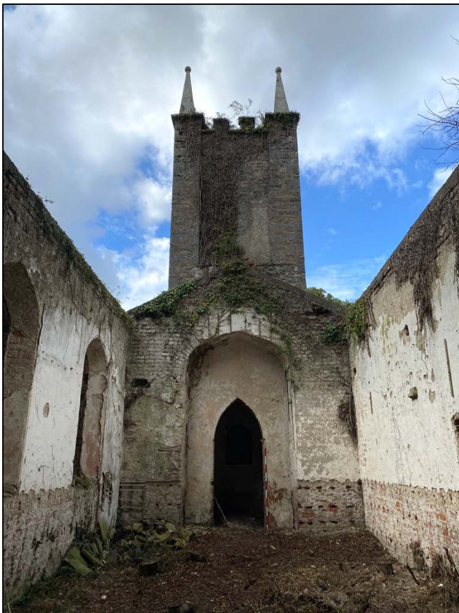
Plate 2: Interior of church with nave and bell tower, facing west-northwest.
