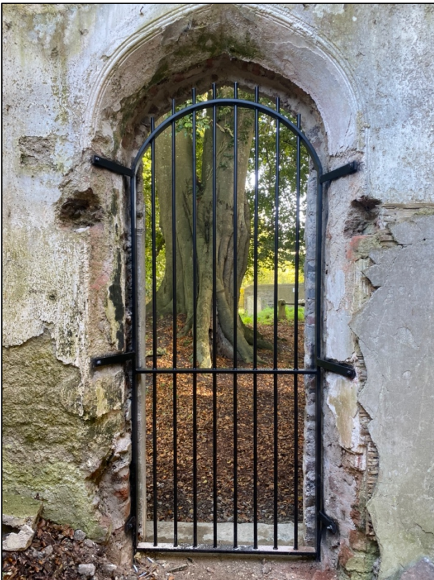
Plate 28: Newly fabricated and fitted gate to vestry, facing east-southeast.
