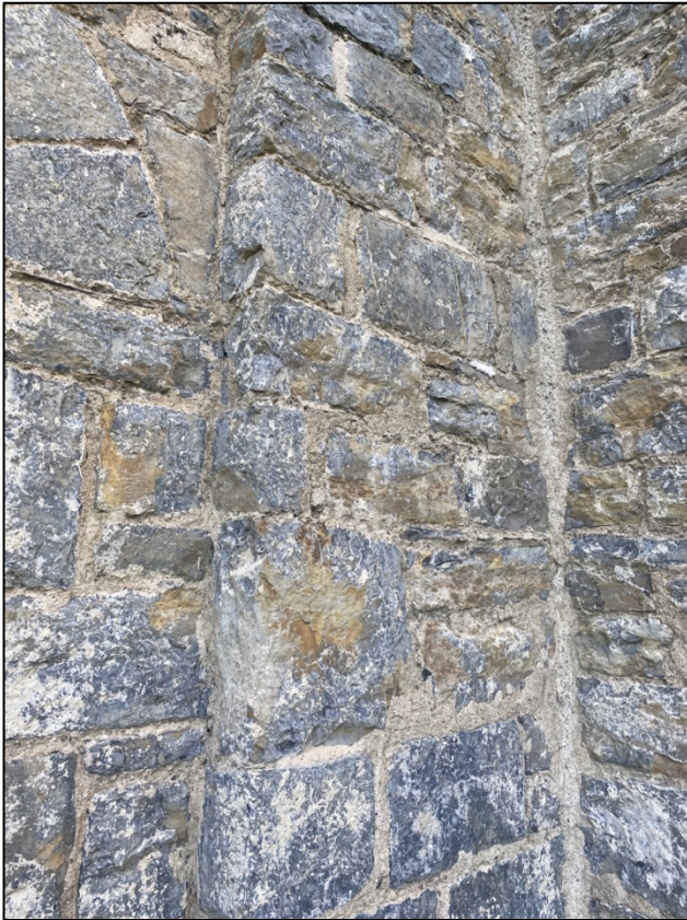
Plate 34: Detail of repointing on south elevation of bell tower, facing northeast.
