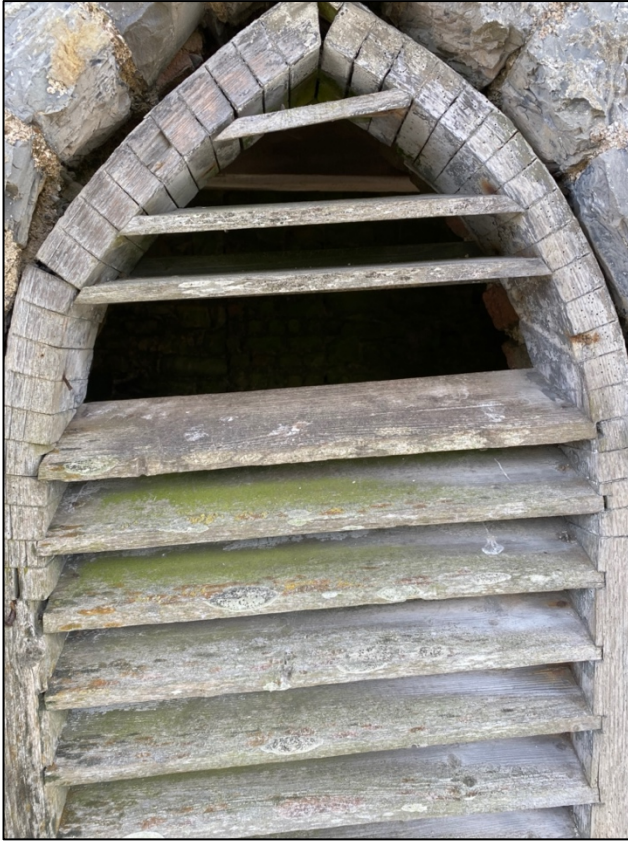
Plate 23: Timber louvres within timber frame in west elevation of bell tower.
