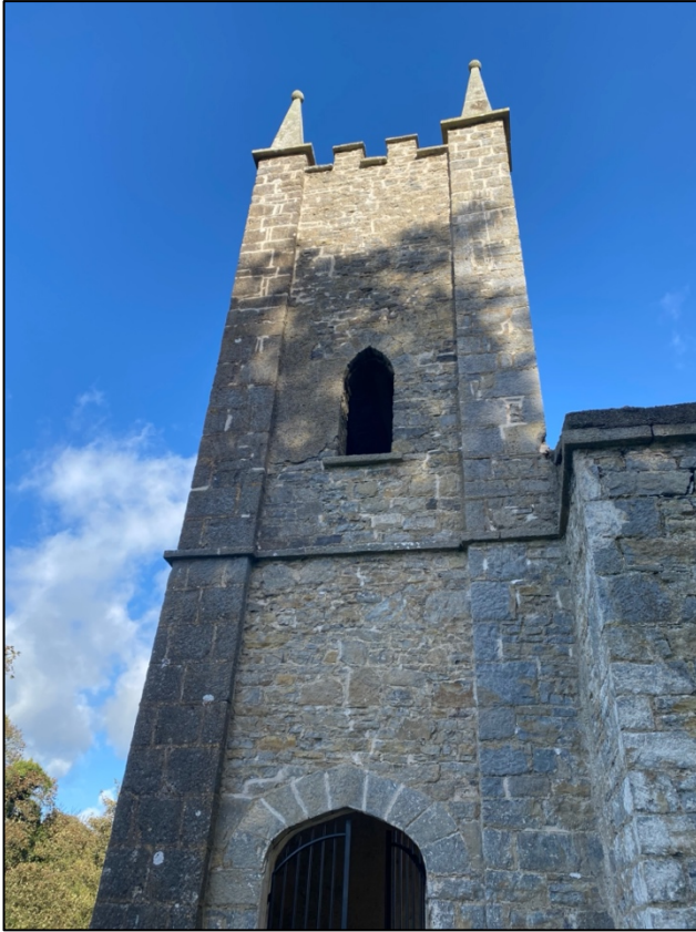
Plate 33: Repointing on south elevation of bell tower, facing north-northeast.
