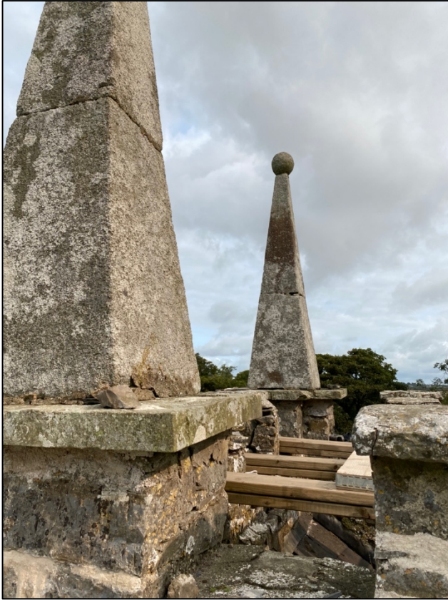
Plate 19: Detail of stone pinnacles in bell tower.
