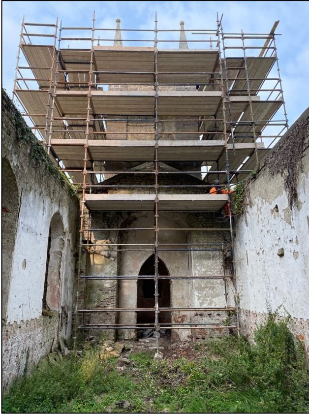
Plate 21: View of scaffold on bell tower from nave, facing west.
