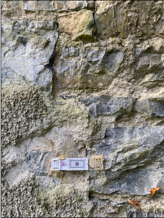
Plate 35: Tell-tale on exterior east elevation of nave, west northwest.
