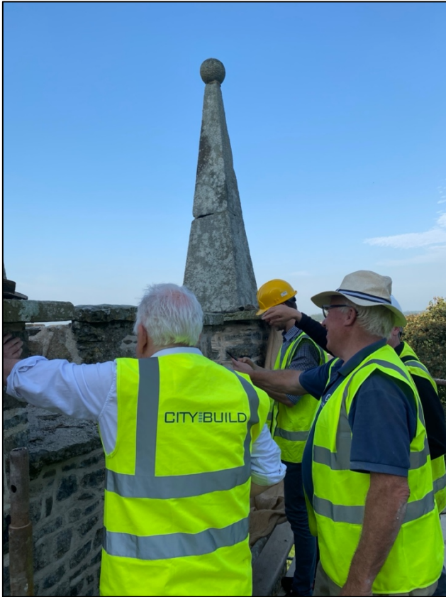
Plate 27: Inspecting pinnacles, stone cappings and crenellations during the NMS site visit.
