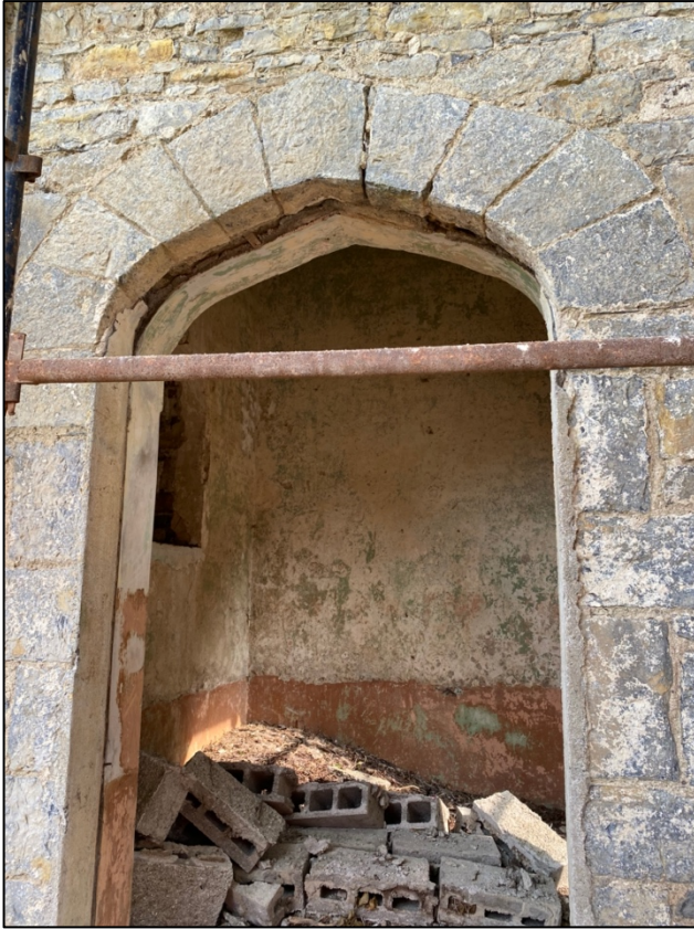
Plate 25: Entrance to bell tower following removal of modern blocks, facing north.
