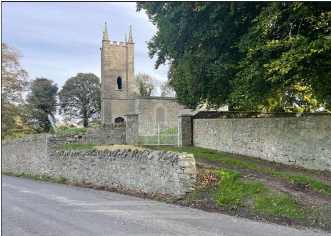
Plate 10: View of entrance to site following removal of welfare facilities and signage, facing north-northeast.
