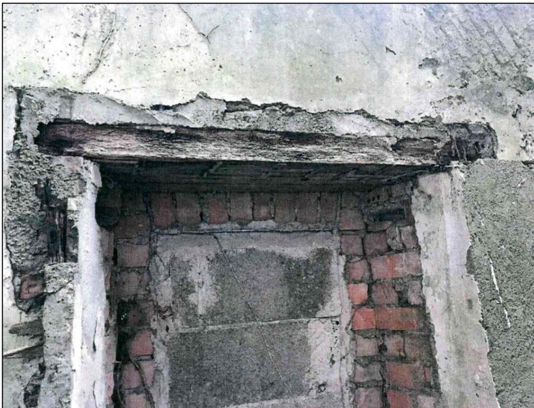
Plate 16: Timber lintel above window on west wall of vestry.
