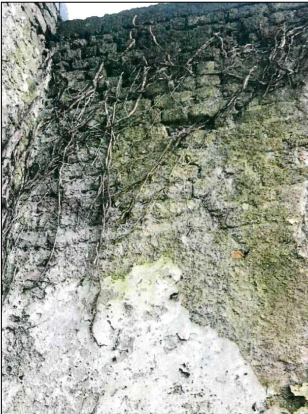
Plate 18: Diagonal cracking in brickwork at south internal elevation.
