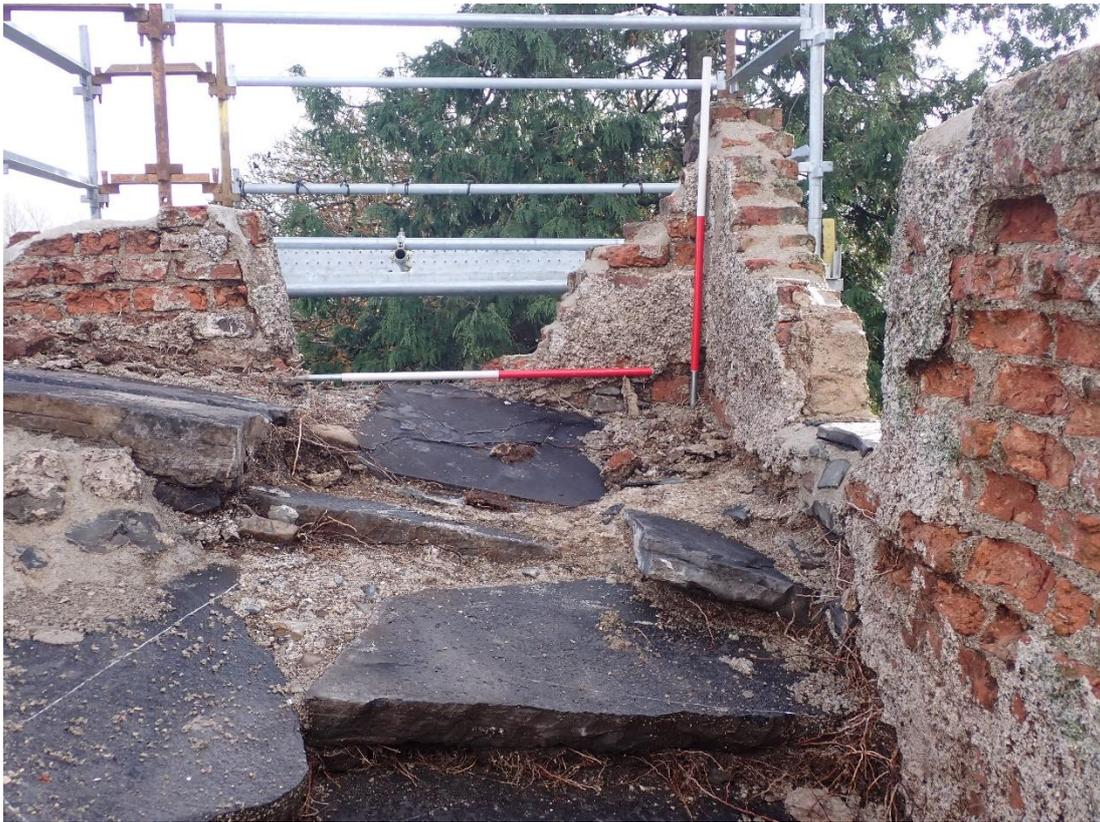
Plate 3: View to south of roof showing flagstones sloping from east to west and from south to north
