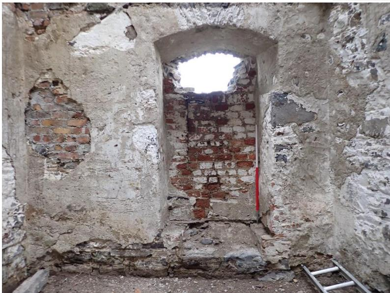
Plate 29: First floor window opening, east wall. Repair to brick to left.
