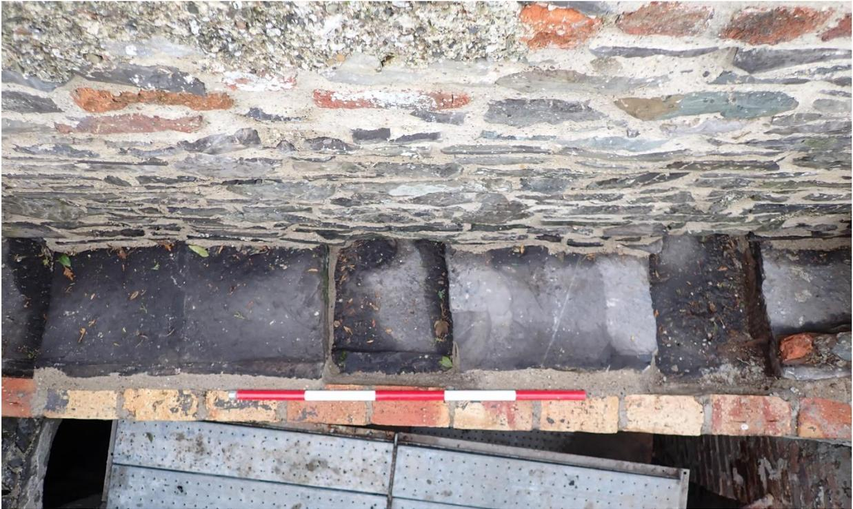
Plate 12: Wall walk on the north side during conservation. The ranging rod sits on replaced brick.
