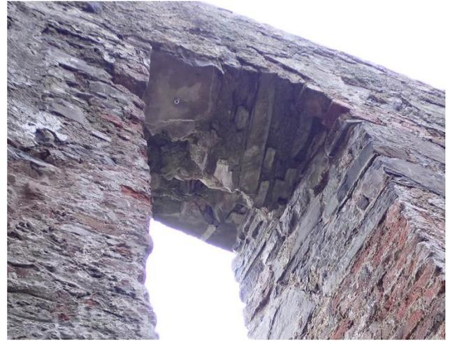
Plate 19: The screw threaded through the unsupported masonry beside the end of the arch
