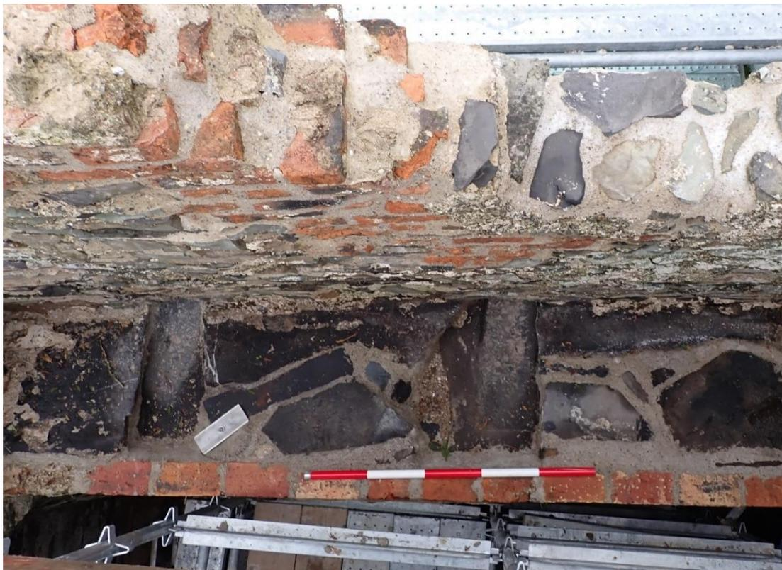
Plate 20: The plate and head of the threaded bar pinning the masonry beside the window arch on the south wall walk
