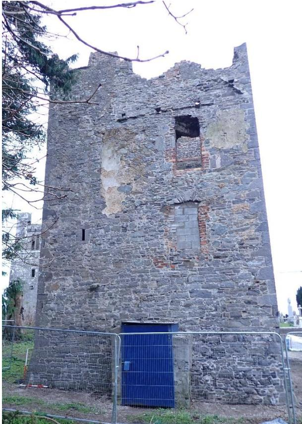
Plate 16: South wall after conservation. Note roof scar and conserved plaster.
