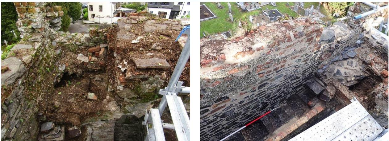
Plate 10: Slate line in NE corner, before and after conservation
