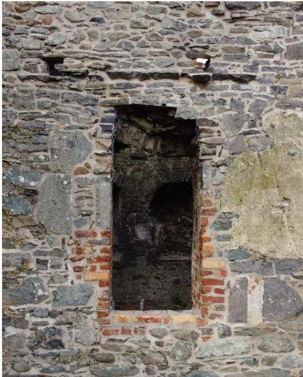
Plate 18: The repointed opening with infilled stonework; the newly revealed window loop is at bottom right
