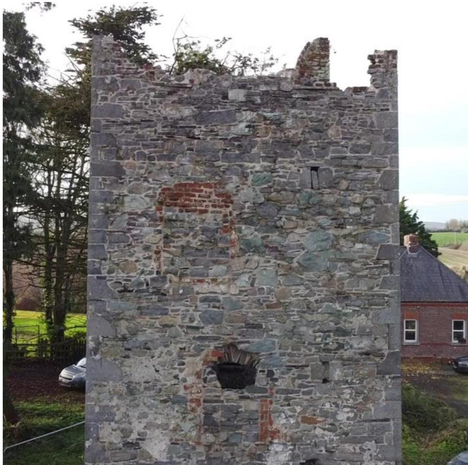
Plate 22: View of the mid-section of the east wall showing the arrow loops, and consolidated brickwork
