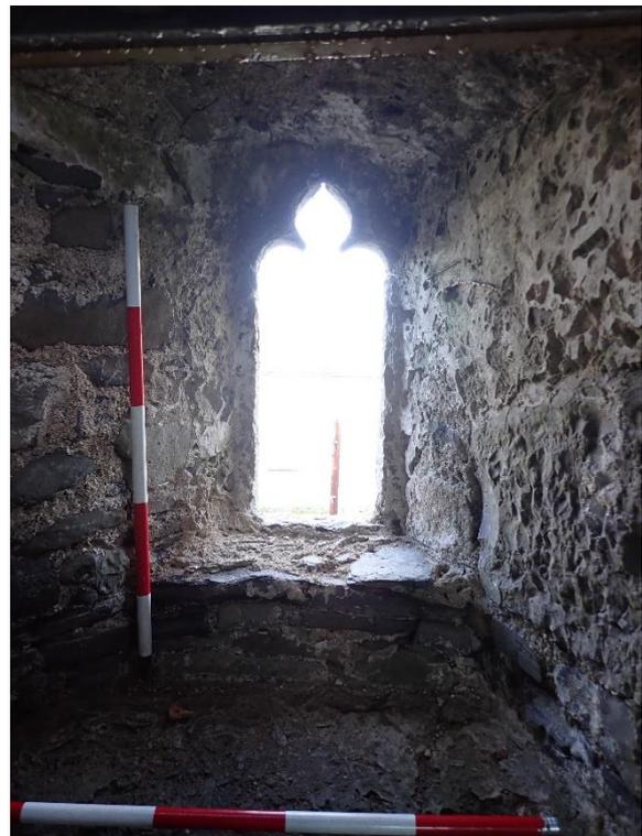
Plate 25-26: Window reveal repaired, first floor level and window area cleaned second floor level, north wall
