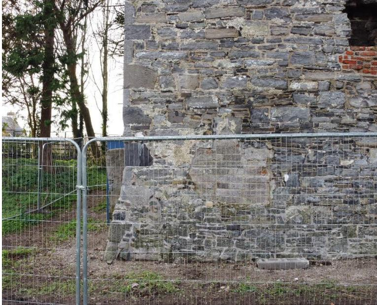
Plate 21: View looking west at the SE corner which has been repaired and consolidated.
