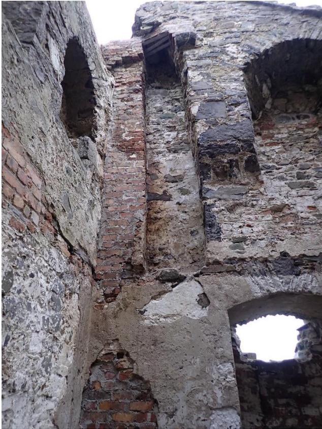
Plate 27: looking upwards along the north side of the east wall, chimney flue repaired and stitched with bar through the cavity
