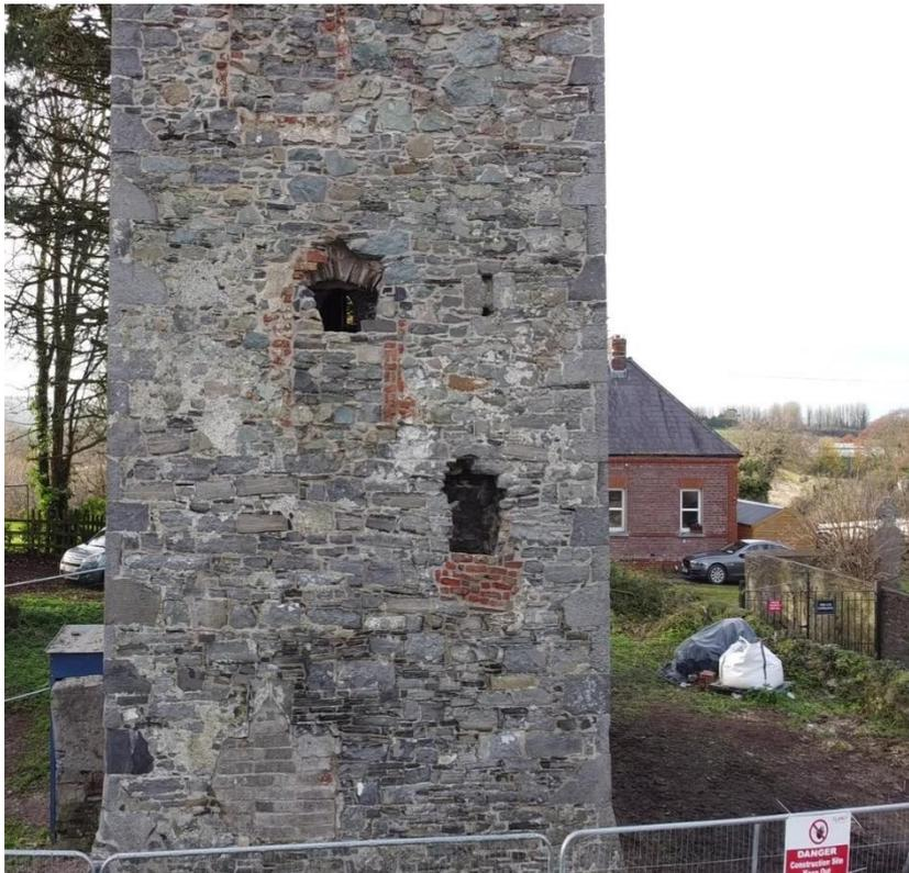
Plate 23: Lower section of the east wall exterior showing cleaning and repairs
