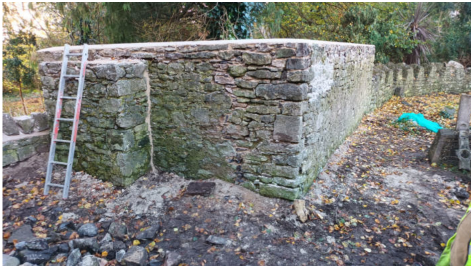
Plate 11: View of re-pointed building at south of boundary wall from east
