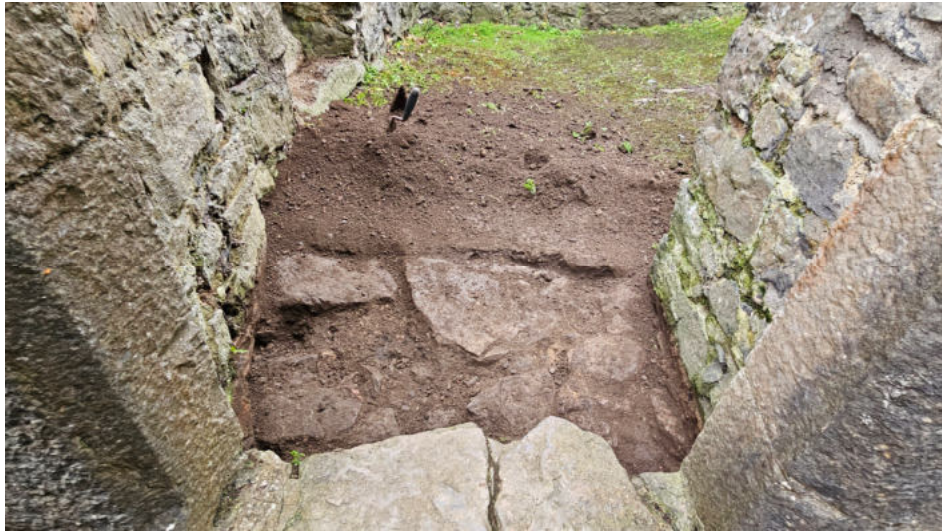
Plate 29: Threshold at first floor level in the residential tower
