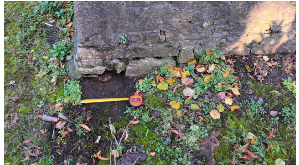
Plate 32: Soil removal from under external buttress at western corner of church
