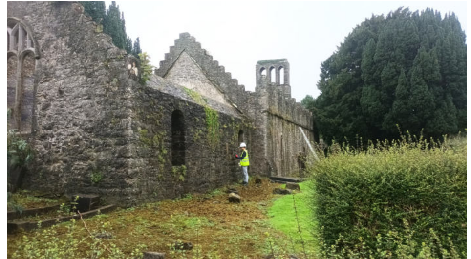
Plate 4: Removal of vegetation from external north wall
