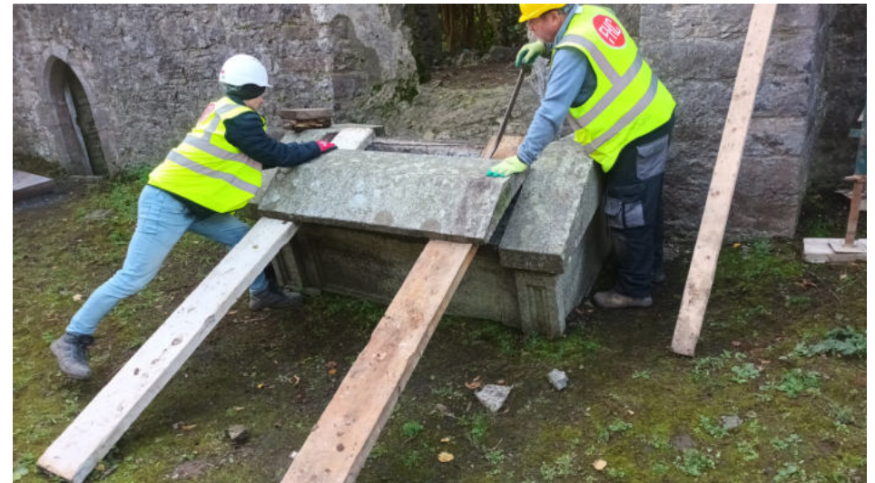
Plate 24: Dismantling of tomb structure from north
