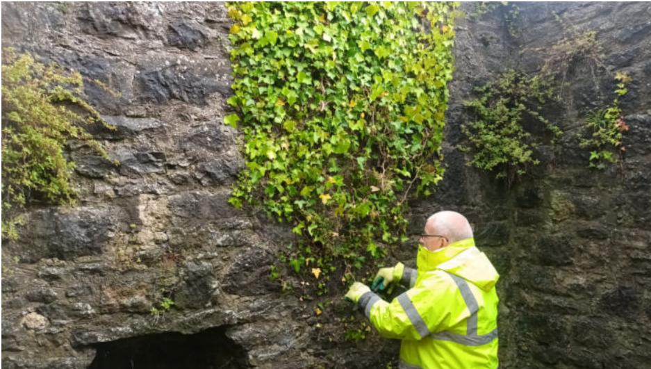
Plate 3: Removal of vegetation from internal first floor of Residential Tower
