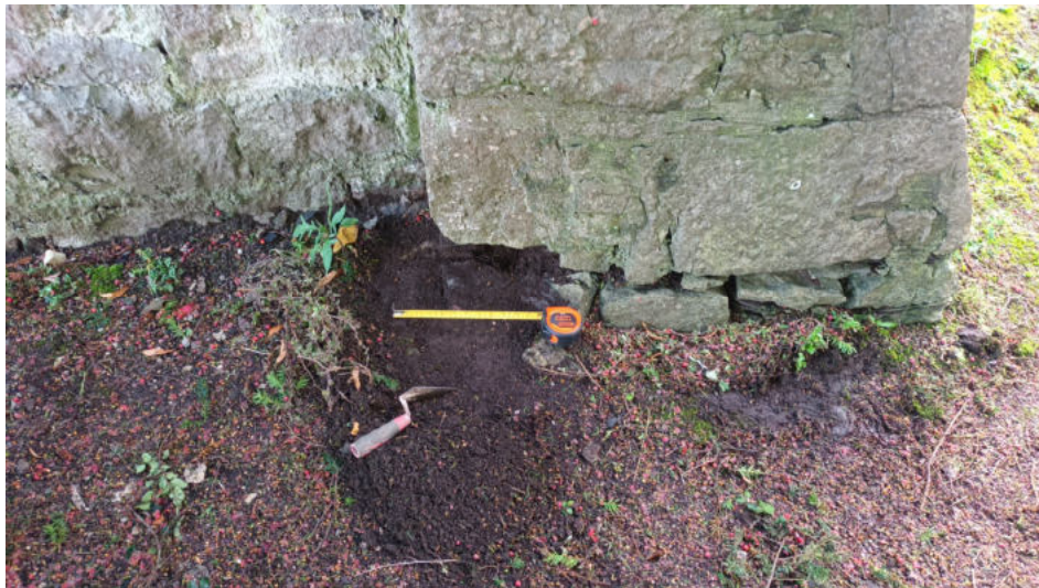
Plate 31: Soil removal from under external buttress at northern corner of church
