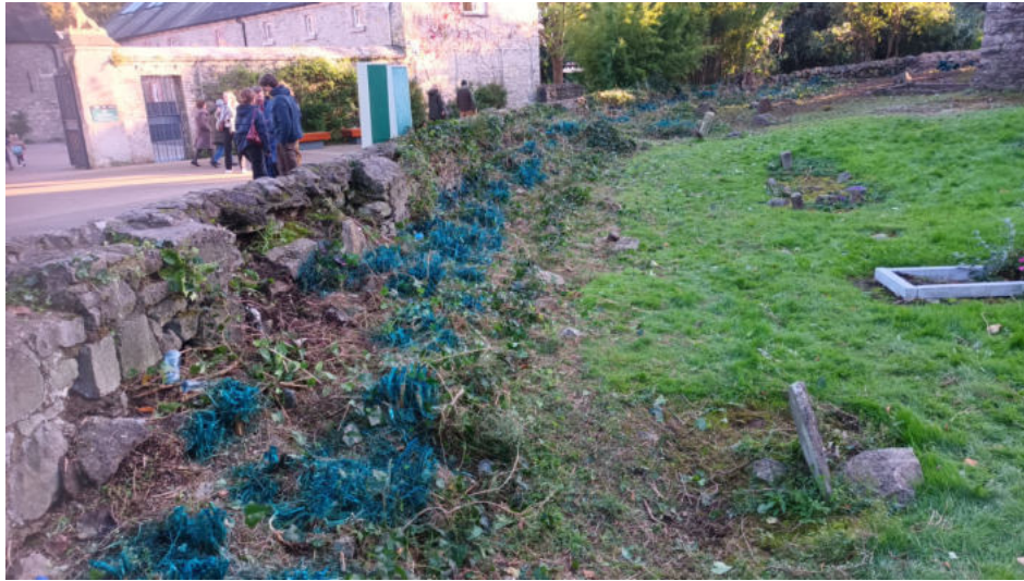
Plate 13: Removal of vegetation from internal side of boundary wall from northeast
