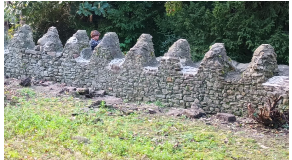
Plate 12: View of repairs to boundary wall from east
