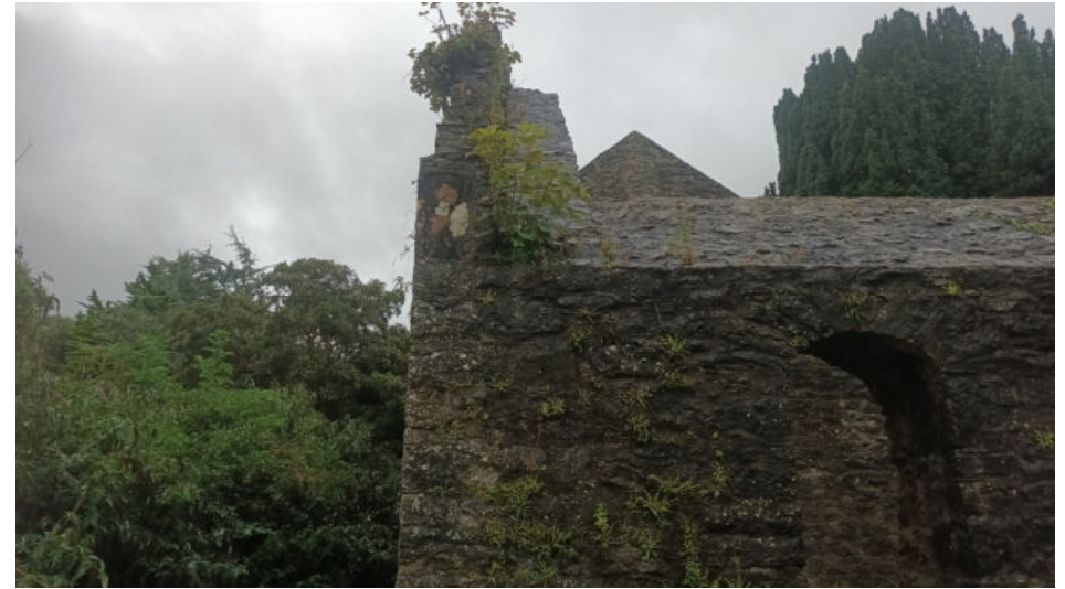
Plate 2: View of NE external wall showing vegetation and Sheela-na-gig DU012-031002
