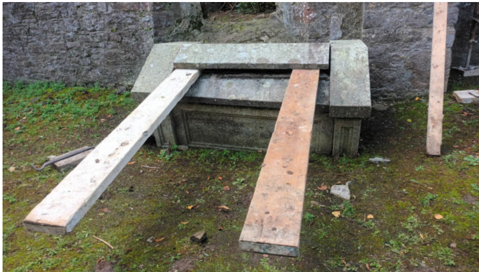
Plate 23: View of tomb in advance of dismantling from north
