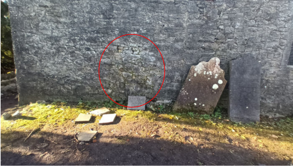
Plate 5: Stone infill observed in east gable following vegetation removal
