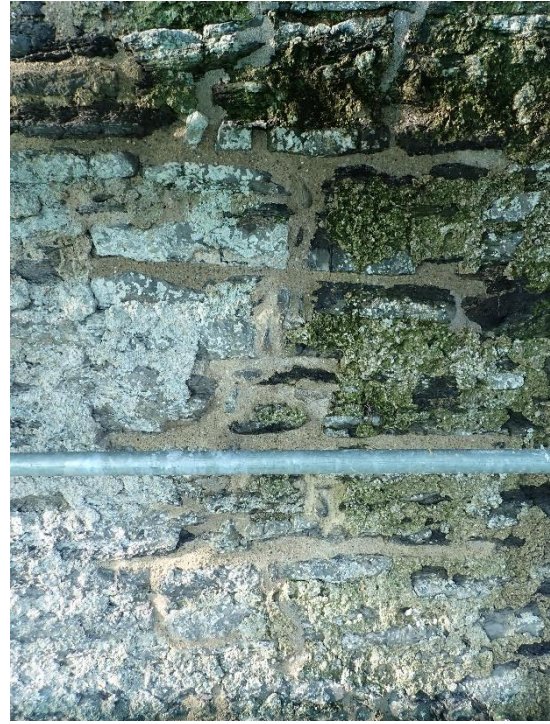
Plates 17 and 18: East face, crack below clock being stitched, filled and then pointed.
