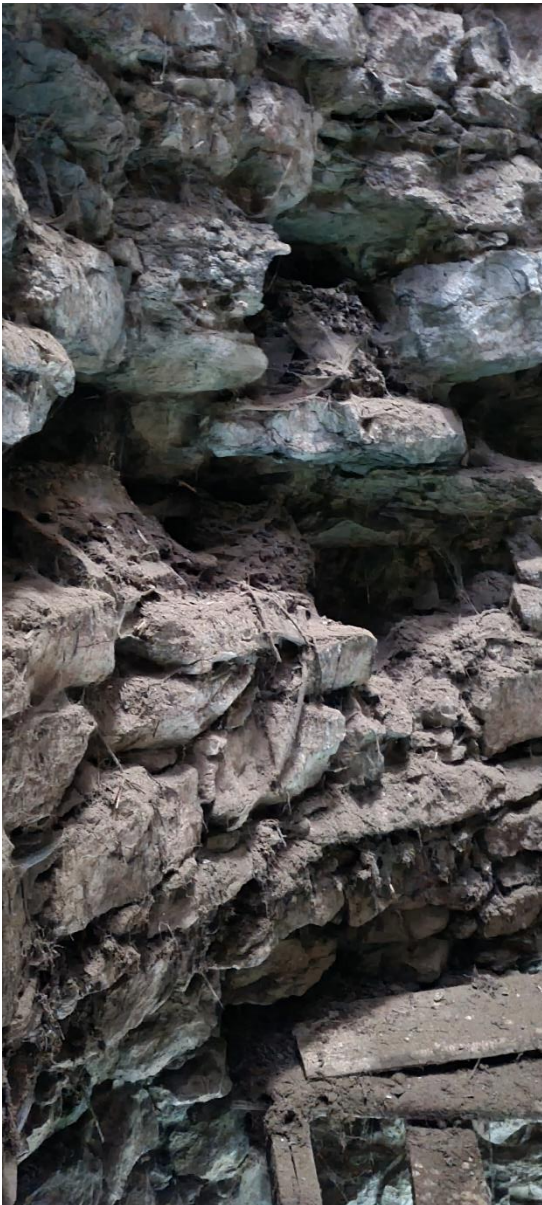
Plate 10: View from the north window looking down. The east window is left below, and the apparent stone loss is from above the corbels of the first floor.
