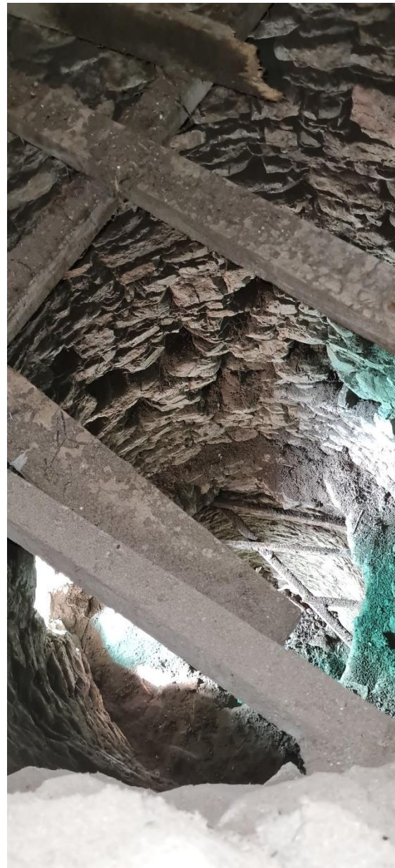
Plate 10: View from the north window looking down. The east window is left below, and the apparent stone loss is from above the corbels of the first floor.
