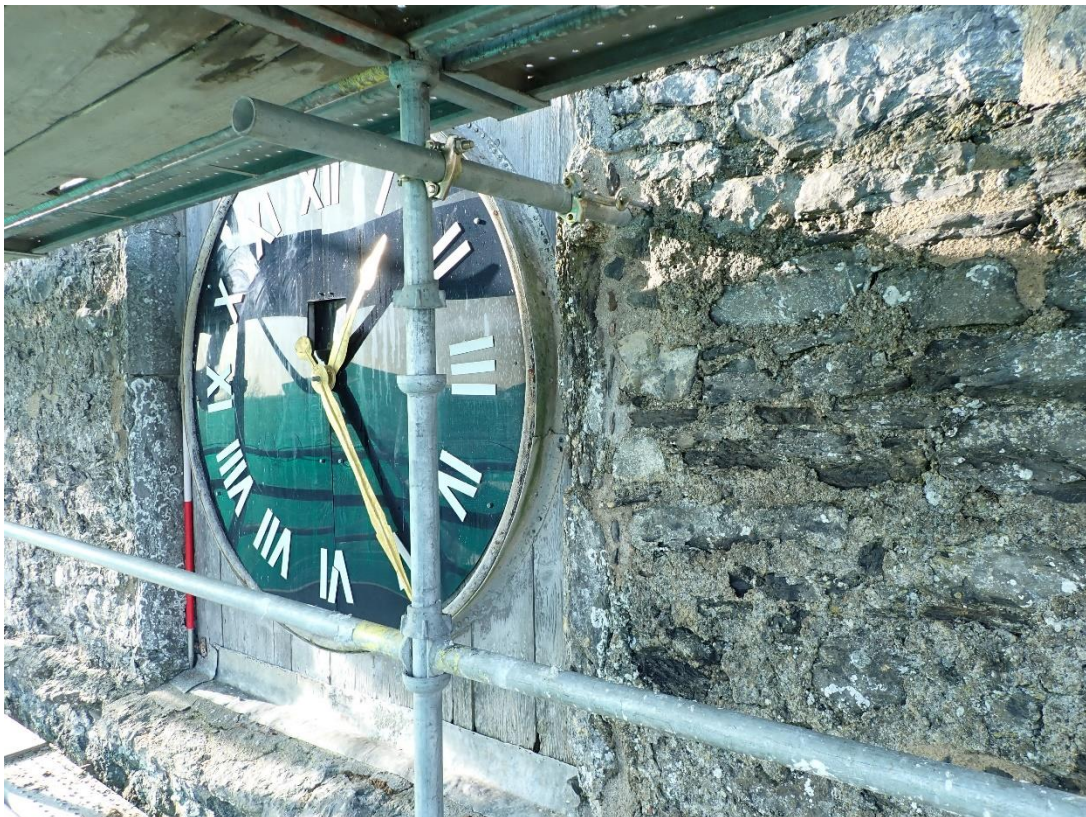
Plate 16: East face, repairs to string course beneath clock
