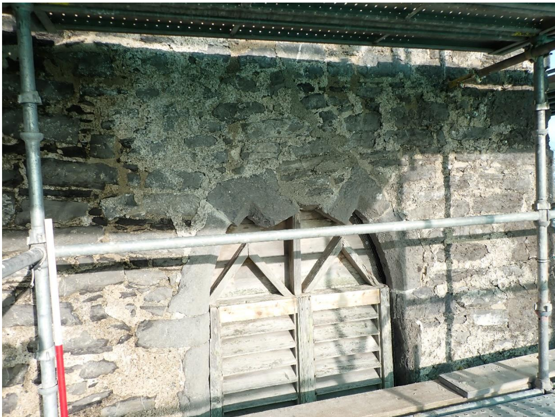
Plate 23: South face, arches above window after stitching with steel bars.
