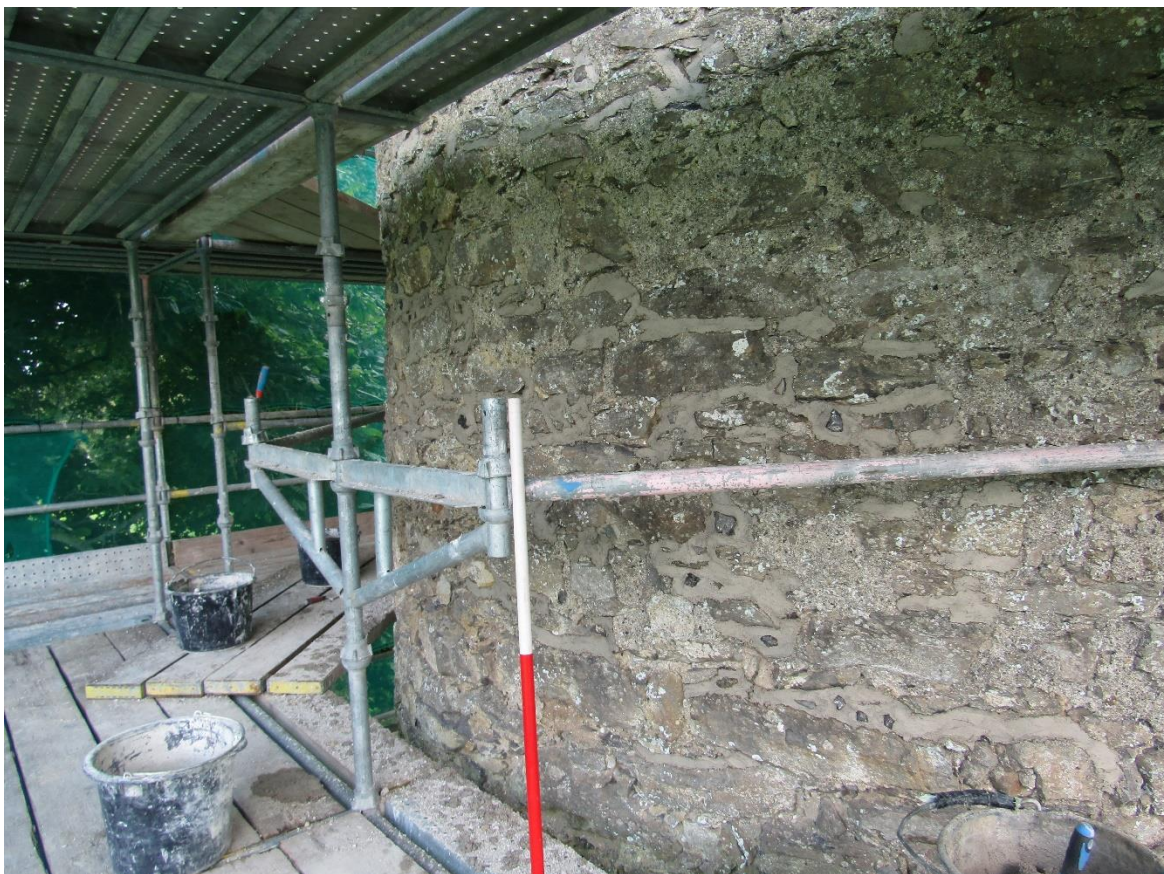
Plate 4: the northwest side next level down with deep gaps being filled.
