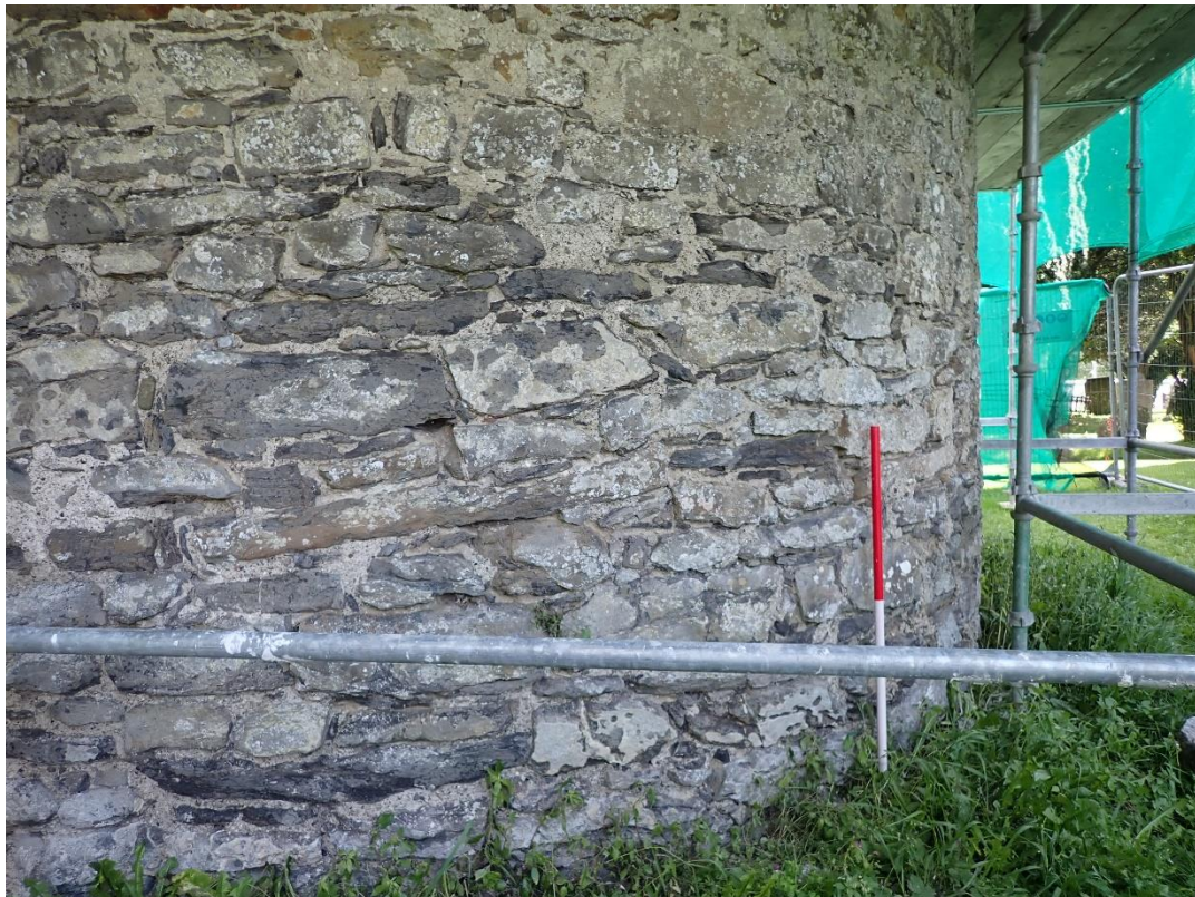
Plate 6: the northwest side at ground level before work was completed.
