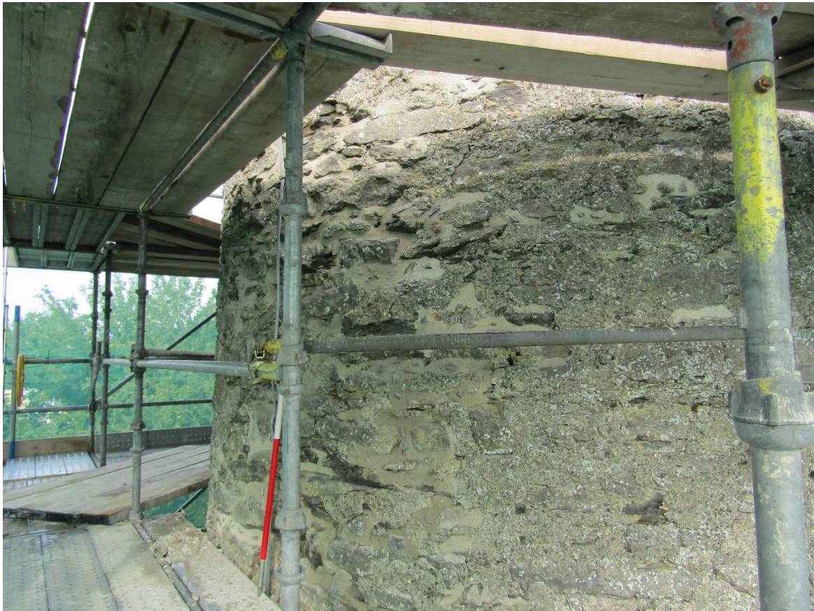
Plate 3: The same section after re-pointing
