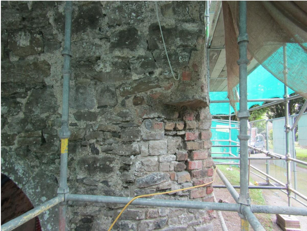
Plate 29: Southeast corner, brick facing on cut out corner, before repair.
