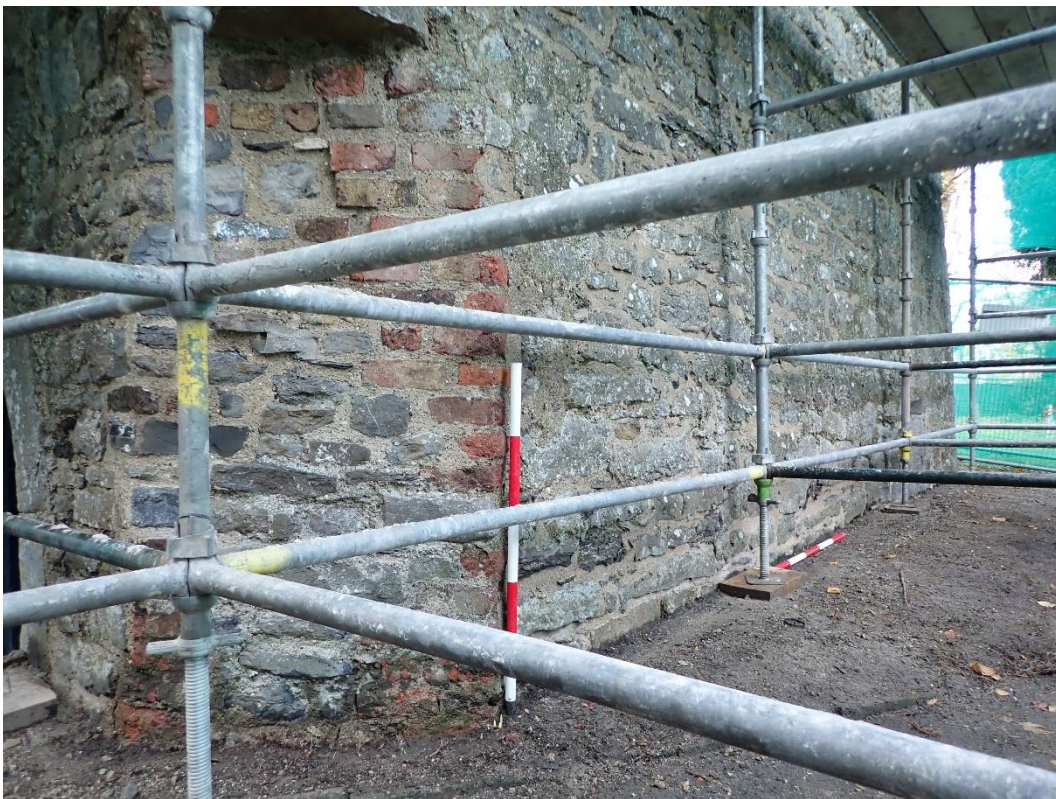
Plate 30: Southeast corner, repairs and re-pointing work completed.
