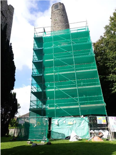
Plate 1: the tower with scaffolding in place
