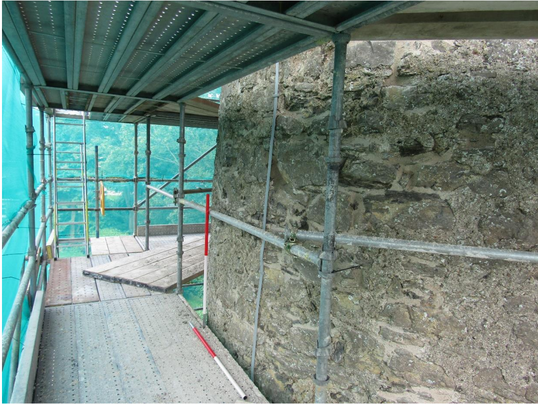
Plate 5: the southwest side after re-pointing
