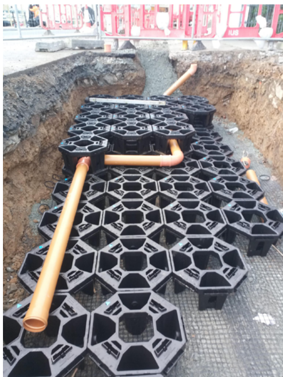
Tree pit under construction
