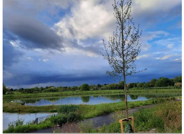
The GSDS has outlined SuDS as a sustainable way to manage surface water as we prepare to meet the challenges of climate change. This example of Millers Glen in Swords, shows an example of surface water being held onsite, providing treatment via appropriate planting, and then discharging at greenfield runoff rate. This is a move away from the traditional method of collecting all surface water via piped systems which can often no longer manage the intense rainfall's being experienced.
