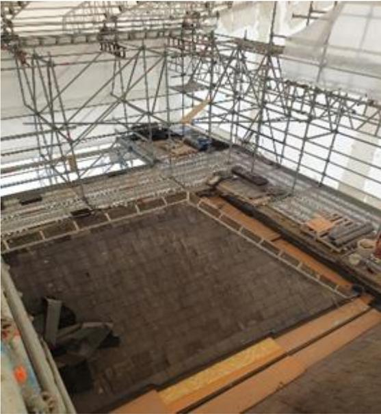
The roof and window conservation works on Newbridge House are progressing well. Insulation of the attic areas have been completed and the fall restraint systems have been installed. Repair works to the window sashes and frames are well underway and are being reinstated in batches as they are completed.
