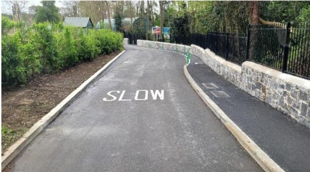
Before and after photos of road widening and new footpath in Shackelton's leading to gardens area Improvement works to widen at the bend in road for vehicles, also a new stone wall and railings on right hand side of road with designated footpath and bollards for pedestrian walkway
