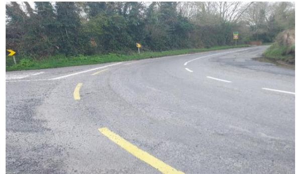
Ballymadun- New lining to improve road safety on the approach of the bend. New warning signage installation in progress.
