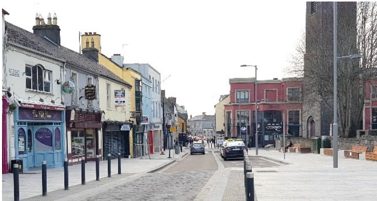
Image 6: Traffic Calming and Increased Footways Along Church Street, Athlone.
