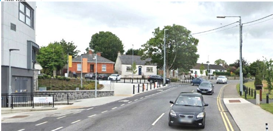
Image 34: Bridge Street / Church Street Junction. Source: NdJ.
