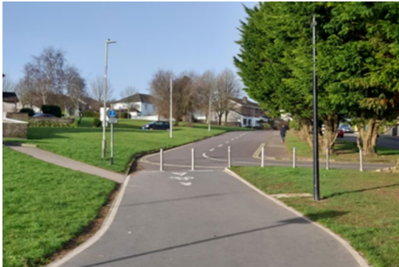
Image 40: Example of Filtered Permeability as Part of Quietway at Ballybrack Valley Pedestrian and Cycle Route, Cork.
