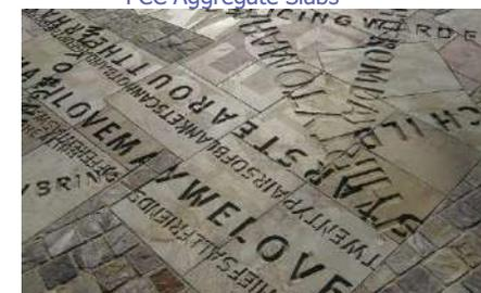
Example of Etched Granite Paving
