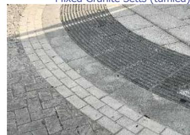
Stone Edges and Tactile Paving
