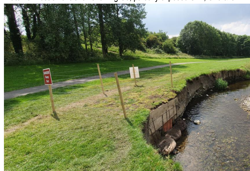
Plate 15: Reinstatement showing safety signs, facing SW
