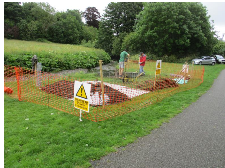
Plate 3: Excavation begins, fencing and safety measures in place, looking NE
