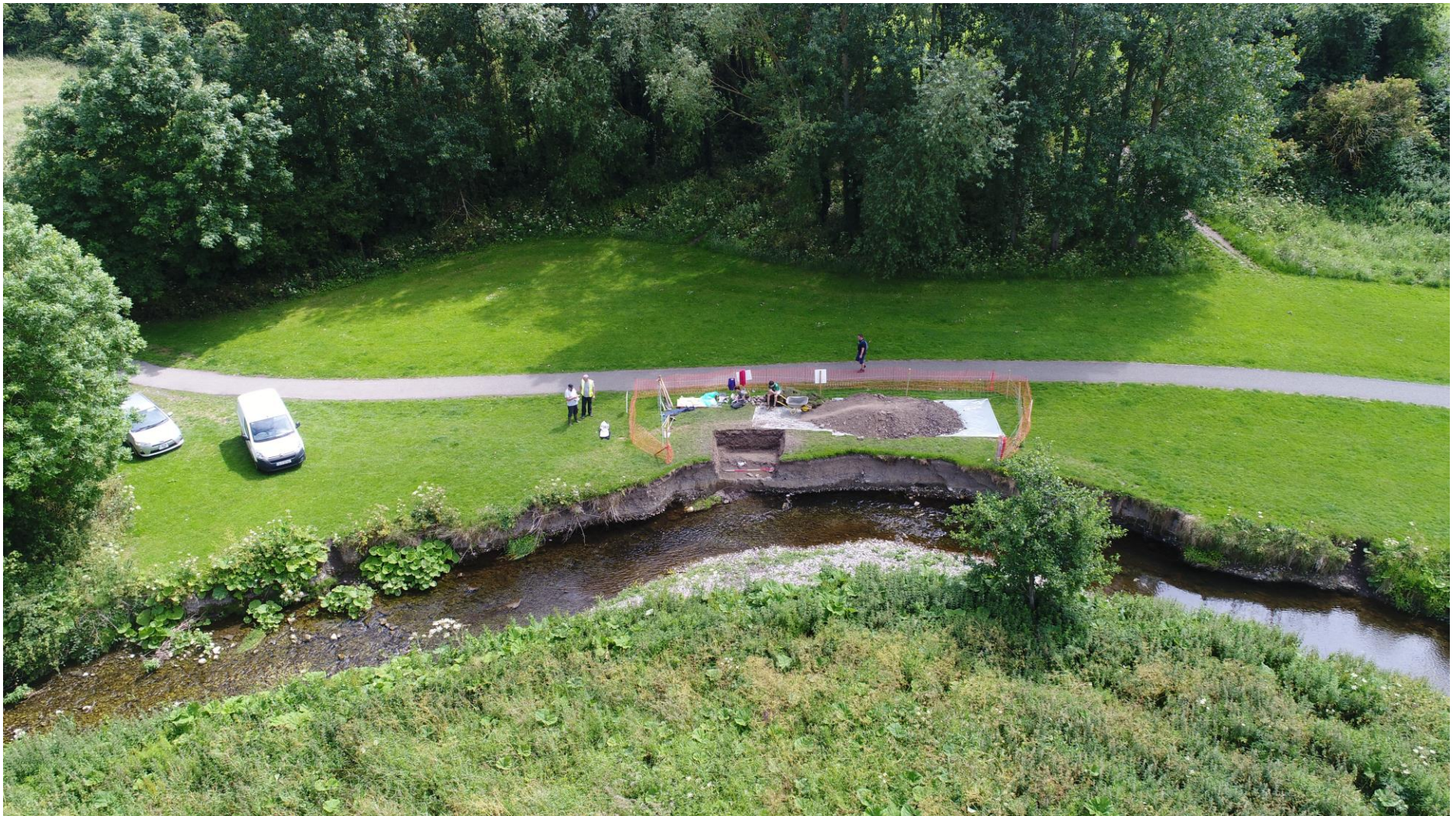
Plate 6: Elevated Pre ex of trench, displaying bend in the river and eroded riverbank, facing south
