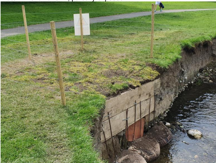
Plate 14: Revetment holding back fill in place, facing SW
