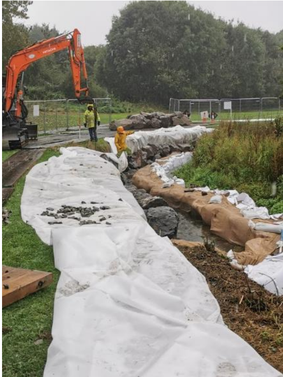
Plate 4: View looking west at the placement of boulders against the bank, protected by geotextile
