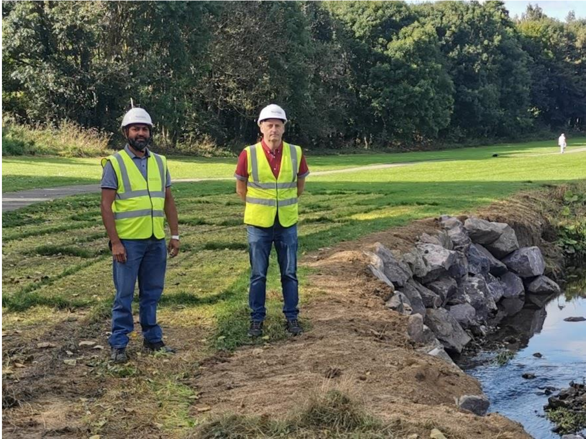
Plate 10: Removal of bog mats after completion of all the reinstatement measures
