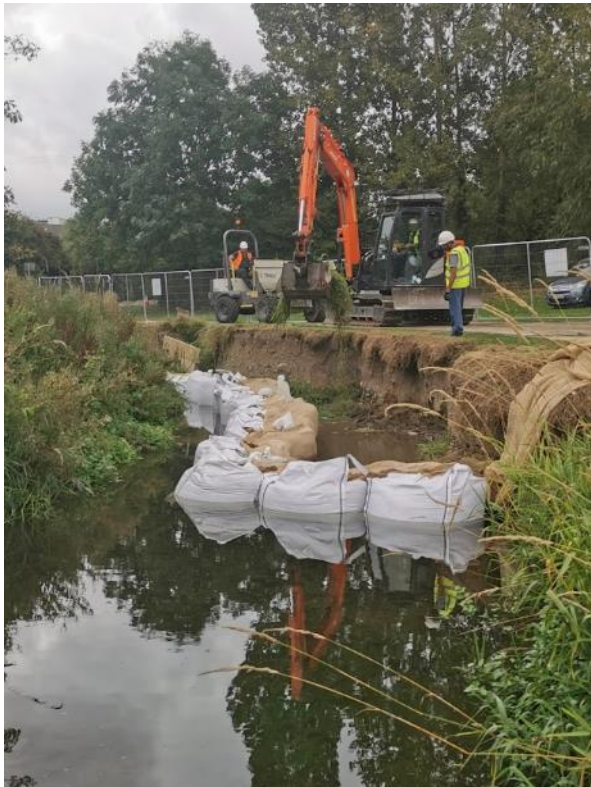
Plate 2: View looking east at sandbags and cleaning of the riverbed
