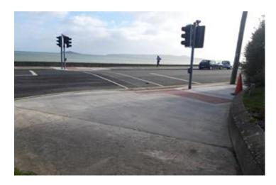
Upgrade of Tactile Pavement and Surrounding Footpath by Wendell Avenue-Coast Road, (Signal heads to be replaced later to ELV type)
