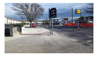
Upgrade of Tactile Pavement and Surrounding Footpath – Grange Road (Signal heads to be replaced later to ELV type)
