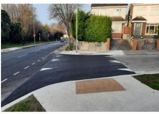
The provision of uncontrolled crossing locations give a safe defined crossing location along the route. These crossing points include tactile paving and drop kerbs which allow a safe crossing location for all road users.
