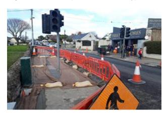
Upgrade of Tactile Pavement and Surrounding Footpath by The Hill - Malahide, (Signal heads to be replaced later to ELV type)
