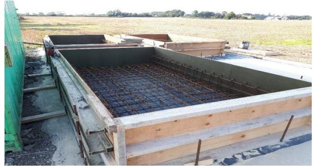
**Installing formwork for beams and deck**
