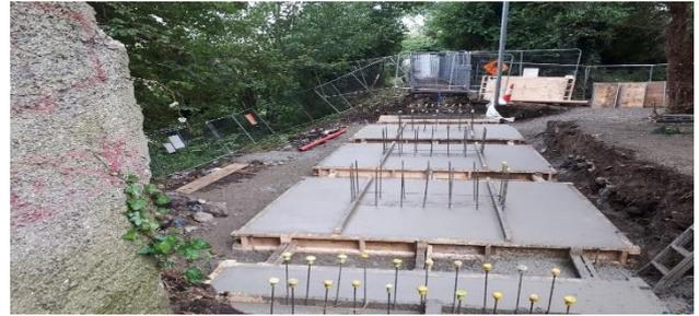
**Prefabricating reinforcement for beams and deck**
