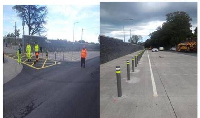
**Installation of Bollards on Carrs Lane has commenced with the purpose of a 3m wide pedestrian walkway along the cemetery wall.**
