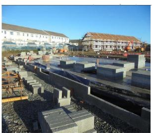
Floor slab & blockwork to units 43-51 (27-35 Kilhedge Drive)
