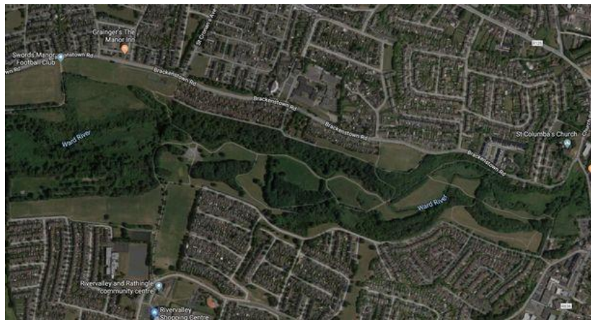
Aerial View of Ward River Valley Park, which acts as a connection hub for all the housing estates surrounding it (Google Maps).
