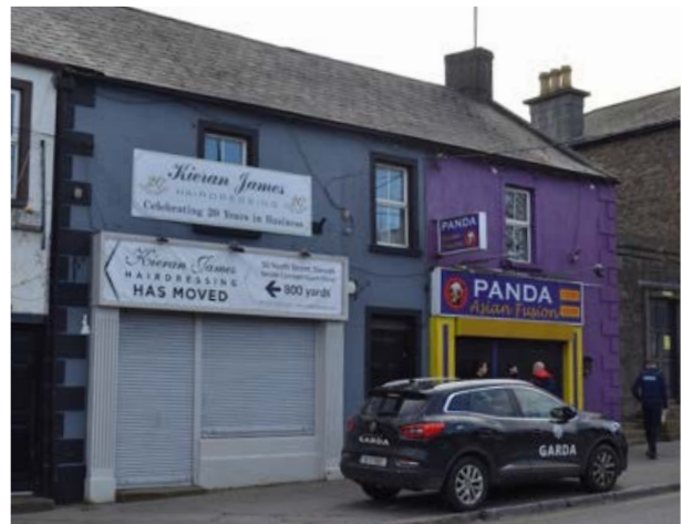
19th century houses with poor signage & shopfronts.
