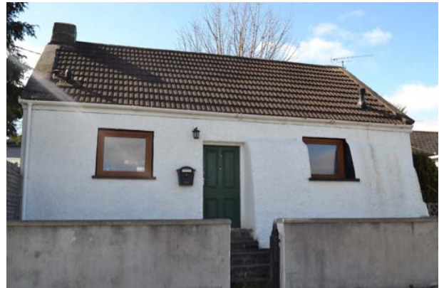
Mudwalled former thatched cottage, probably early 19th century Church Road.
