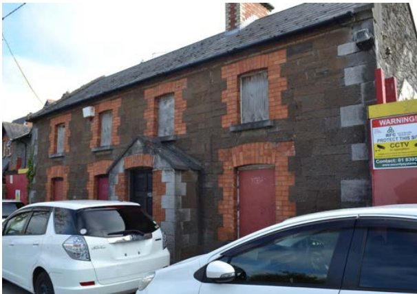
No.40? North Street.
