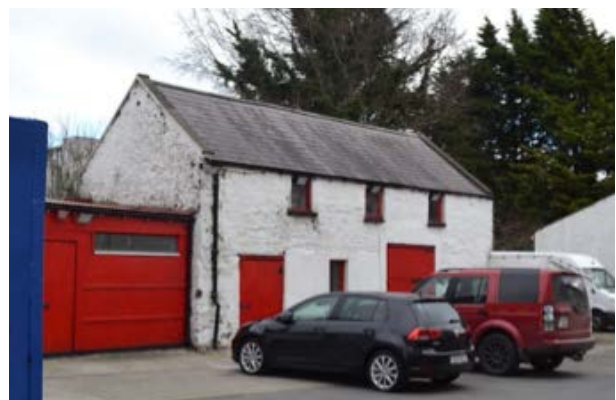
Good quality, possibly co-eval, outbuilding to the rear of No.93 Main Street.
