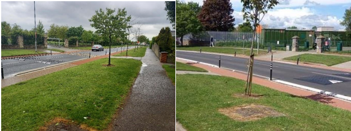
Two Unmarked Crossings on the Rathingle Road (left), and River Valley Road (right). Both these crossings link from nearby schools to parks.
