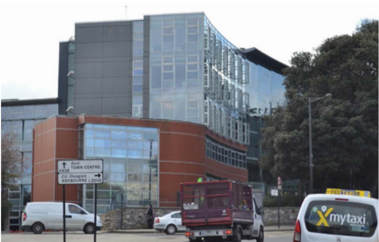
County Hall, Main Street.
