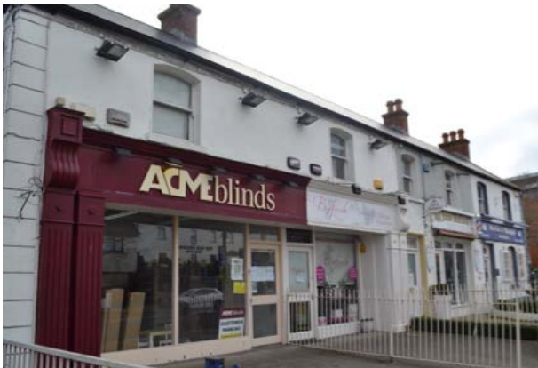
Terrace of houses at 59 Main Street that have been altered with poor quality shopfronts.
