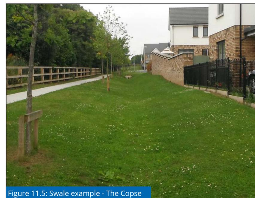
Figure 11.5: Swale example - The Copse
