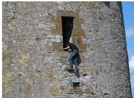
**Figure 30: Martello tower showing door opening and missing brickwork**
