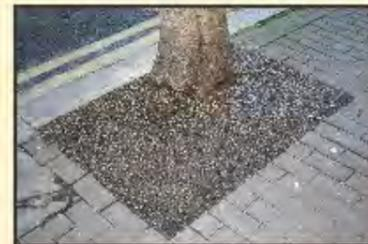
Example of reinstated surface at base of tree using a new flexible material
