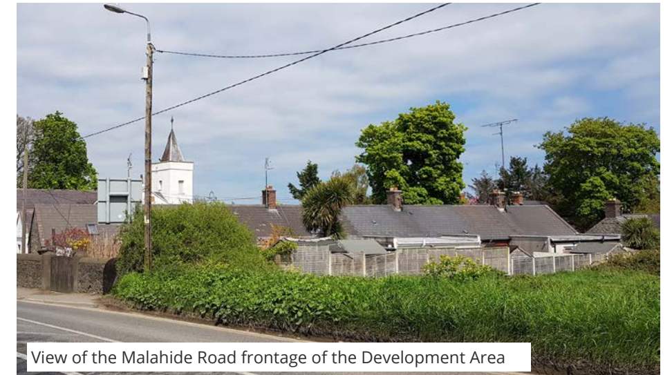
View of the Malahide Road frontage of the Development Area
