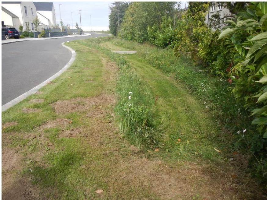
**Figure 6.10** Example Roadside Swale
