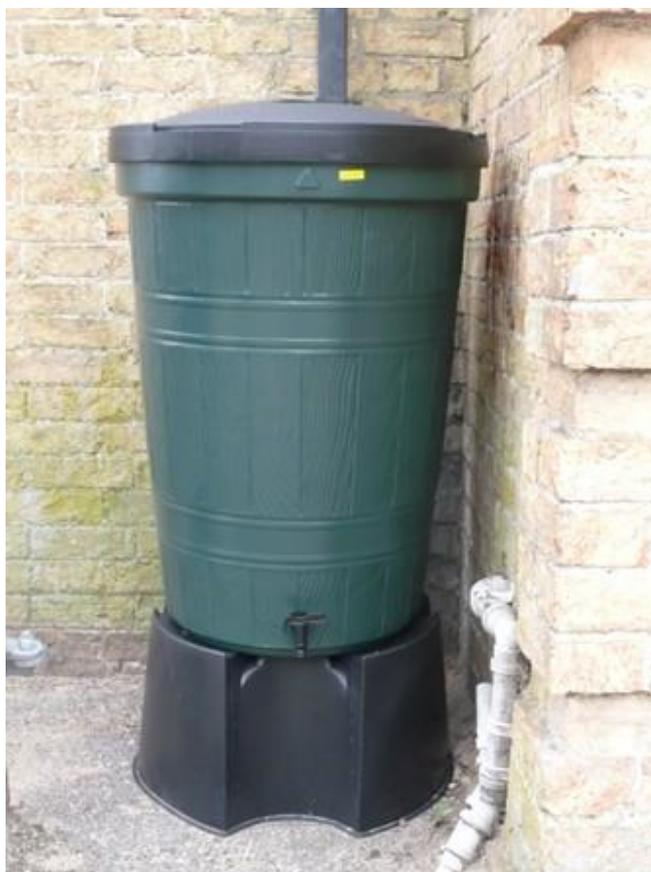
**Figure 6.2 Domestic Water Butt (Susdrain.org)**
